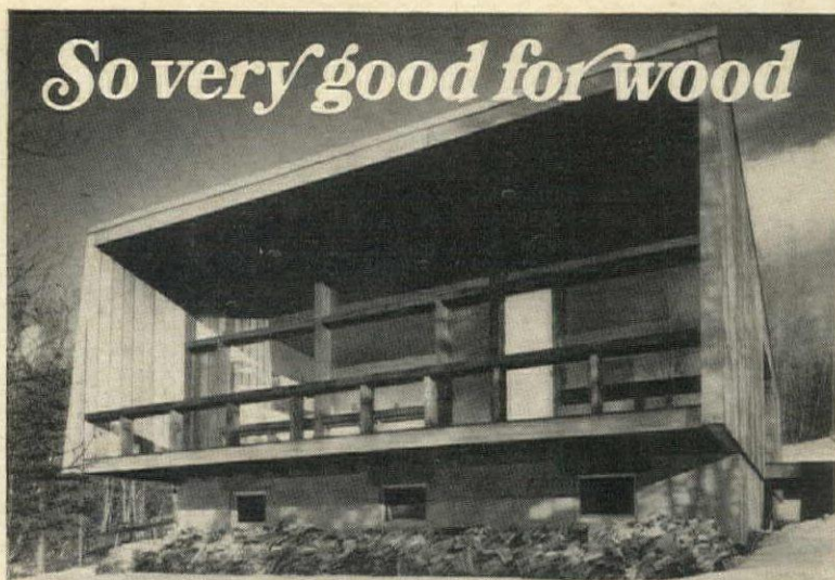
Mountain retreat. Architect: Andrew Daland, Cambridge, Mass.; Cabot's Stains throughout.
