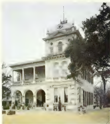
In 1890 the Mathis house gained tower wing
