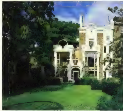
The rear "face" façade of the house
