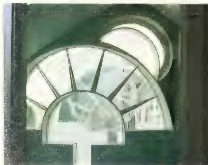
One of two lunette windows looking into the vertical shaft of the Moonwell.
