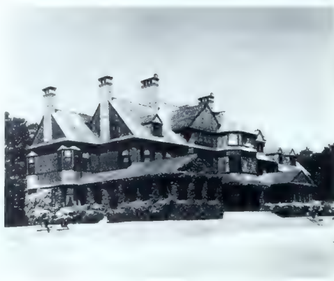
Newport Shingle Style: McKim, Mead & White’s 1883 Southside.
