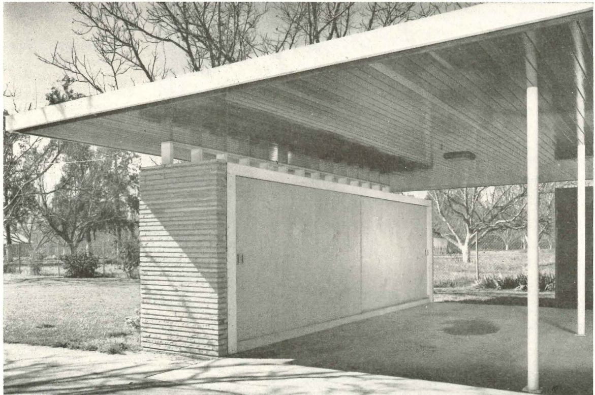
8. Carport storage wall: This storage wall custom-designed by Abe Grossman, Los Angeles, could be adapted by builders anywhere. It is an important design asset, makes the house seem wider; at the same time it provides about 700 cu. ft. of space, behind sliding panels.
