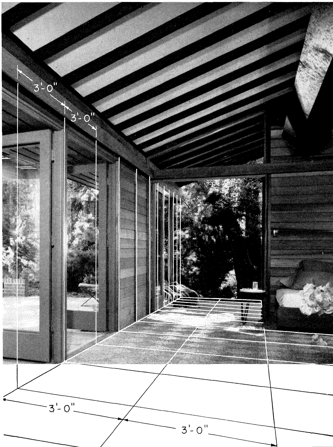
EARLIER PREFAB designed on 4' module was built by Drake in 1947, published in ARCHITECTURAL FORUM that year. Below: typical Harris plan on 3' grid.
