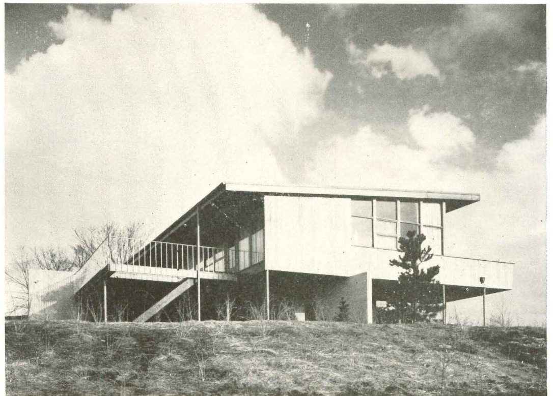
c) Sitting terrace, outside bedroom windows, faces southeast, for morning sun. Jog in plan and extended wall create partial shelter on both sides and above, and covered door to living area (center). The 6' overhang roofs out summer sun, lets winter rays into the living room.
