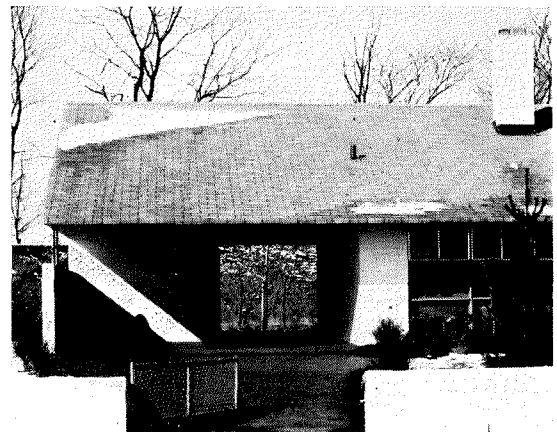
14. Throughway carport: Levitt's new $17,000 house in Pennsylvania (H&H, Feb. '52) has the carport attached at side (or at an angle in front) to make house look wider. It has an 8' x 9' storage room at rear left; area between this and house can double as a porch or rainy day shelter for outdoor furniture. (There is a paved terrace at back, to the right.)
