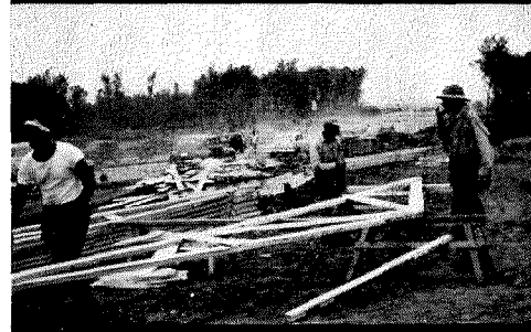
Roof trusses came pre-cut, were assembled at each house.
