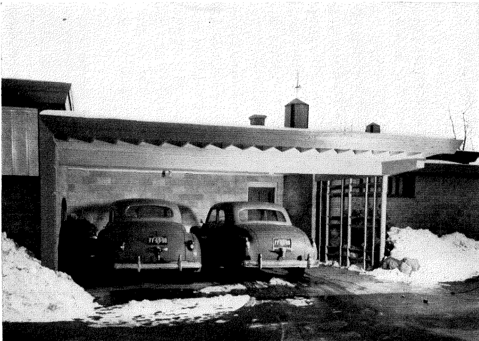
13. Covered entrance-carport: In straightforward treatment (left), architect Kenneth Welch put the carport right at front door of his Michigan house. It is 24' wide, provides a covered entrance. Wood is stored on a low concrete platform at rear, which also serves as bumper for front tires. Turn-around space is big, the driveway economically short.
