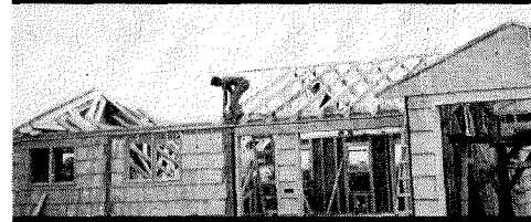
Speed of getting house enclosed was greatest advantage in use of prefabs.
