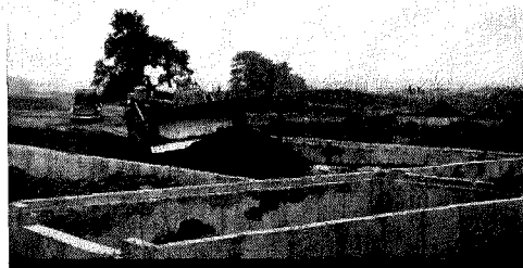
Same slab foundation served prefab and masonry houses.
