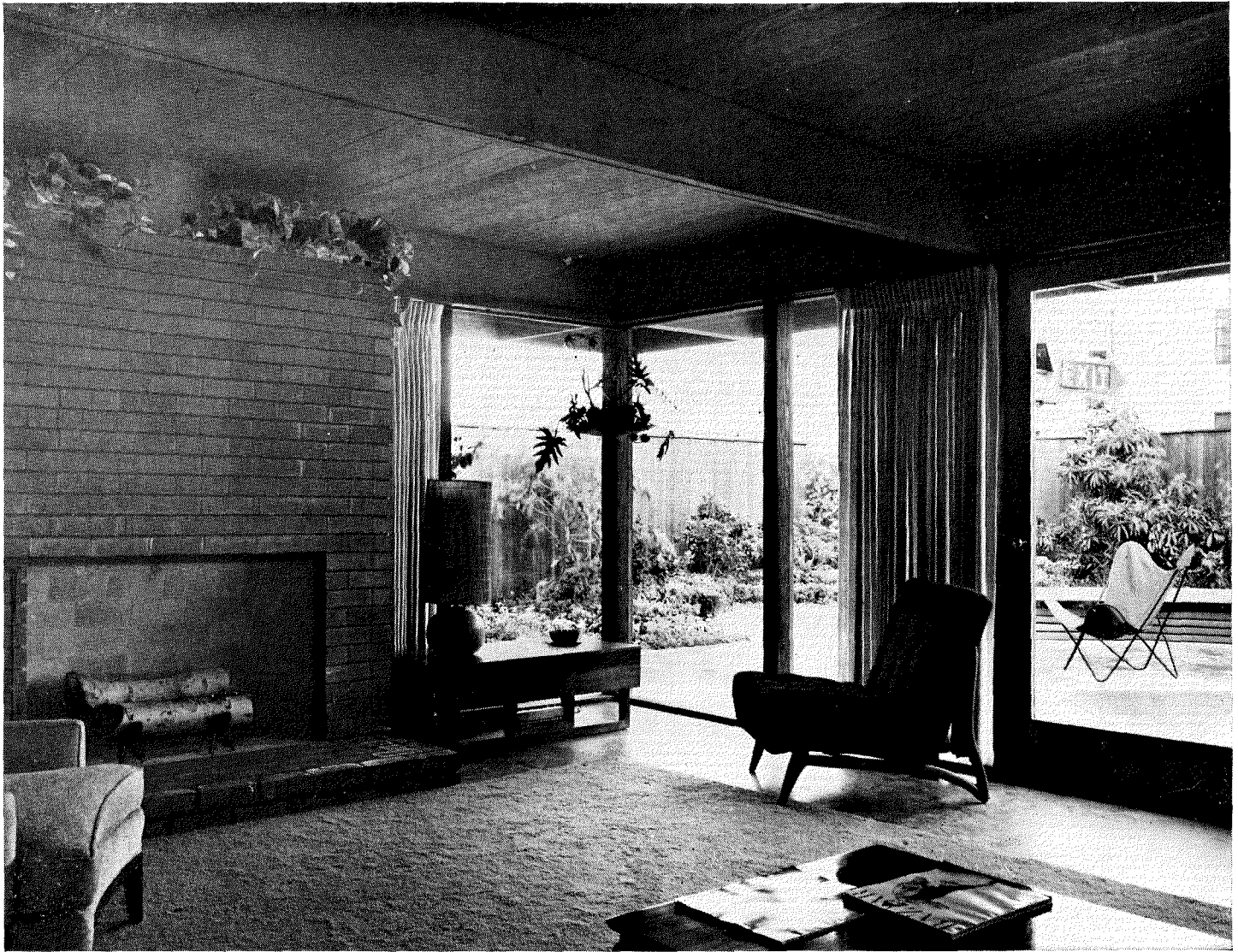
Finished ceiling is underside of 2" x 6" tongue-and-groove roof planking. Brick fireplace was thought to give better color and pattern than concrete blocks originally planned.
