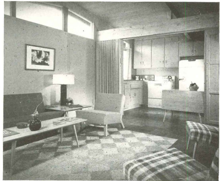
View from living room shows openness of plan, with kitchen and dining a part of the main room. Roof is lifted visually by open ceiling, high windows, open space above partition.
