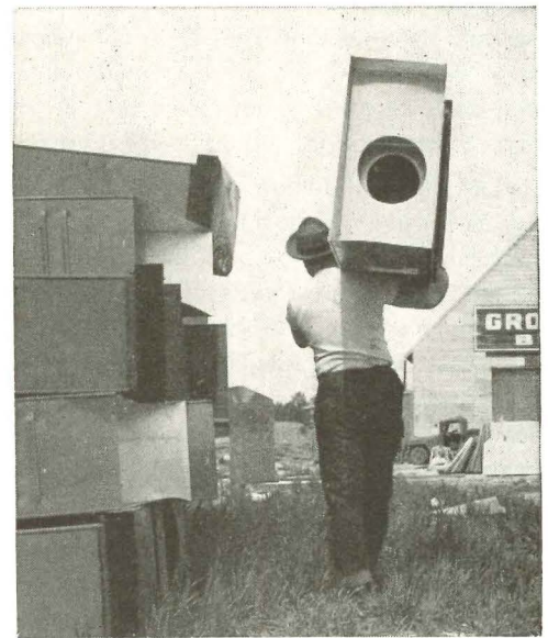
Prefabricated aluminum chimneys are light, easily installed. Favorable weather conditions make outdoor storage feasible, save warehousing expense for stockpiled items.
