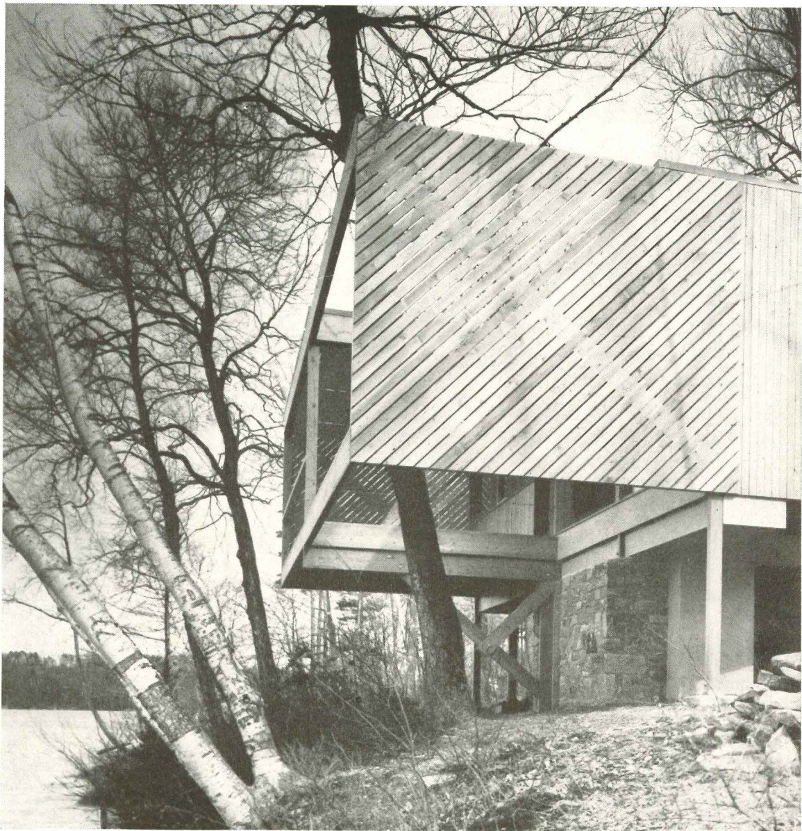
Caesar Cottage, Lakeville, Conn., 1952 (George J. Switzer, Gen. Contractor). The blinders on either side of the view-facade protect living area and balcony from neighboring cottages close by. These blinders are diagonal cypress siding bolted to cantilevered floor and roof girders, form a parallel, cantilevered truss 10' in height.
