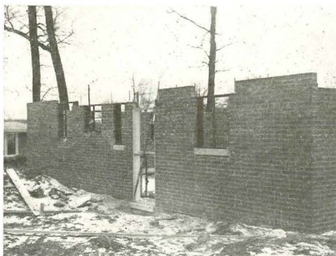
Any moisture which penetrates the masonry will run down the inner face and drain through continuous flashing and weep holes. "SCR" brick and furring need only 8" foundation.
