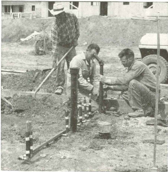
Simple water and waste lines are assembled in factory, hooked up on site. Closet flange spacer (foreground) saves 1½ hrs. of chipping concrete.
