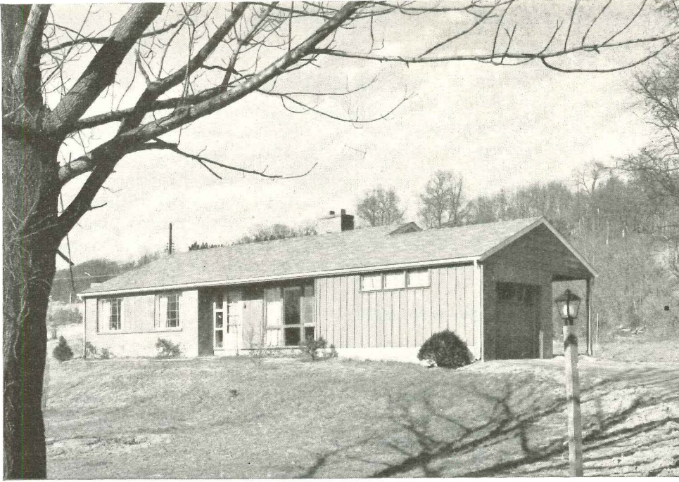
Ground cover, rather than grass, will be used on steep slopes (left) to anchor soil. Fears of erosion were minimized when five-day rain early this spring did only negligible damage to unseeded, raw slopes.
