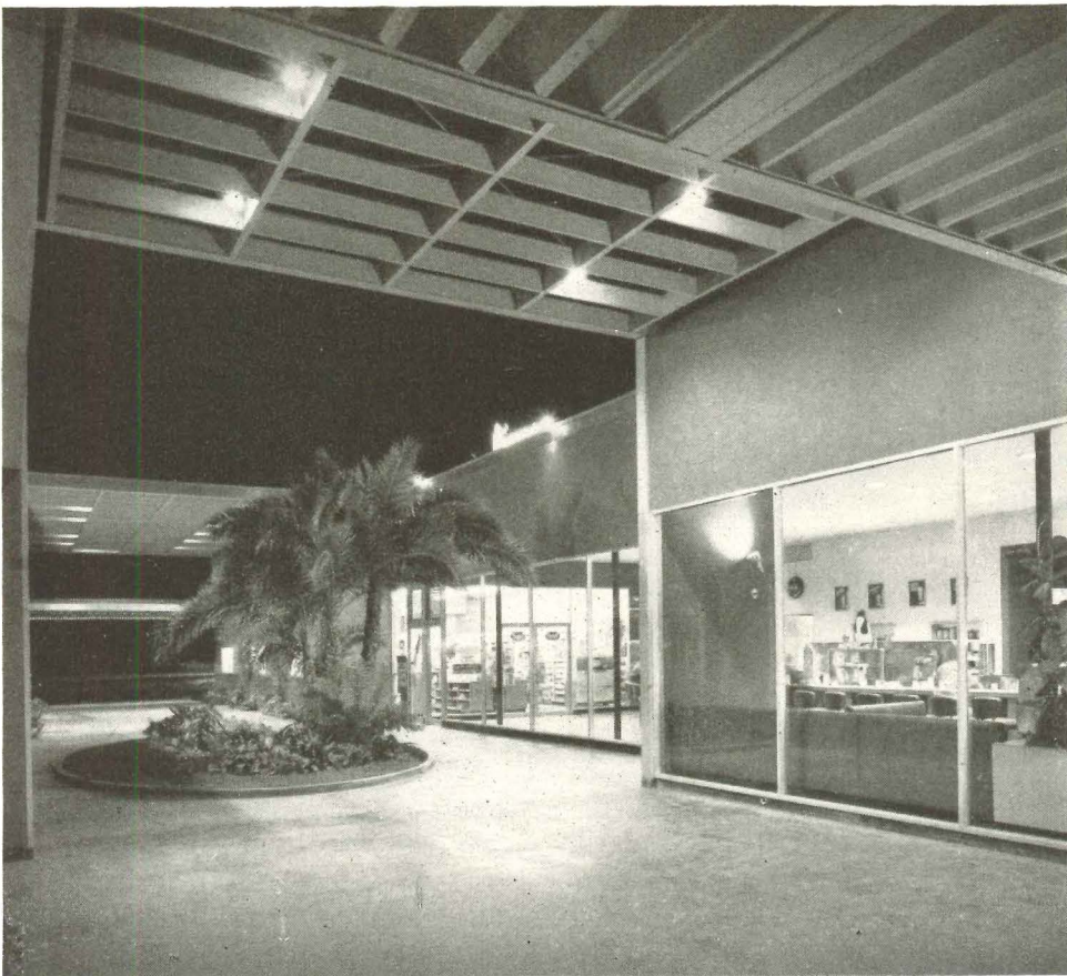
Arcade gives the center additional store fronts, serves as a link between the two parking areas and qualifies legally as a firebreak.
