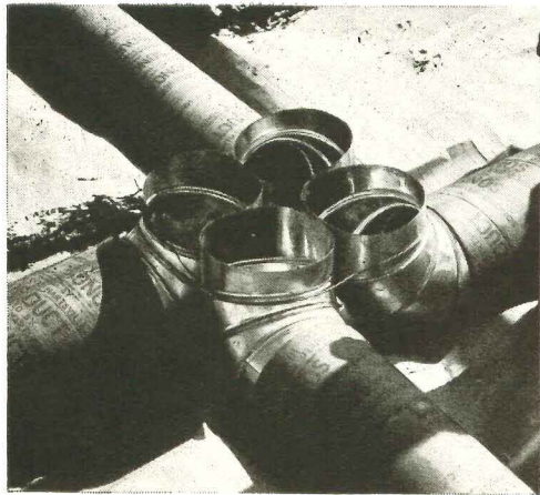
Tod Sloan is convinced assembly, left, is superior to square box plenum under furnace. Elbows act as turning vanes, reduce turbulence. Sheet metal elbows are cheaper than precast concrete plenum.
