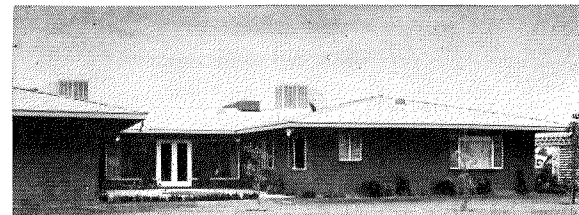
Evaporative cooling units on the roof of a Phoenix house
