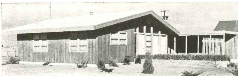
Above is the first of four new air conditioned models Dick Hughes is putting on sale. Right: two doors lead to equipment room. Far right: air cooled condenser installed in the attic.
