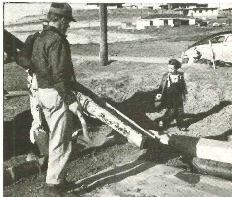
Above: concrete poured around ducts. Photo at right shows spun glass insulation around perimeter foundation and 2 by 4 blocks that raise duct 2" so concrete can be spread below.
