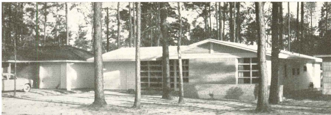
P. S. Luttrell built the house at the left as an experimental model to try out air conditioning, truss roof construction and freestanding storage walls. On the basis of this house, he is set to start building a production line house this fall.
