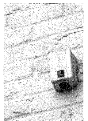
Minneapolis Honeywell's outside "anticipator," below, can forecast inside heating needs.
