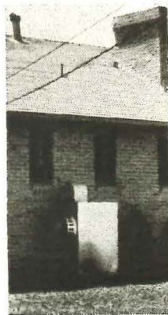
Metal cased forced draft tower.
