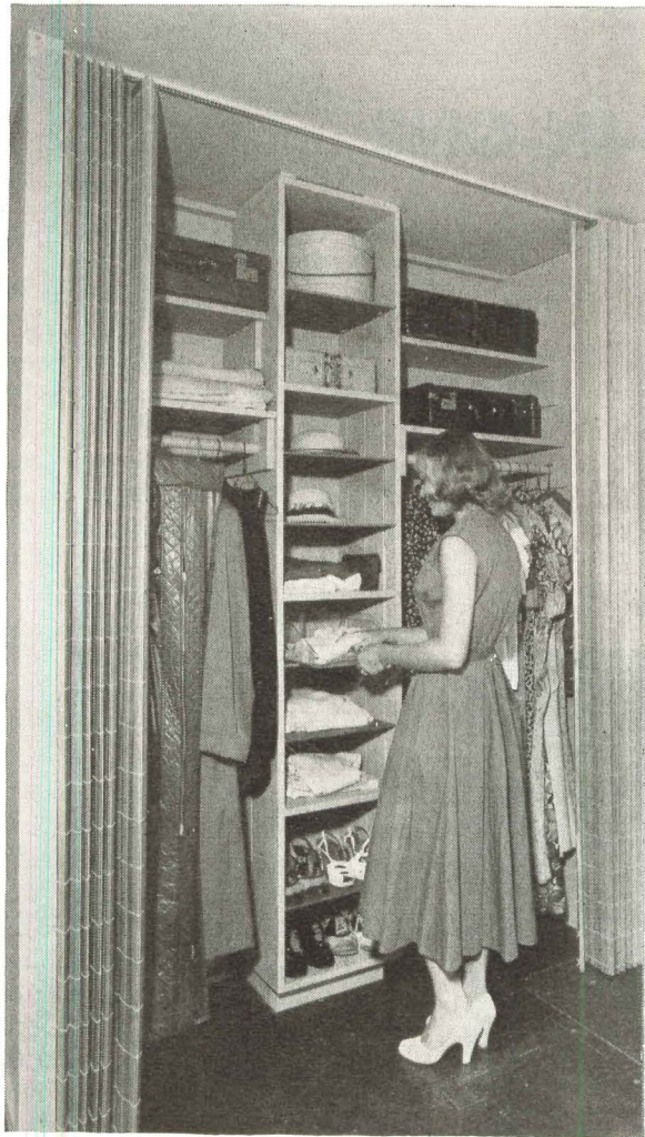
Closet wall developed by SHC under sponsorship of Lumber Dealers' Research Council has multiple shelf unit for stiffening thin wall panels, provides flexible, accessible storage space.
