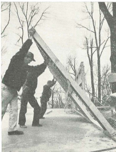
Tilt-up walls are fast, easy to install. They can take roof trusses immediately. A good method in any size operation.
