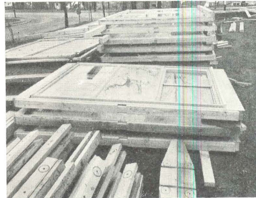
Precutting and preassembly are important factors in reducing building time. In quantity production, an on-site cutting shop would probably be set up.
