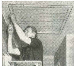
Complete automatic shutter unit fastens with screws to ceiling opening frame; flange forms ceiling trim.
