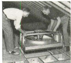
No other attic fan can be installed quicker or cheaper! Fan simply sets over roughly framed opening.
