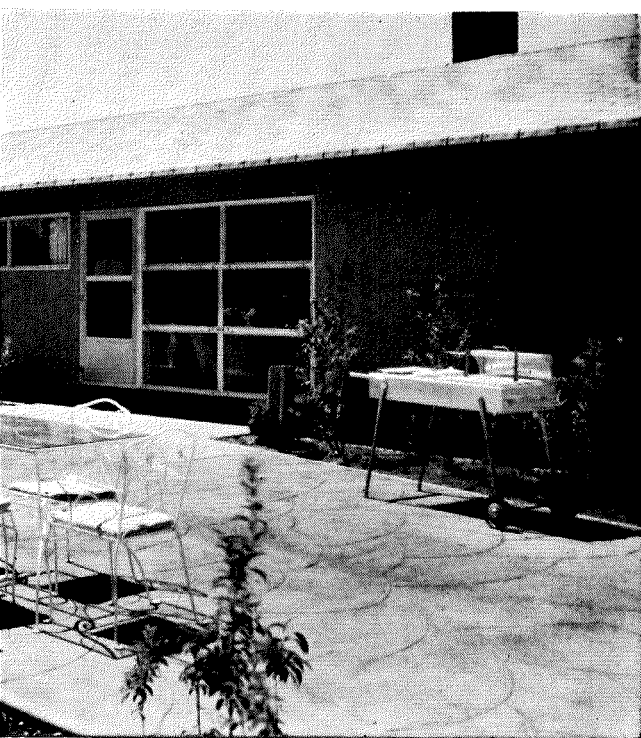
Scored concrete patio, below, simple, inexpensive outdoor furniture like table and chairs, grill on wheels showed visitors to Southwood at Syosset how easily indoor-outdoor living could be achieved. Ideas like this helped sell 315 $10,500 houses in eight weeks. Note big window, door.
