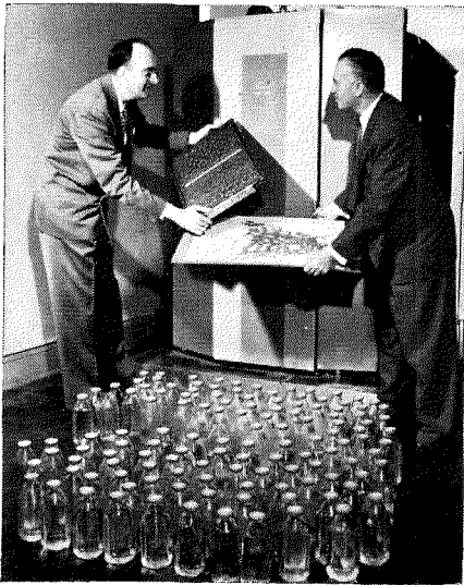
Graphically demonstrating two important by-products of air conditioning is this Servel display: over 100 quarts of water abstracted from the air on damp summer day, amount of dust and dirt screened by filter.
