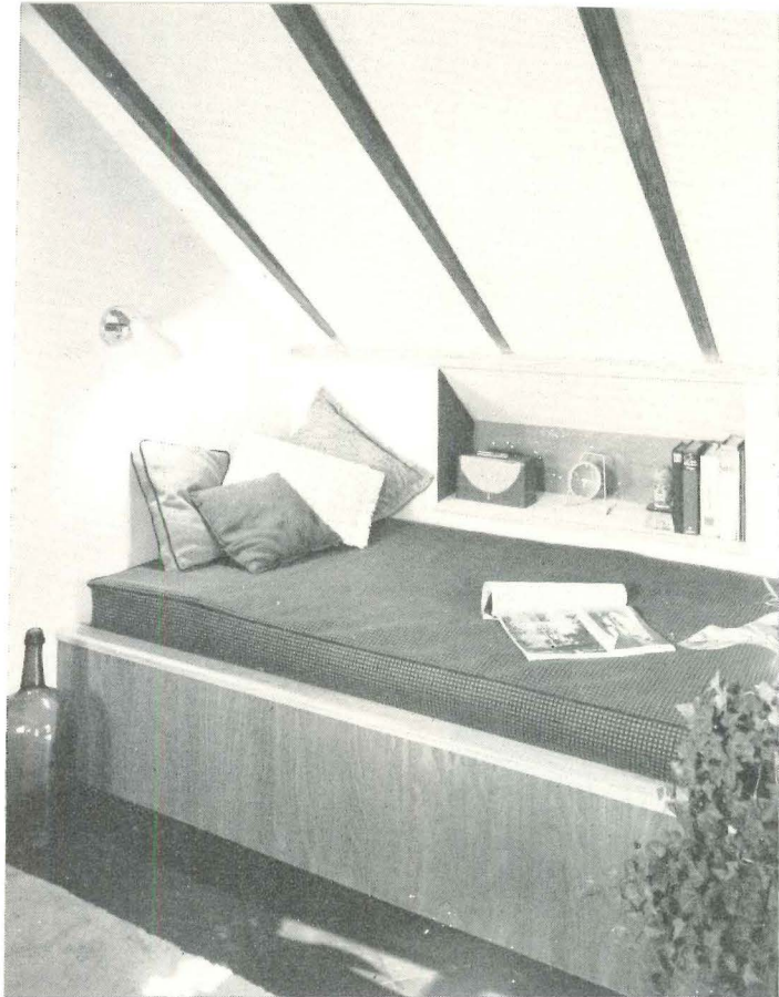
Built for $8 , the bunk is simply two-ply gypsum board over 2' x 3' framing, faced with wood veneer wallpaper. The recessed bookcase follows the slope of the rafters behind.
