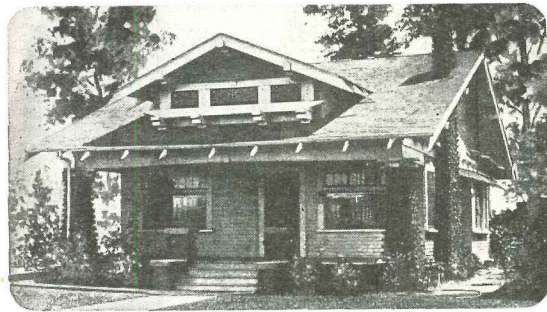
Before: This 35-year-old house needs more than a paint job to make it sell.
