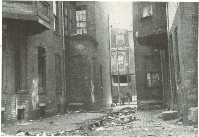
Architect Stonorov's basic problem was to discover which houses, which details such as overhanging bay windows were worth saving. At right, same area from opposite end. One bay window was left, the other was not worth saving. Although houses had similar exterior appearance, each had different interior, called for individual modernization plans.
