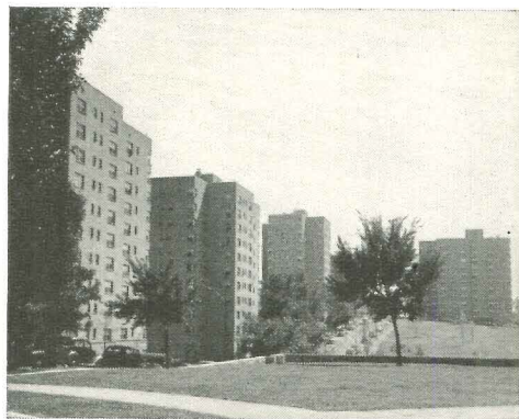
Private redevelopment was done in downtown Kansas City when Lewis Kitchen bought five acres of slum houses, built five 11-story apartments. Rents: $70-$100. Soon he will build seven new office buildings nearby on slum clearance property.
