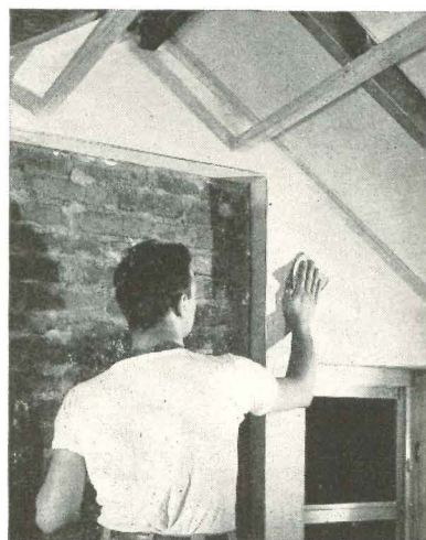
Metal corner bead on tape gives a crisp finish to dry-wall construction.
