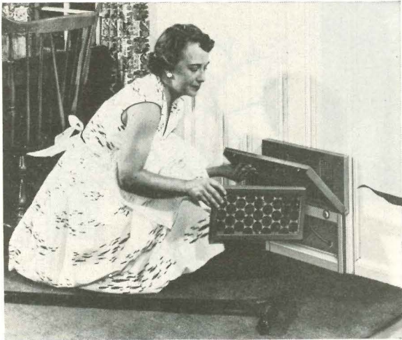
FORCED-WATER AIR CONDITIONING. Baby brother of big-building systems promises balanced heating, cooling for problem houses
