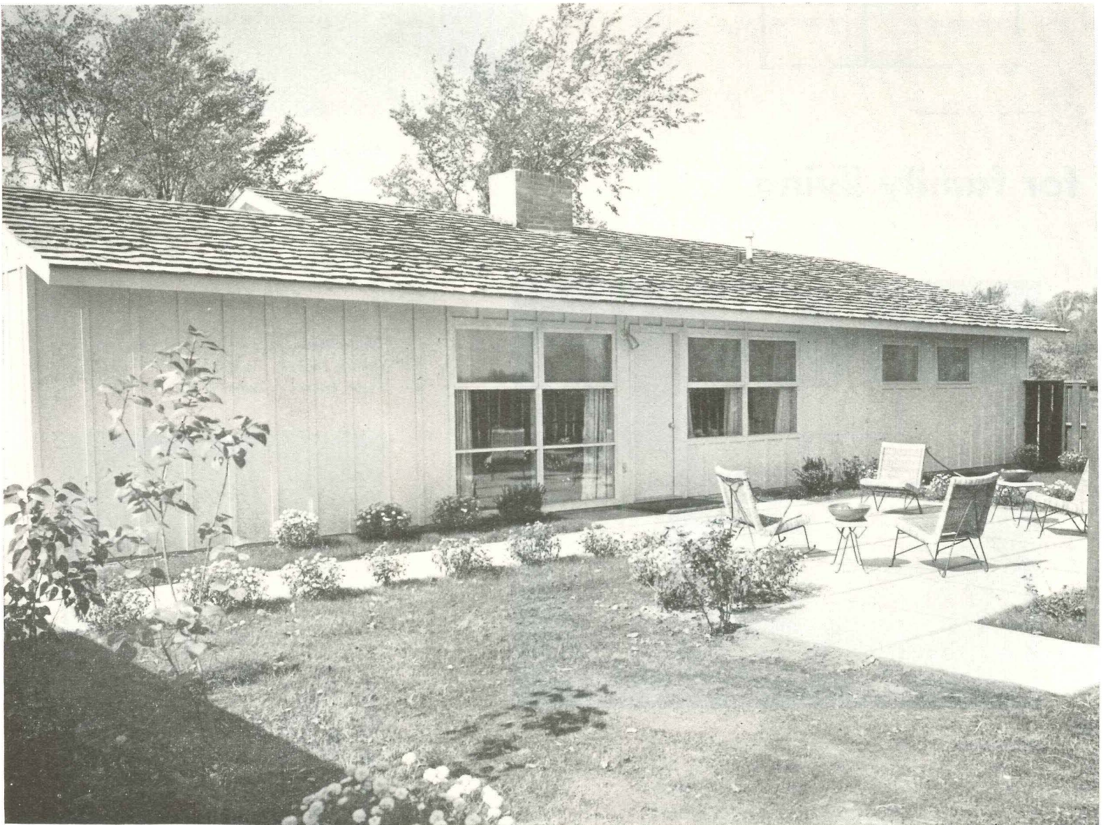
End-to-street model, with private patio at one side, is one of a dozen houses sold before project opened
