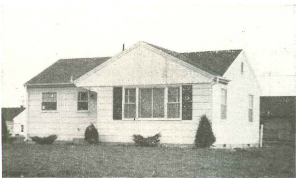
Discarded $8,300 house cost $12 a sq. ft. New house is far better at lower unit cost.
