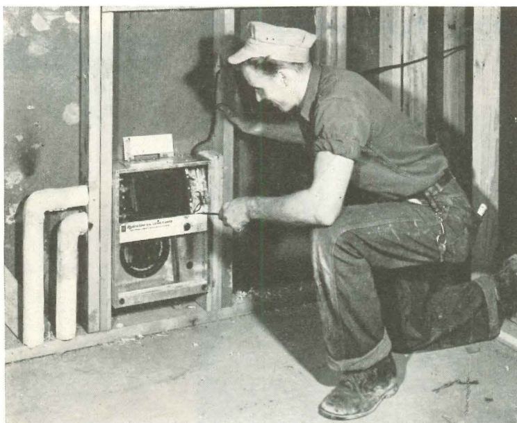
Extremely compact, the individual room units can be set between 16" o.c. studs, or may be installed horizontally between floor joists or ceiling rafters. They also can be adapted to serve both sides of an interior wall.
