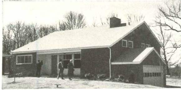
Split at $22,690 (above) outsells ranch (right) priced $19,500, 7 to 1 at "Marble Hills." This is a front-to-back split with three bedrooms running across back of house on upper
