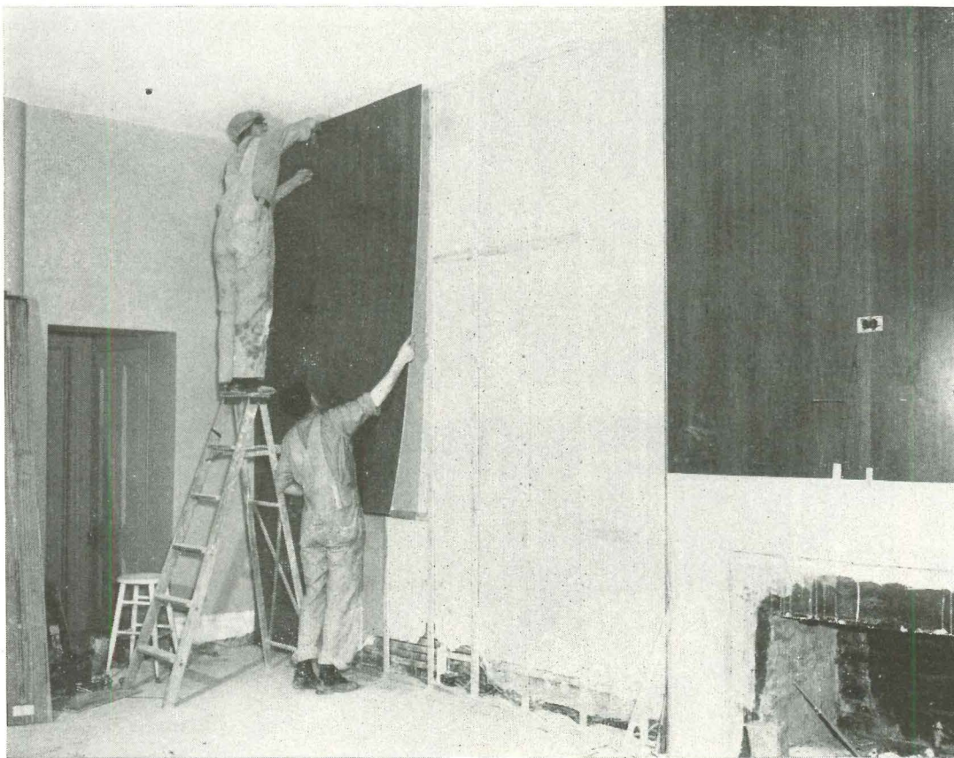
Adhesive is brushed on panel back to fit spacing, then let dry until it is no longer tacky. Studs get same treatment as panel.
