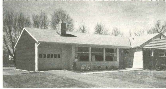
level. Downstairs recreation room, 30' x 14', extends a rear, opens to paved terrace. Ranch house is good but most families will pay more for the larger split.
