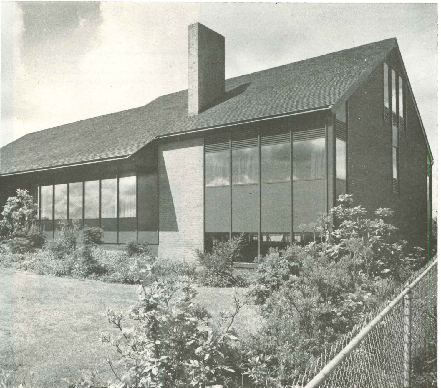
The modular wall panels were painted a gunmetal blue. The brick is rosy red, and the mortar has been colored to match
