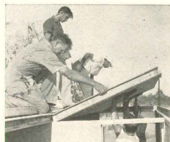
Rigid roof panels weigh 120 lb. each, span 12' with no more than "usual deflection" under load.
