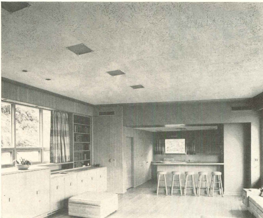
Fissured acoustical tile on ceiling in this kitchen and recreation area of Seattle house designed by George Wellington Stoddard & Associates and built by Nels Hedin is a fiber tile, thus low in cost.
