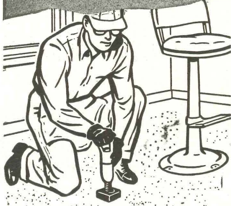
Anchoring seats, bar stools to concrete
