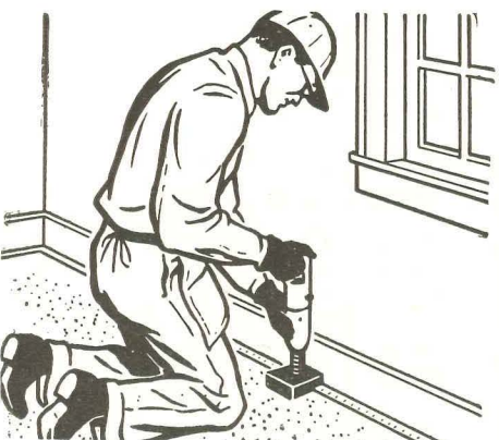
Carpet gripper anchored to concrete
