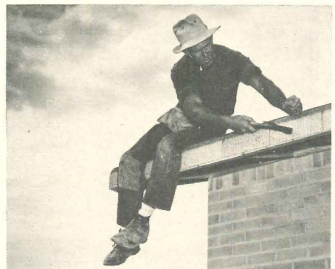
Roll-over shingles eliminate need to paint fascia, have new color pattern which makes them look thicker, with heavier shadow line. Only gutter is a short strip over front door.
