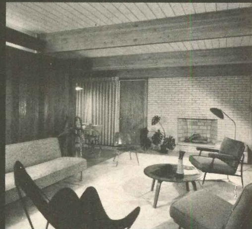
Brick fireplace (above) is treated as wall-element, fits well into modular structure. Heating is warm air perimeter type with floor registers.
