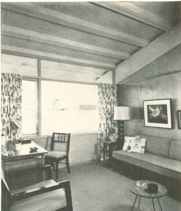
Pan-shaped ceiling plates made of precast concrete which form the roof of Martin Bartling house in Knoxville break up sound waves effectively. Cathedral ceiling also contributes to quiet of house (see p. 114).
