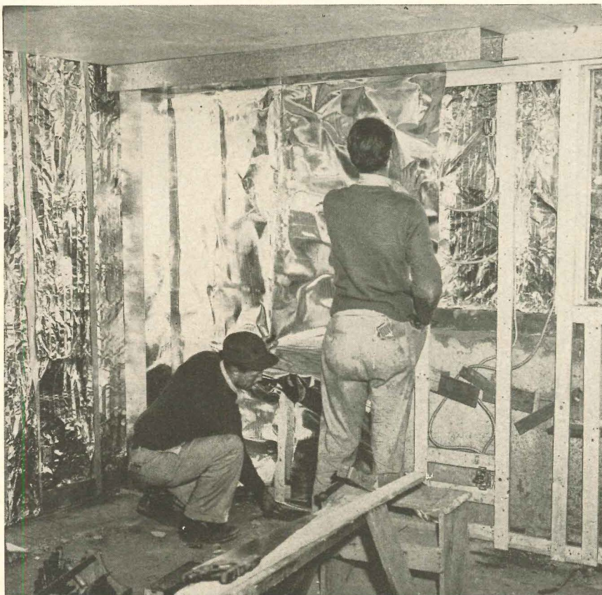
Shiny metal insulation reflects heat, acts as vapor barrier
