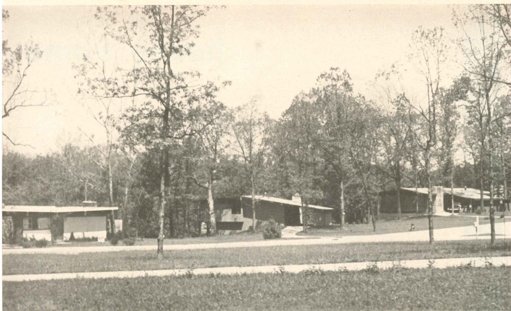
H&H staff photo; architect: Ralph Fournier; builder: Burton Duenke
