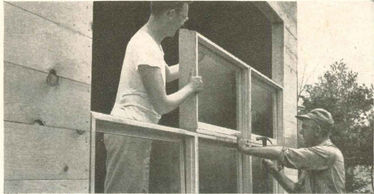
Alternate method for combining Flexivents into large window groups is to build units up right in the window opening. Flexivents come completely packaged ready for immediate assembly and installation.
