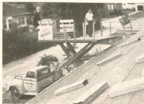
scissors lifts to deliver roofing
