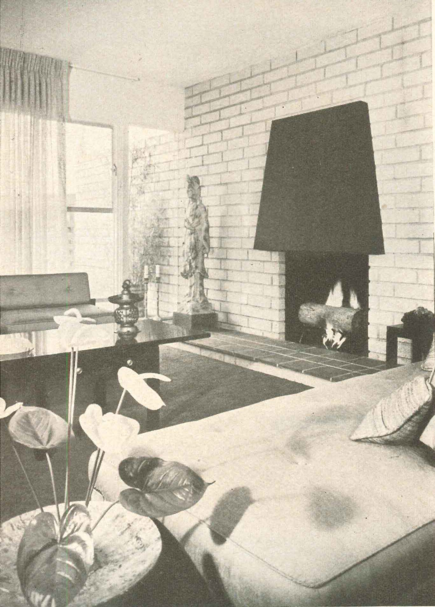
Masonry wall for fireplace with black metal hood dominates the room, adds to expensive look of this $17,600 house. Flush joint between glass and masonry wall is a dramatic feature, is practical for temperate L.A.
