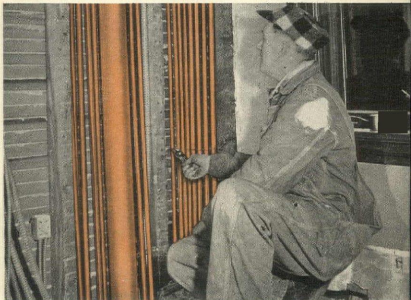
Trim, compact lines. In this remodeling job, two stud spaces served as the chase for the copper tube risers. The large tube is the soil stack; smaller tubes are water supply and heating lines.
