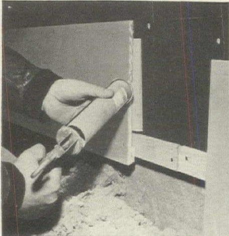
4 Duraply is caulked at each seam to give a tight weatherproof seal. Duraply itself is completely weatherproof—has undergone rigid "tor-ture tests" to prove that it's unaffected by boiling, steaming or freezing—will stand up to most weather.
