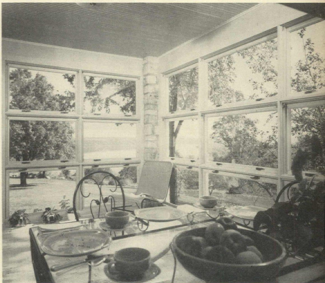
AFTER: Modernized porch was enclosed with unit-windows, turned into all-year-round family room and dining area. Flexible arrangement of ventilating sash makes for better control of breezes. Awning-type units permit use of porch even in rainstorms. Concrete floor slab was finished with composition tile.
