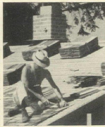
Asphalt shingles are inexpensive, now come with interlocking joints for greater wind-resistance.
