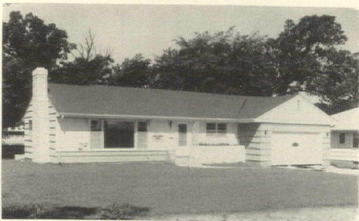
Minneapolis. Builder O. M. Spande saved $25 on this 1,312 sq. ft. house when he cut heating-cooling bills from $214 to $171 a year.
