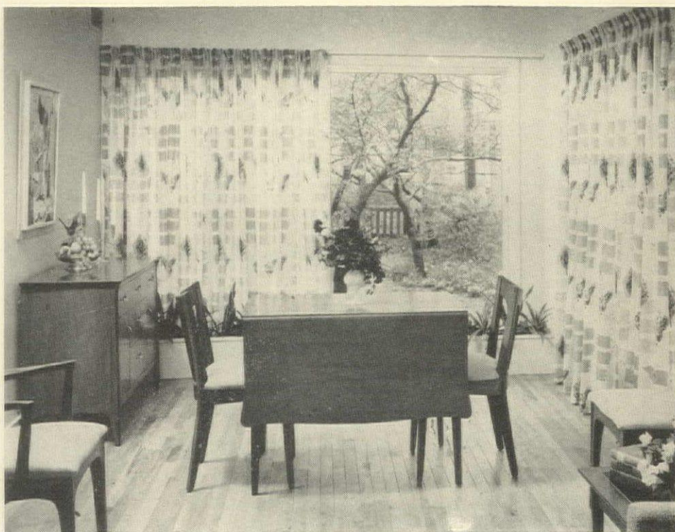
AFTER: Rear wall was opened up with sliding glass doors, turning the view to the private rear yard. Planting box is removed, according to season, for access to the rear terrace.
