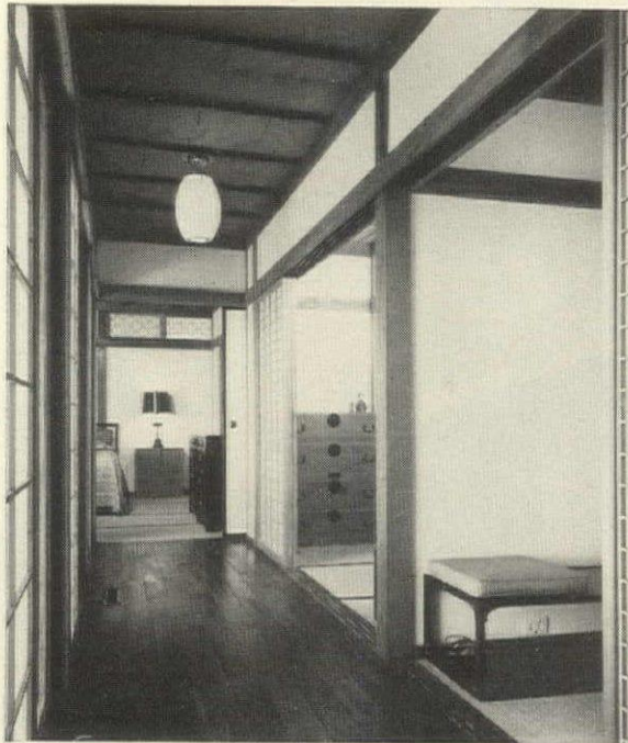
Detail (right) at entrance to living area shows post with one side unplanned. This is traditional "post of honor." Fretwork grille above doorway appears throughout house above the 6' high continuous lintel.
