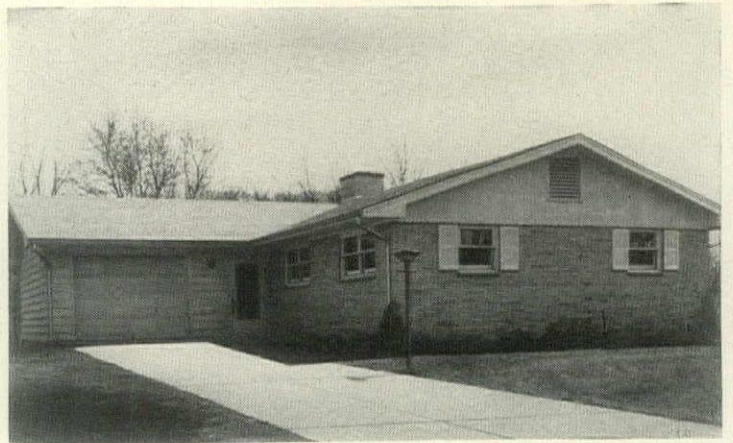
Chicago. By spending $98 more on this 1,315 sq. ft. house, Shiffler & Sons cut heating-cooling $47 a year in an area of high utility rates.
