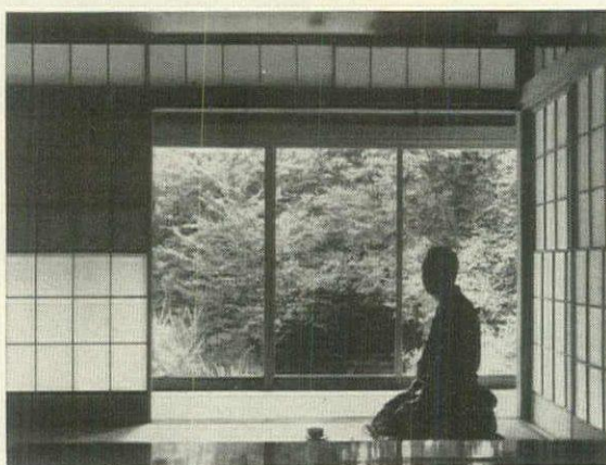
Owner sits on floor mats, his eye level about 2½' above floor. This height governs much of traditional Japanese design. Shoji screens slide horizontally, but each screen is also divided into halves that slide up and down just like our double-hung windows.
