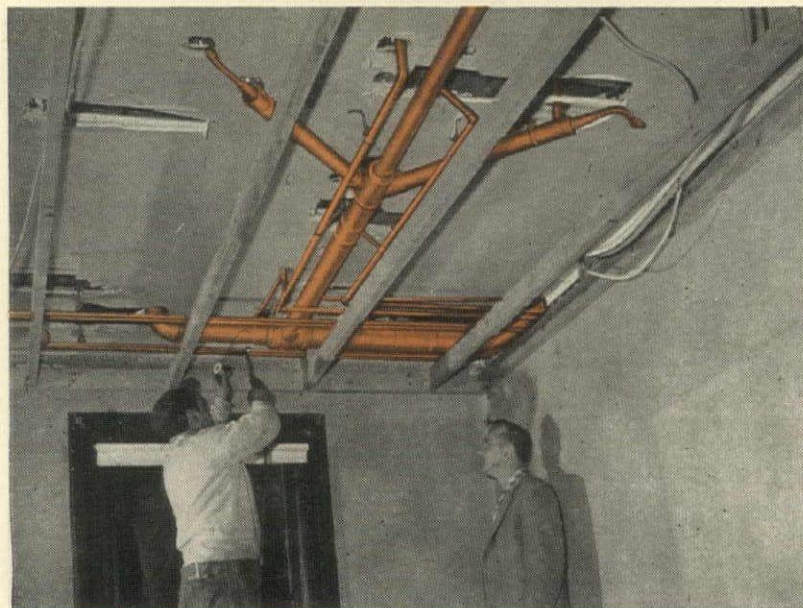
Simplify remodeling jobs. Lightweight copper tube and solder-joint fittings made light work of an otherwise back-breaking job, in adding two baths in this remodeled residence. Note how little ceiling height was lost.
