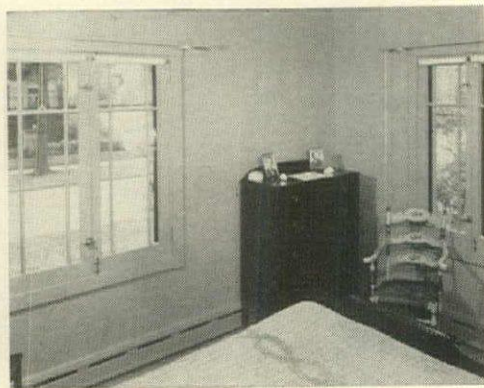
AFTER: Baseboard unit around outside walls provides better heat, takes up almost no bedroom space.
