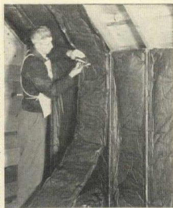
Bat insulation is good for attic remodeling, comes in standard widths to fit between rafters.
