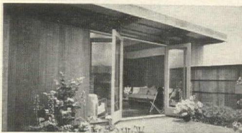
House in Carmel, Calif. Designers: Gordon Drake, San Francisco Stained with Cabot's Creosote Stain
