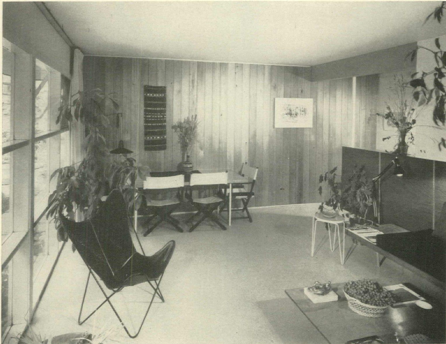
REMODELED HOUSE has the handsome look of a new house because of added textured surfaces. Architect Alexander Kouzmanoff specified vinyl floor tiles, 1 x 6 boards (on far wall) and a plywood room divider, right. This started as a typical expansion attic, postwar house.
