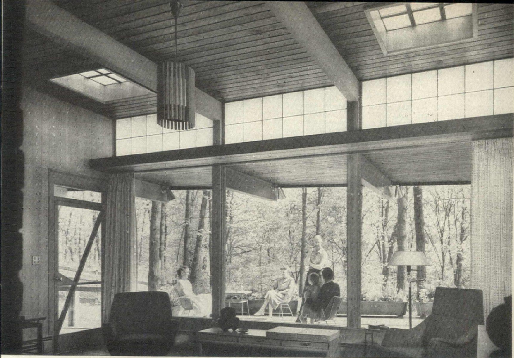
Clerestory and skylights made of the new block bring living room illumination to 60 ft-c. A partial roof for the porch shades the big clear-glass windows. Rear of the lot is heavily wooded, and the trees are extra protection against low-angle sun rays.
