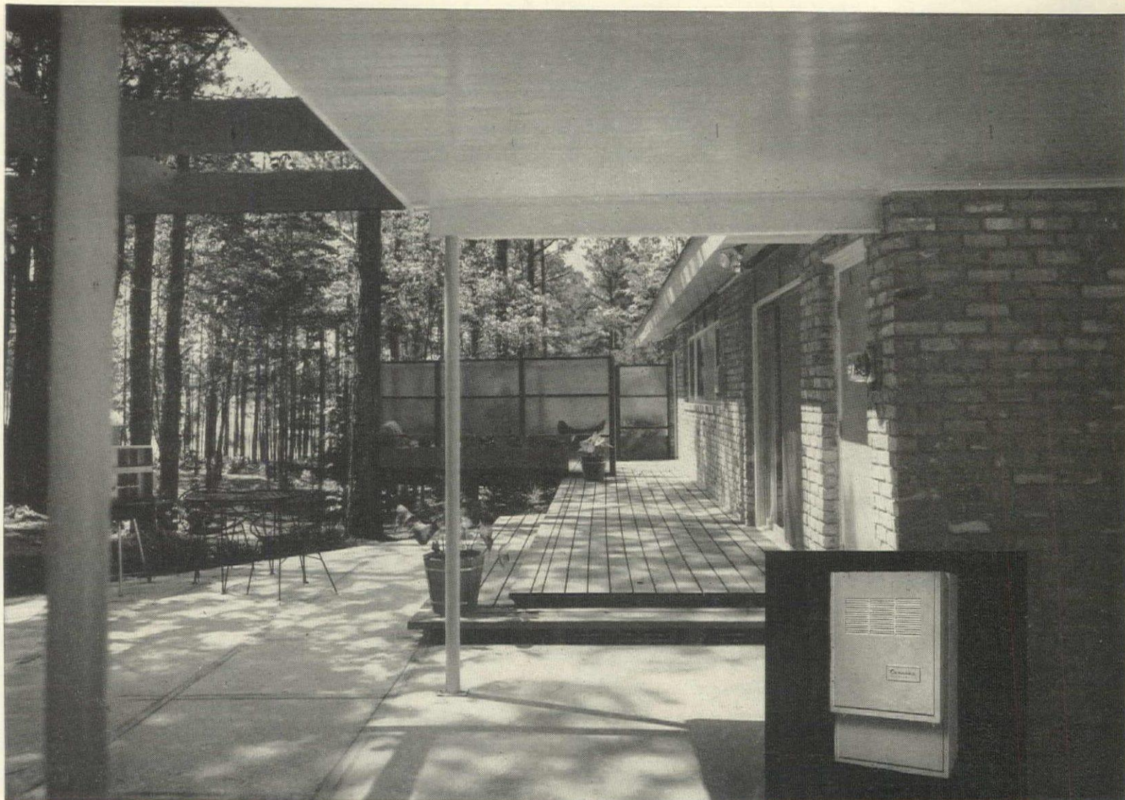
Patio of model home in Sexton Woods, Atlanta, Georgia. Builder: Boyd-Jackson Corporation. Architect Henry D. Norris made impressive capital of the Carrier air conditioning in these $17,000 and up homes.
