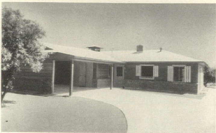
Phoenix. Bixby Construction Co. saved $148 on this 1,363 sq. ft. house by making changes that cut the heating-cooling bills to $143 a year.
