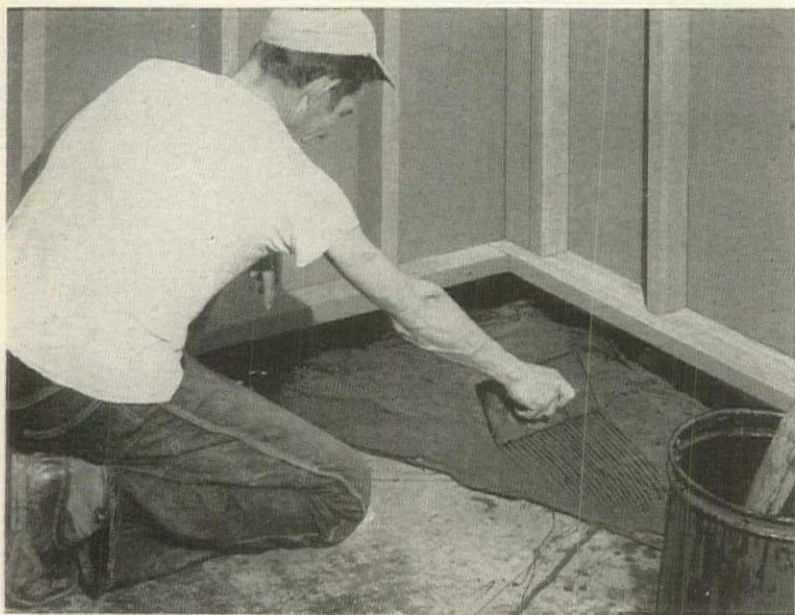
① Spread mastic over waterproofed slab.
