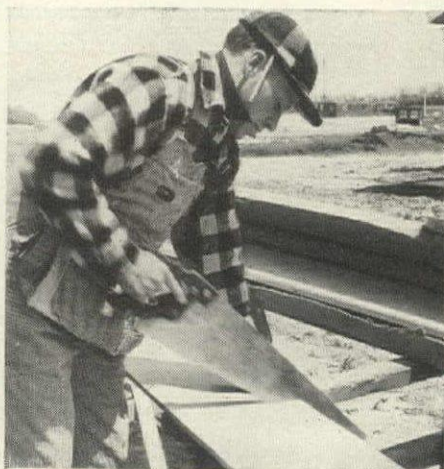
2 Duraply is easy to work... can be sawed with any saw used to cut plywood. Special overlay holds wood fibers tight—reduces edge splintering. Ten pieces of Duraply—pre-cut for lap siding—come in each carton (shown in back of workman).
