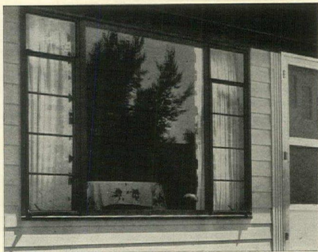
In this cottage, a fixed picture window is flanked by casement-type windows. Thanks to steel's rigidity and its freedom from warping, these casement windows will stay easy to open and close for many years of service. And occasional painting will keep them good-looking for the life of the house.
