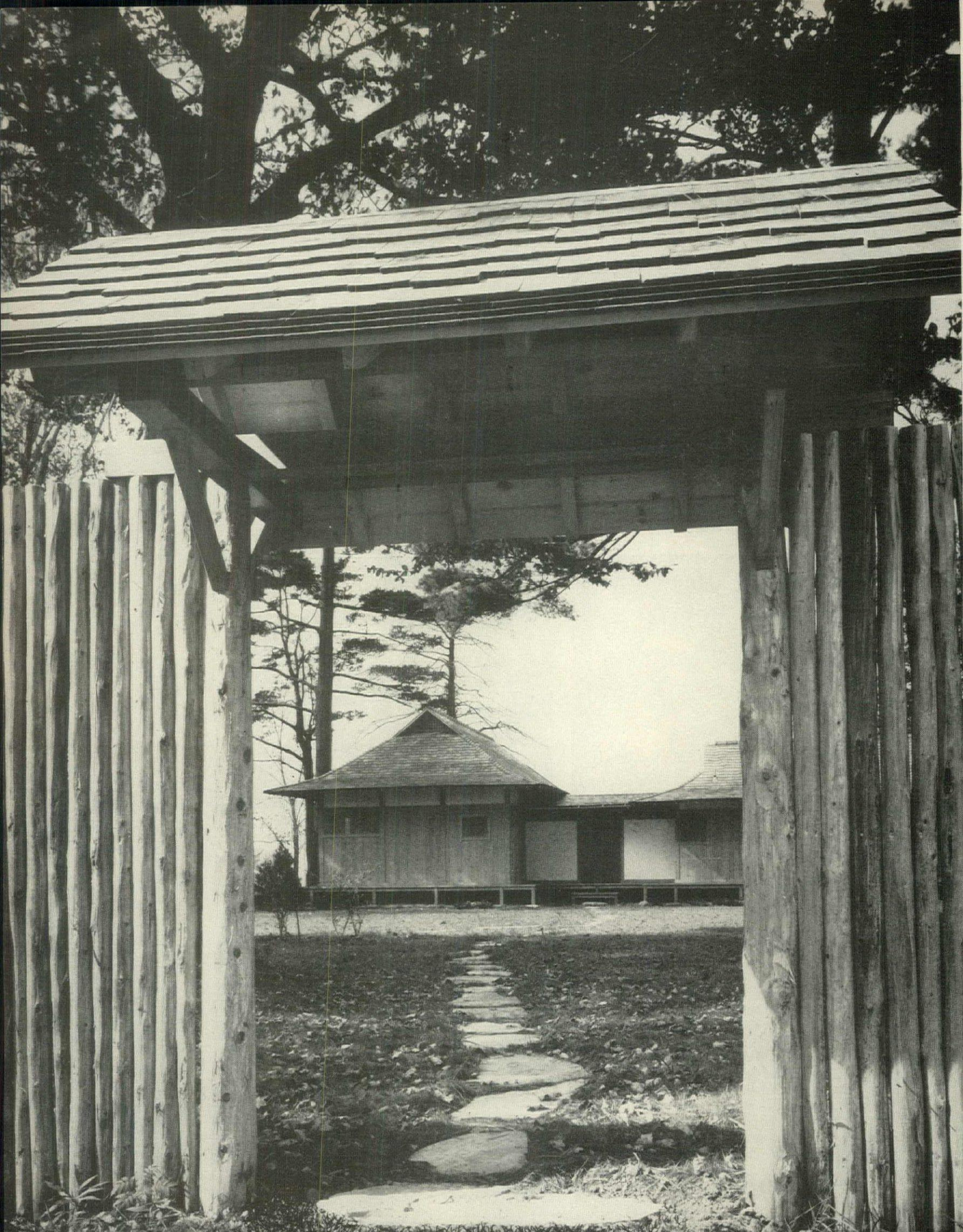
Typical Japanese garden entrance is roofed over, faces the road. House sits on posts which, in turn, rest on stones. Landscaping is still incomplete, may take years to finish properly.
