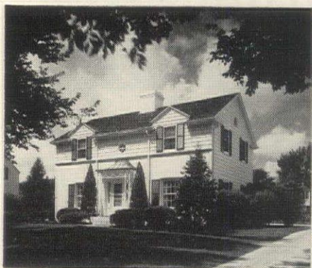
Relative inexpensiveness permits generous use of double hung wood windows with metal weatherstripping.
