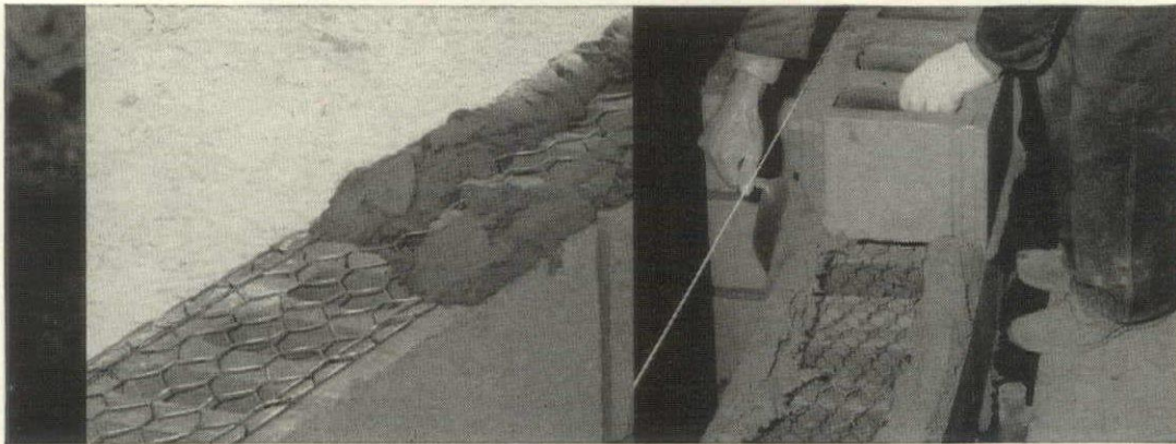
MORTAR FLOWS READILY around KEY-WALL to give full embedment, as well as maximum reinforcement value. Tests show an exceptional bond.
