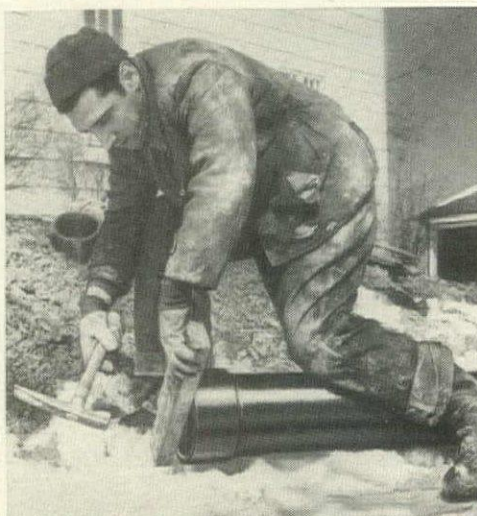
Joints are quickly and easily made by simply tapping together—no cement, no calking.
