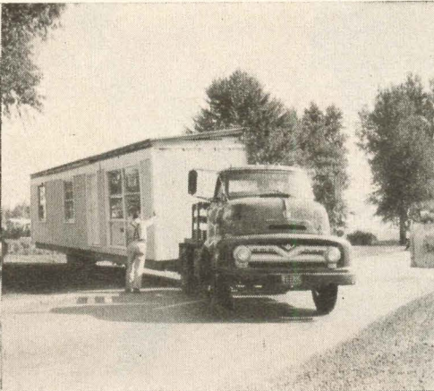
Low-boy trailer is backed on site.
