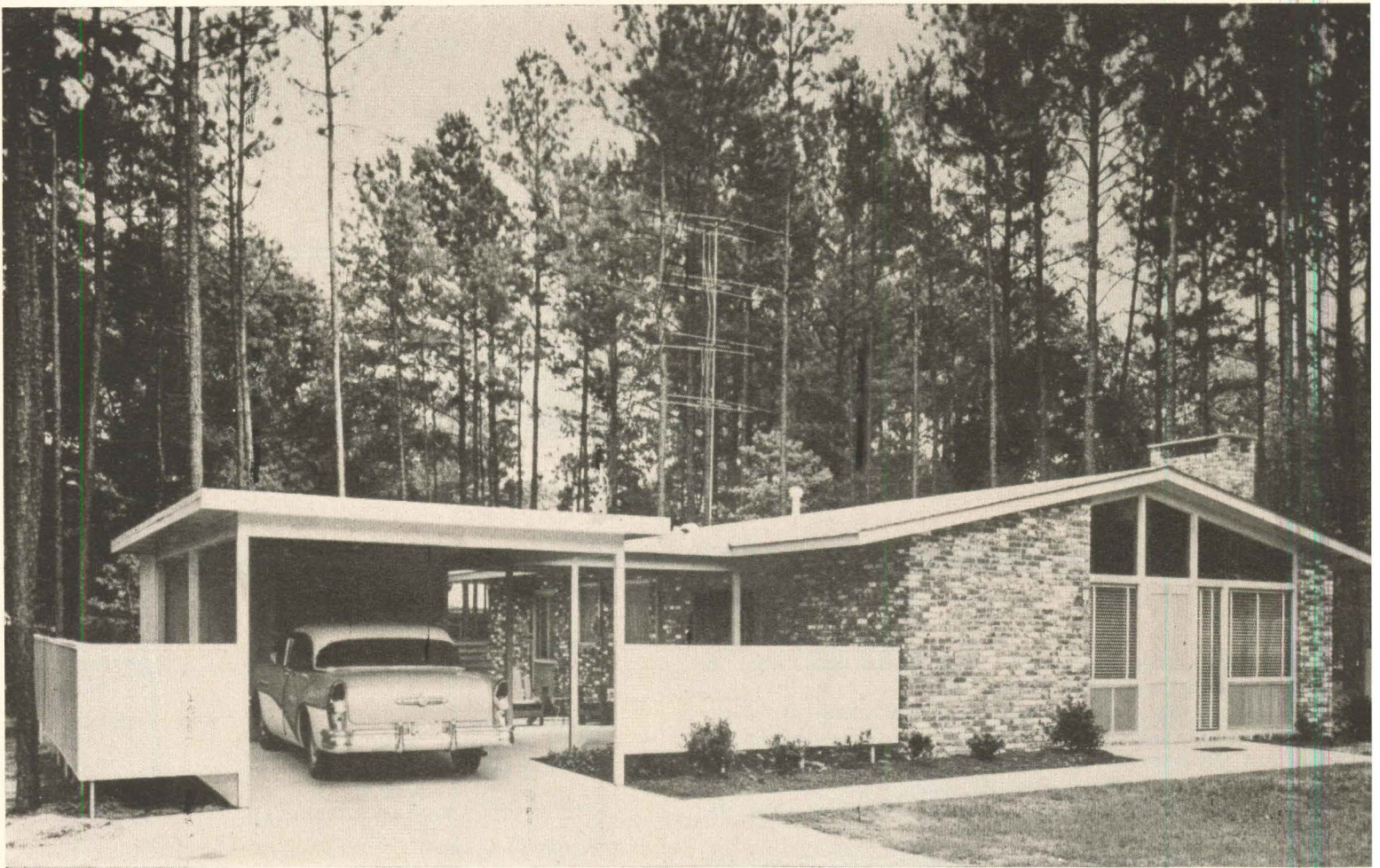
Carport and storage area is separated from family entrance by 12' covered walkway, forming a patio. Fencing screens the patio from street.
