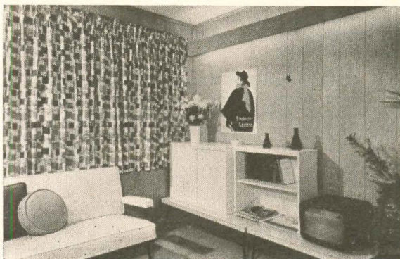
Living room walls show how random grooves hide joints.
