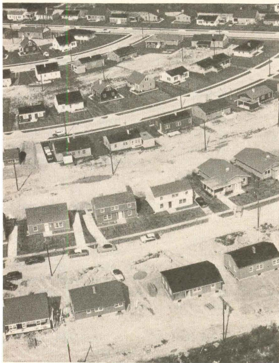
Variety of models made possible by use of prefabs is shown in this photo of Lincoln Village, Columbus, Ohio. Midwest Homes put over a dozen models in the project.
