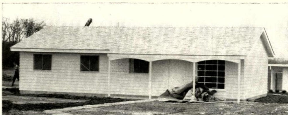
$10,945 MODEL with four bedrooms has neither garage nor carport, no basement, gutters or downspouts, but offers 1,162 sq. ft. of living area. Lots average 75' x 180'. The tract is to be served by builder-owned water and sanitary sewage disposal systems.
