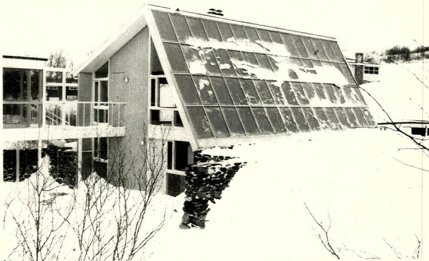
FROM SOUTH new MIT solar house is one big (40' x 16') heat collector, tilted at 60°—perpendicular to winter sun in this latitude.
