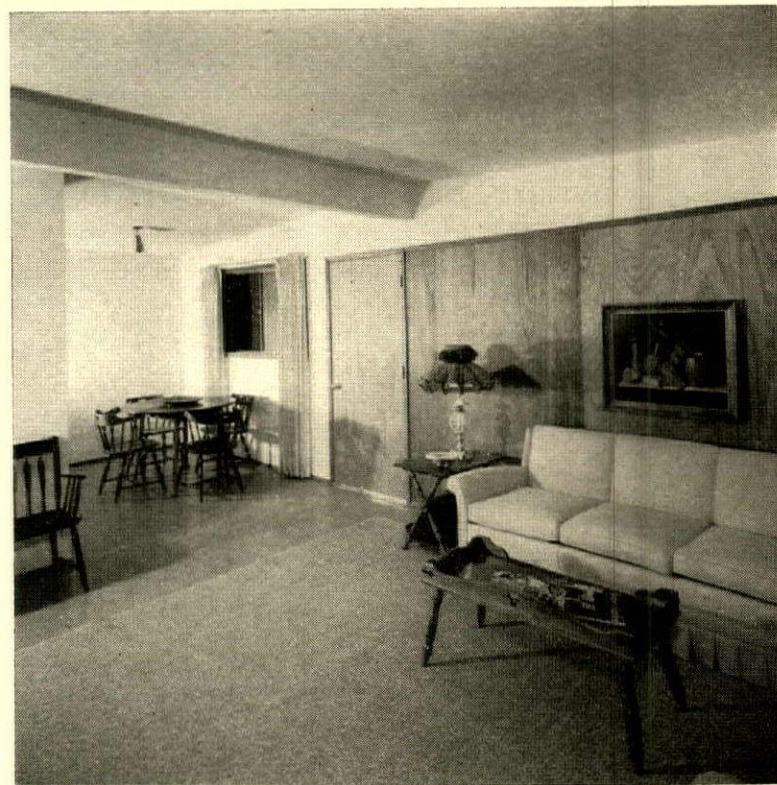
One side of living room has 8'-high mahogany plywood paneling. In earliest model, living room opened directly on kitchen.
