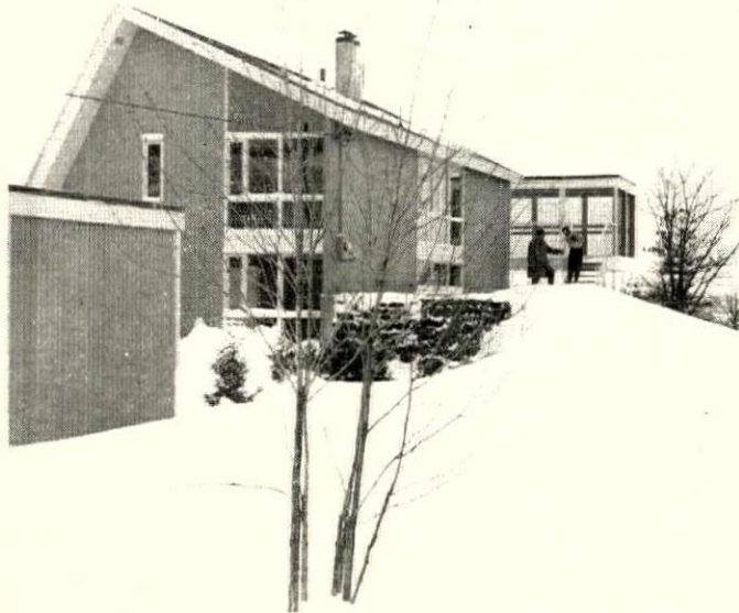
FROM NORTH-EAST house looks much like an ordinary Contemporary. Construction and insulation are mostly standard. But wall supporting collector is extra heavy (2x10s, 16" o.c.), and earth mounded against north and south walls cuts heat loss.
