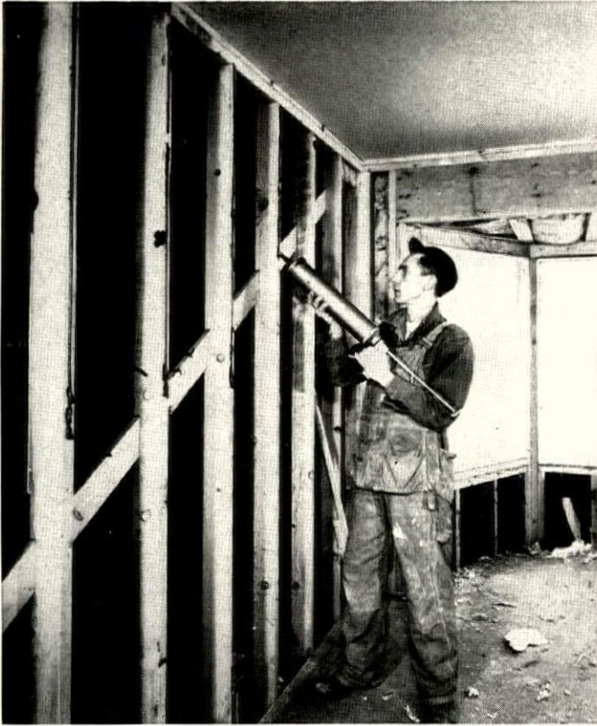
STEP 1: Apply a bead of a new adhesive to the framing members...
