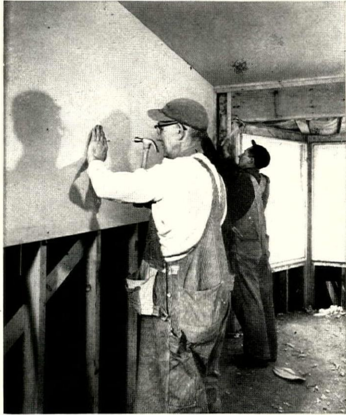
STEP 2: Press the wallboard into place and nail it. Result:
