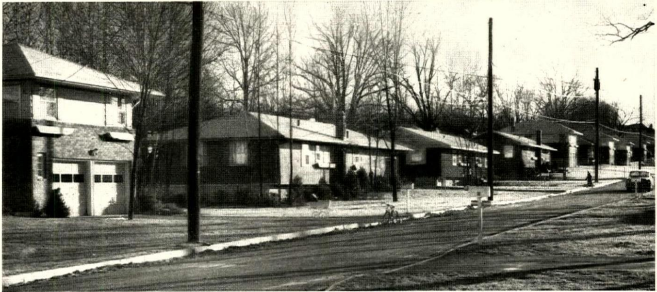
General Electric Thinline air conditioners are one of the most talked about sales features of these Sherman Woods Homes.
