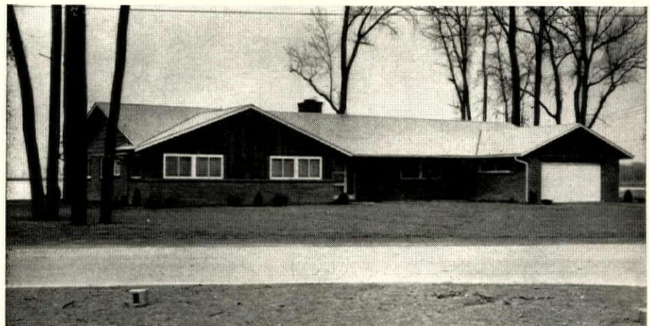
$50,000 HOUSES and others ranging up to $75,000 are built by Sandusky Development Co. All are oriented to get the best views.
