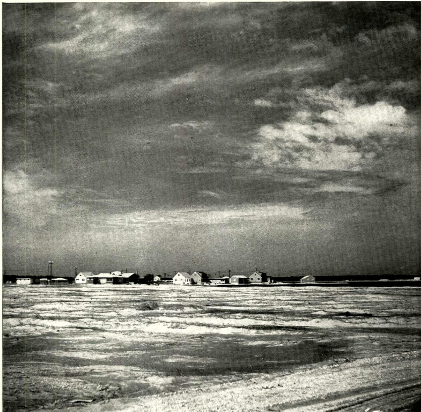
42" OF SAND was pumped onto marshland to build up Windsor Park tract on Barnegat Bay off the New Jersey mainland.
