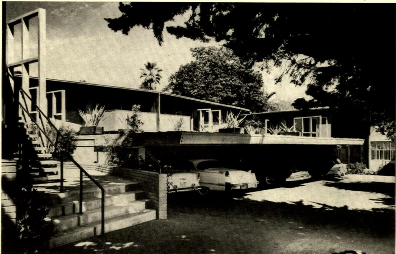
UNUSUAL CARPORT has rooftop garden used by tenants of upper-level apartments. Large trees in right foreground were kept to shade gardens and entrance driveway. Architects: Howell & Arendt and Neal Butler. Builder: W. S. Hamilton, Santa Barbara, Calif.
