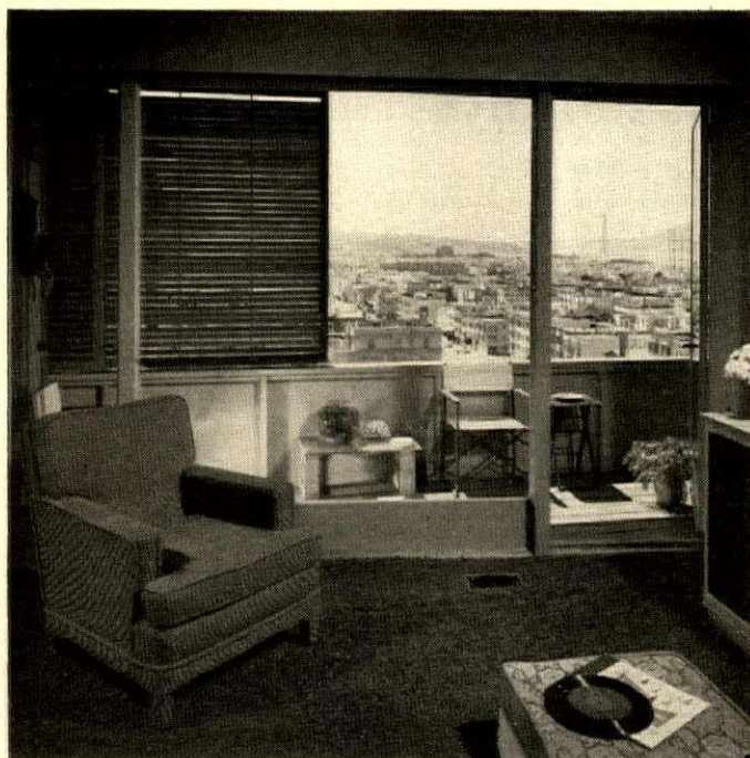
SLIDING LOUVERED SCREENS , partly open at left and closed at right, protect from glare. Use of other sun controls (overhangs, sun-
