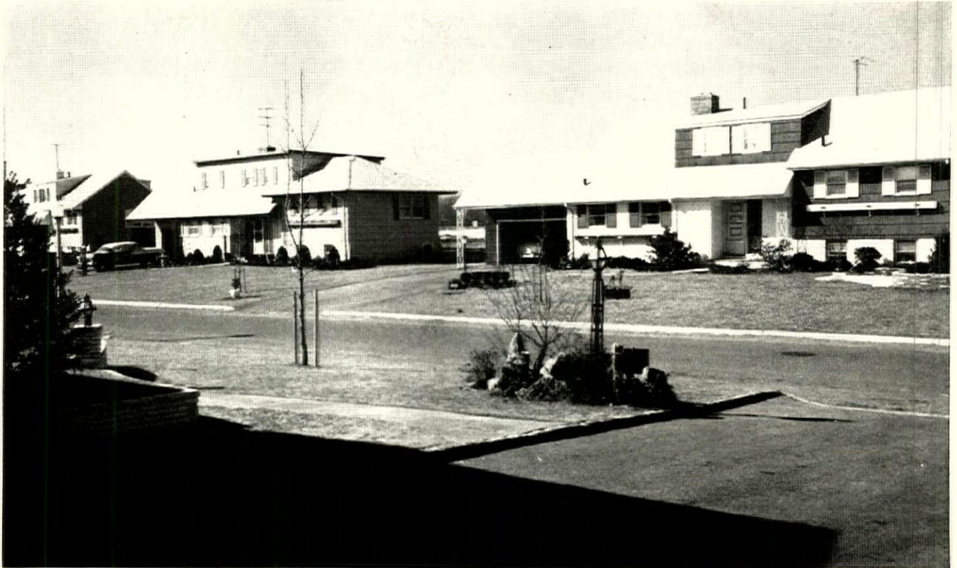
LAWRENCE BAY PARK TRACT includes split-level, ranch and contemporary houses designed by Architects Schuman & Lichtenstein.
