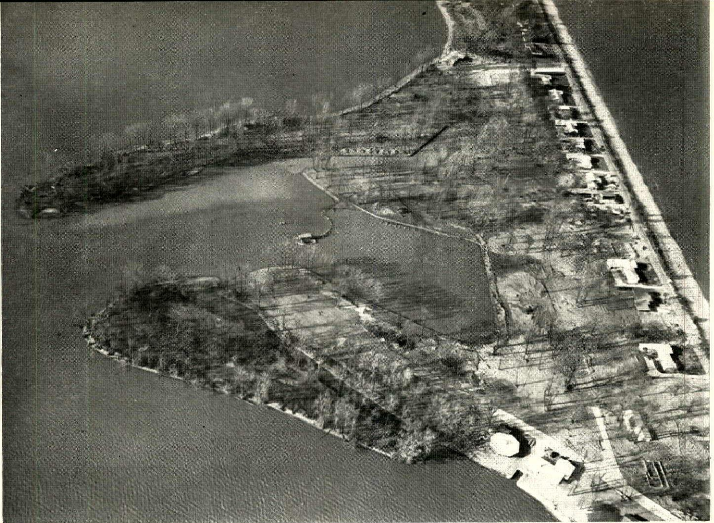
RECLAIMED LAND FOR HOUSES is created on a narrow, marshy sandpit off Sandusky, Ohio by hydraulic dredge (shown in cove), which pumps 135 cubic yards of fill an hour through 8" pipe. Land at lower left in photo will be developed as a park with a boating harbor.
