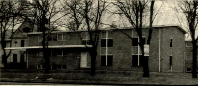
Arch.: Irwin Baker. Buldr.: Frank E. Cooper. Developer: Lou Heller. Baltimore H&H staff
