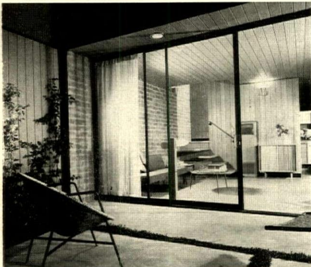
PATIO is outdoor living room. Glass wall, set back from face of building, uses upper floor as overhang. Designer: Craig Ellwood. Builder: Henry Salzman. Hollywood, Calif.
