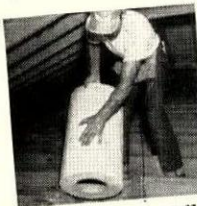
One man can install a Van-Packer in 3 hours—saves on labor costs.
