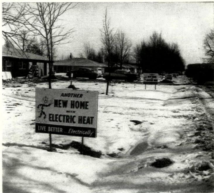
Medallion homes now under construction at the "Swanson Highlands" subdivision. Every home has its own sign featuring electrical living.
