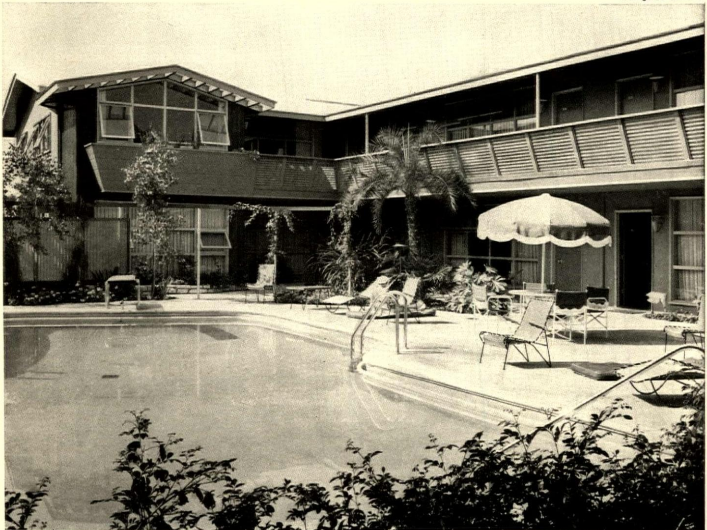
SWIMMING POOL is in center of O-shaped apartment building. Balconies serve as public corridors for second-floor apartments, are covered
