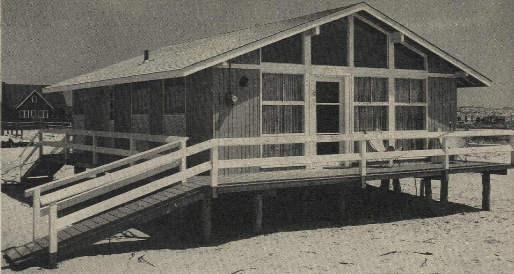
BEACH HOUSE sits on sturdy pile foundation. Roof shingles are glued and nailed to withstand high winds.
