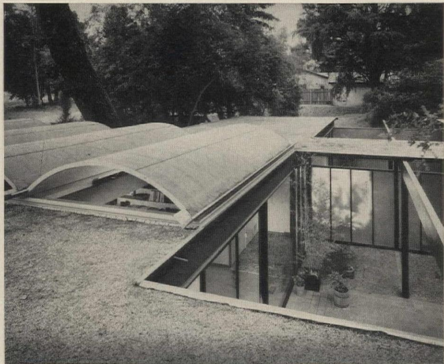
VIEW FROM ROOF clearly explains relationship of vaulted dining area to open dining court. Roof plane across court is over entrance walk.
