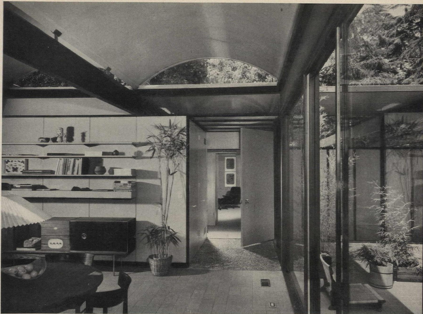
VAULTED DINING AREA is off main entry. Graveled entrance walk continues right into the house. Roof vaults with glass-filled ends open
