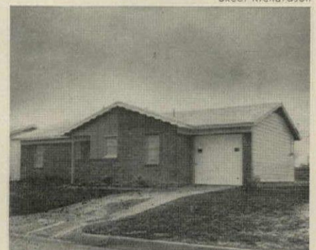
costs from this plan. At right is photo of the house as later built and financed through FHA.
