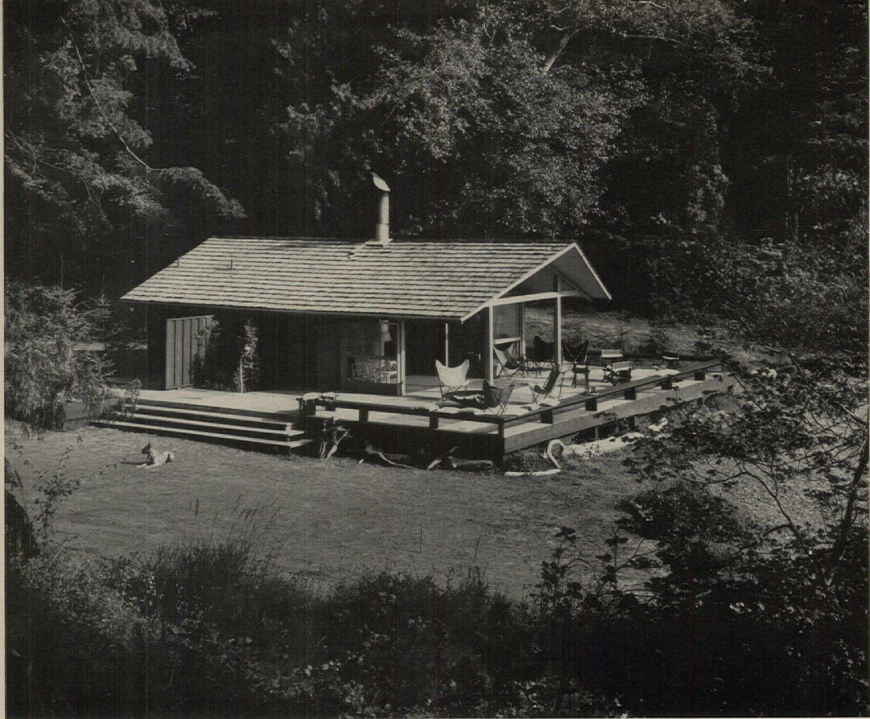
HOUSE HAS THREE MAJOR UNITS: the huge platform, the somewhat smaller roof above, and the very small area under the roof.
