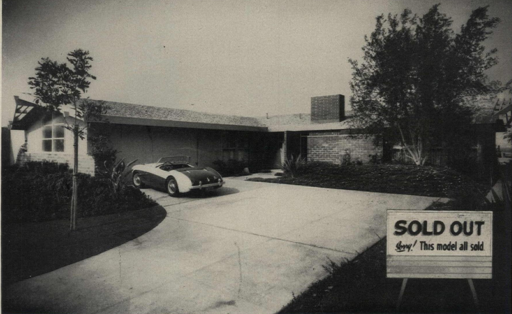
FROM STREET , the $19,300 "Golden Estate" looks impressively large. Roof is built-up with rock topping, has trellised gable-end overhang.
