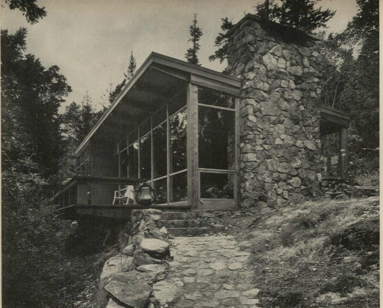
NATIVE STONE used in fireplace and lower walls anchors house into slope. Roof overhang shades living room windows and part of deck.
