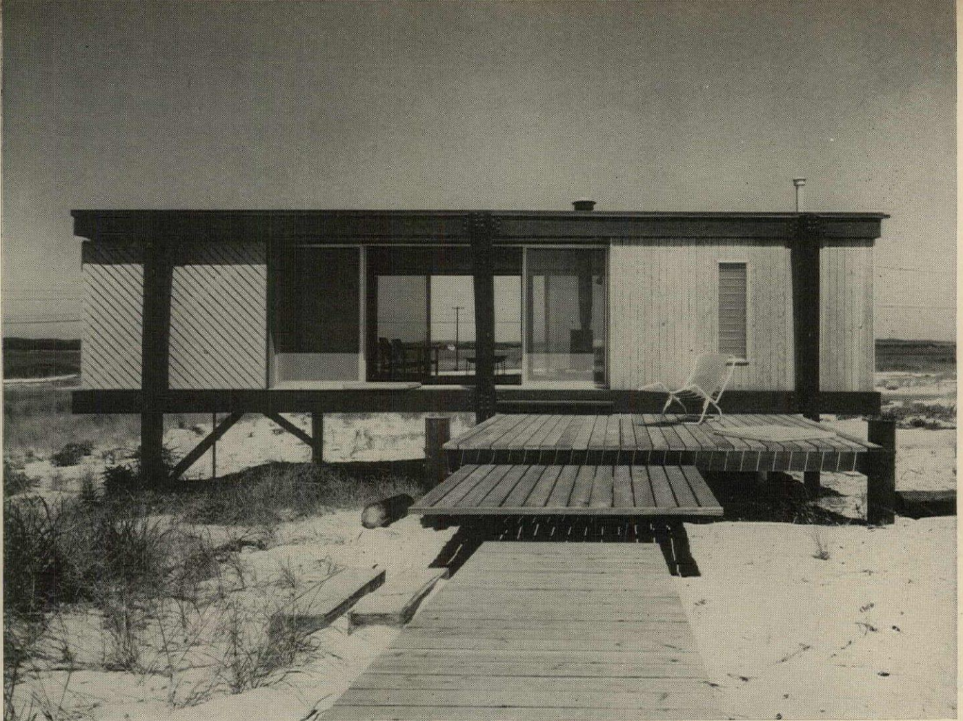
OPEN DOORS stack at left, making center of house a breezeway. Sliding glass walls are set back 2½' so they are shaded from sun.
