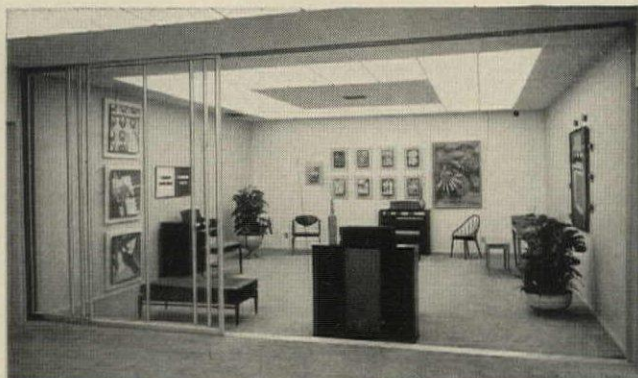
Multiple sliding "pocket" installation is the Ador Flush Threshold door shown in this smart studio salesroom. Threshold sets in slab or mounts on sub floor.
