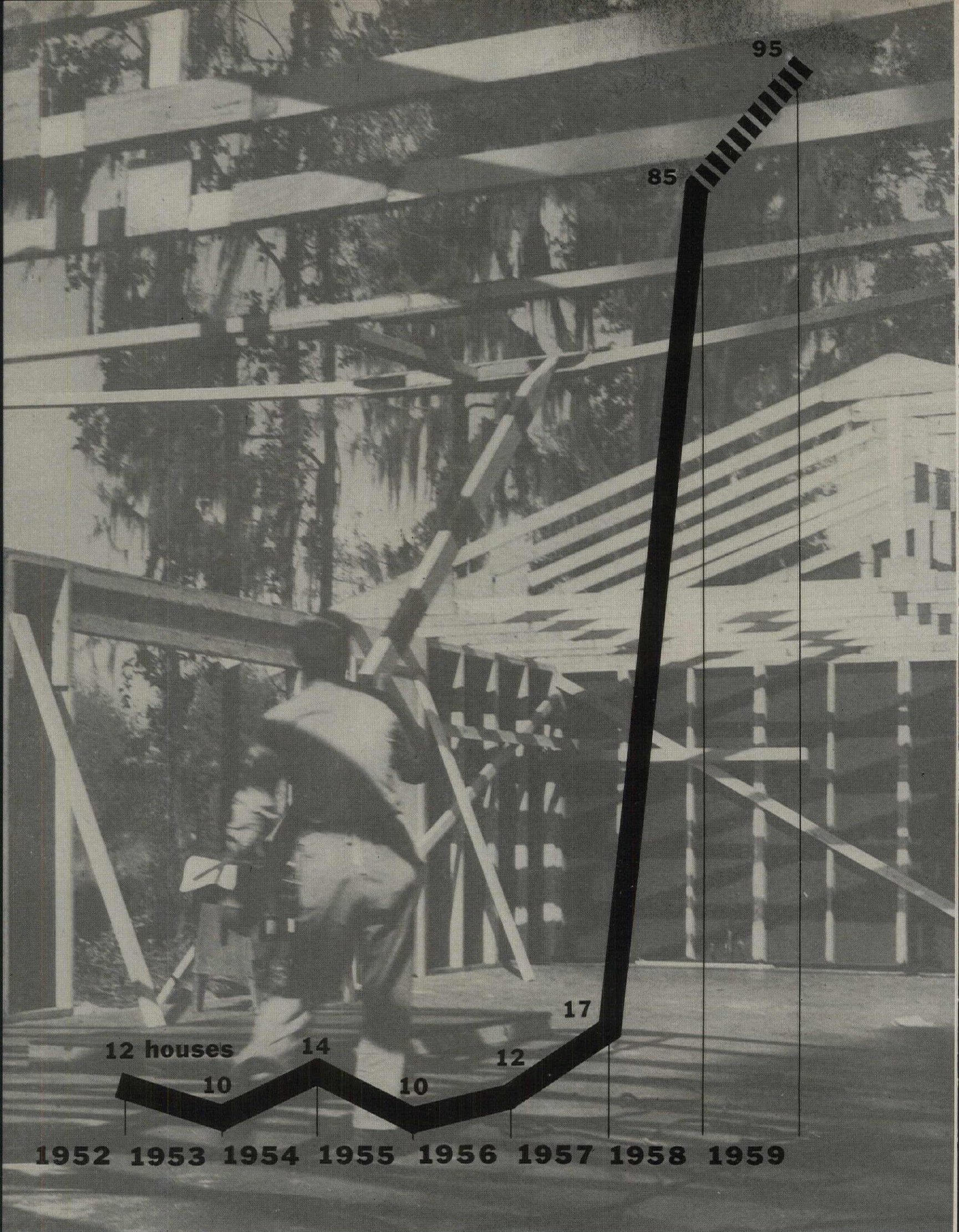
HOUSE PRODUCTION skyrocketed for Builder Dyches when he switched to components and started building on a 15-day schedule in mid-1957.
