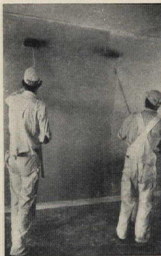
TWO COST CUTTERS: long-handled paint rollers, and a suspended soffit that eliminates horizontal 2x4 lookouts (H&H, Jan p 198).
