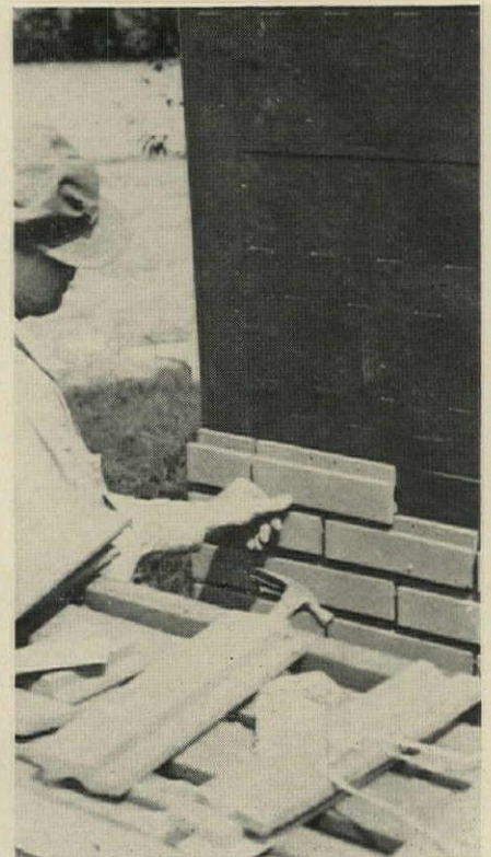
Use 6" bricks in bearing wall . . . use 4" brick in reinforced panels . . . or nail on thin bricks for veneer
