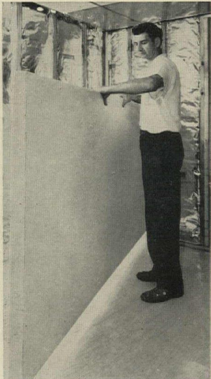
BIG CEILING PANEL is easily handled by one man. Two-mil vinyl face resists soiling.
