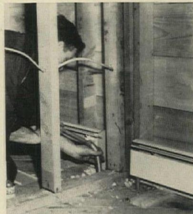
FLEXIBLE CONNECTORS are sweated to the baseboard, then pushed through a hole in the floor to join piping below.
