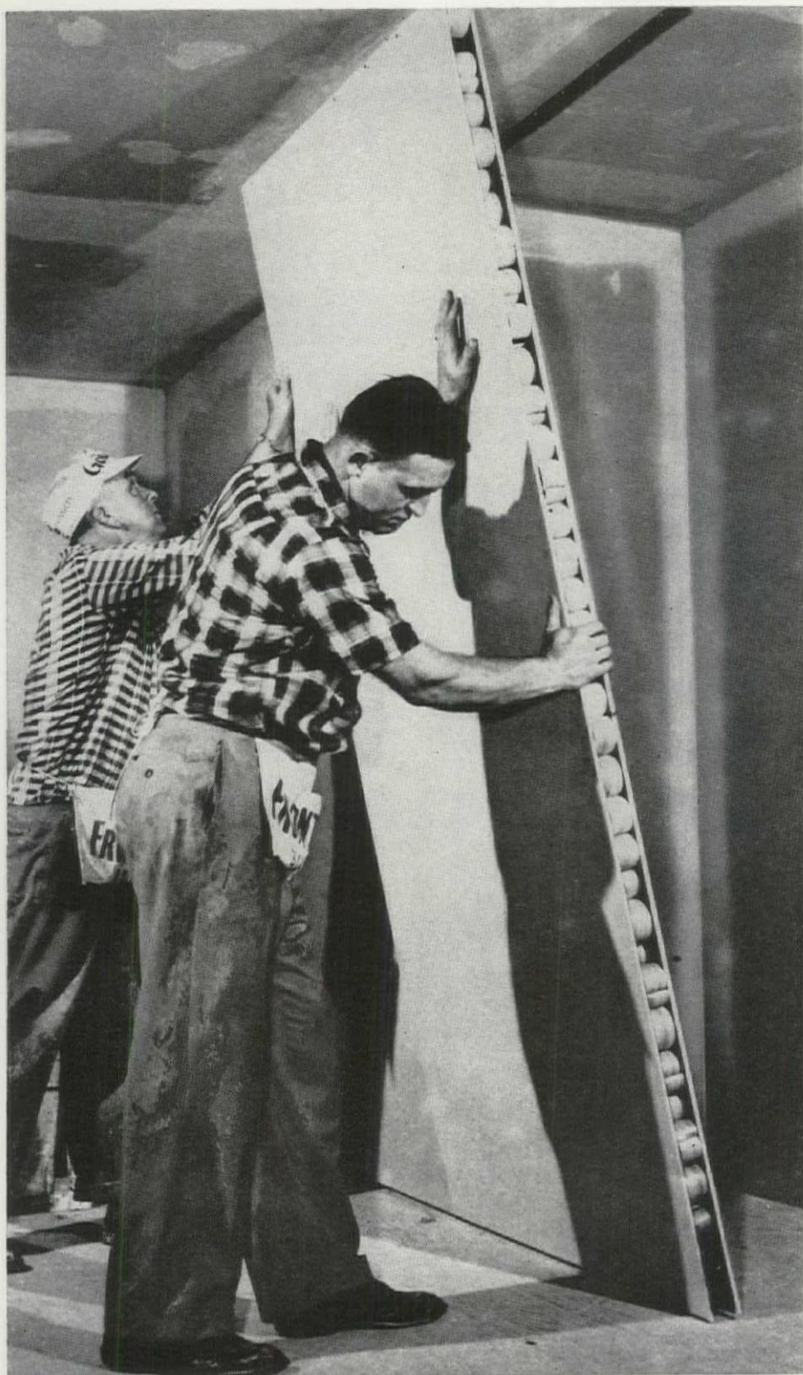
SPIRAL CORE PANEL is placed by two men who can partition a typical house in a few hours. Panel rests over a 2x2 centered on a \frac{3}{4} "x2 \frac{3}{8} " sill. Built-in header is also 2x2.
