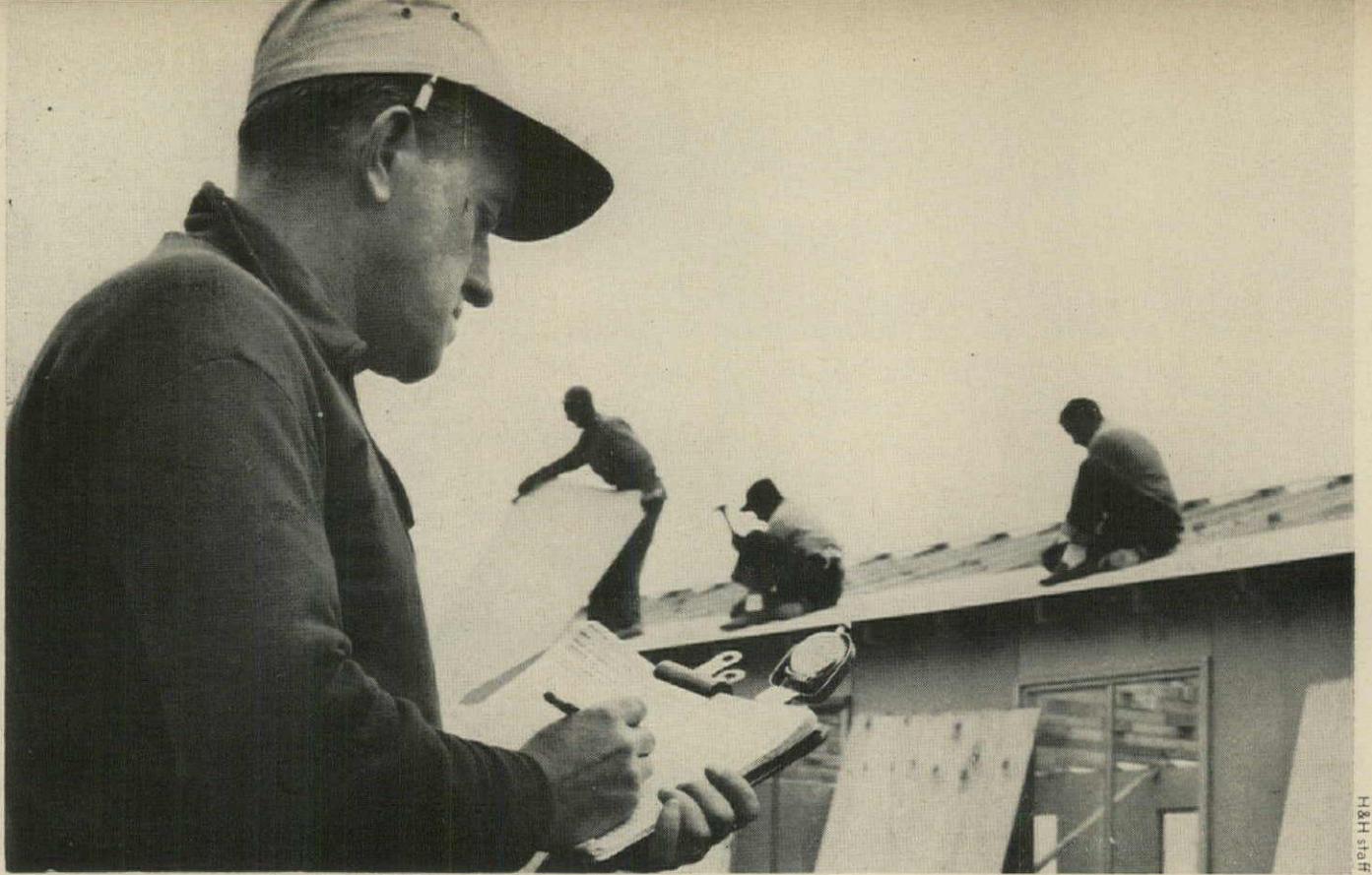
TIME STUDY MAN lists what each man does and how long it takes, so later analysis can show where time is being wasted and raise productivity.
