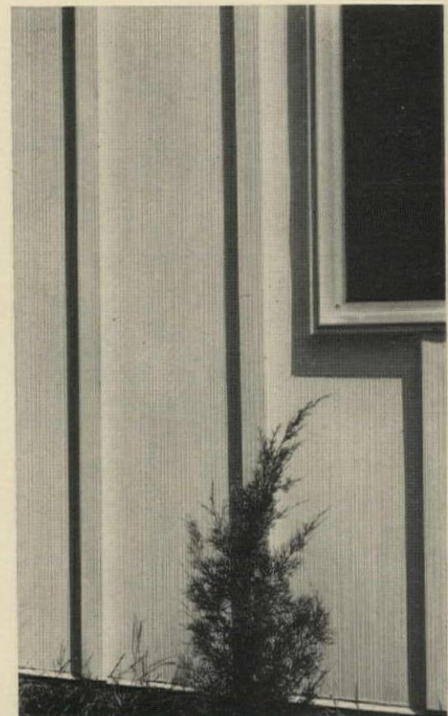
ALUMINUM BOARD-&-BATTEN is made from sheets fastened to plywood. Battens snap on.
