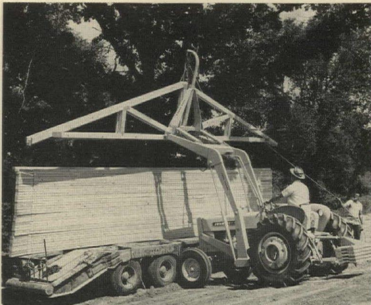
Loader hook lifts trusses, puts them on the house.
