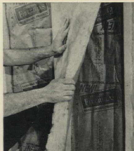
SOUND-CONTROL BLANKET for stud wall also installs by friction-fit method. (No. 6)
