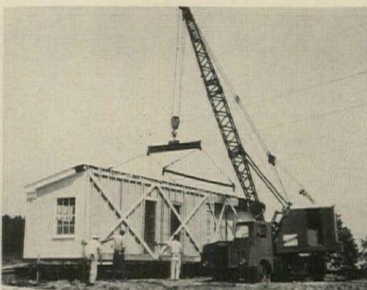
prefabs in three sections (17,000 lb) . . .
