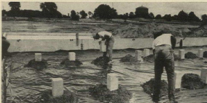
CONCRETE BLOCKS , intermediate support for joists, are set to lines.
