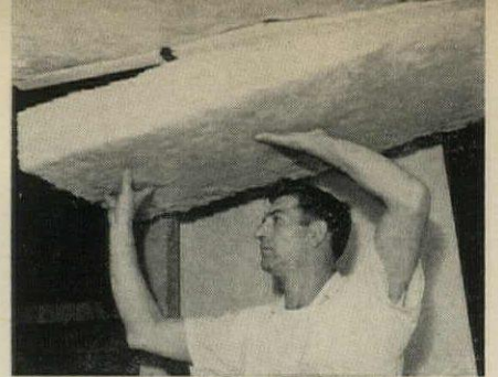
CEILING BATTS are self-supporting. With roof vents, no vapor barrier is needed.
