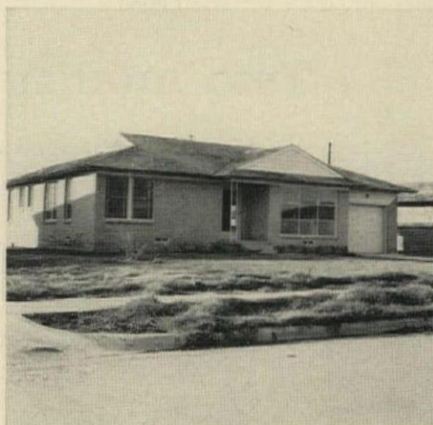
GABLE-END LOUVERS like these seldom look well in hip-roof houses.
