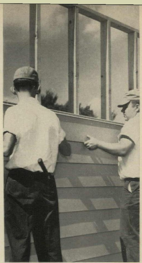
ALUMINUM CLAPBOARD needs no sheathing with foam, fiberboard, or fiberglass backing, says FHA.
