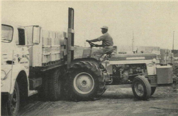
Fork lift on tractor carries masonry pallets.
