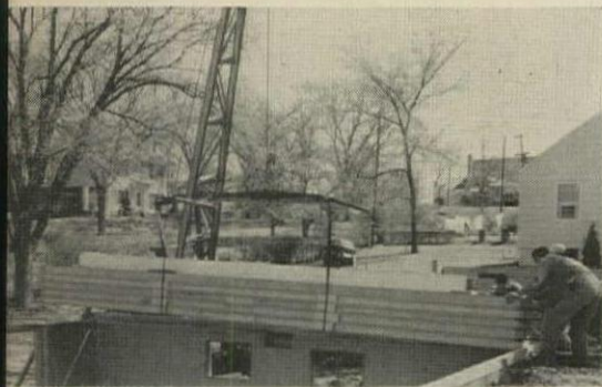
house-width floor panels (460 lb) . . .
