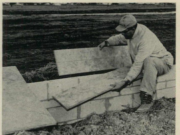
PERIMETER BOARD breaks easily at score line or can be folded against foundation. Fiberglass costs less than plastic-foam boards. (No. 3)
