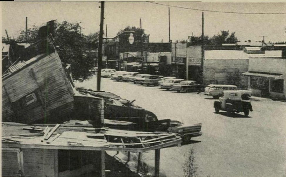
FIRE-DAMAGED BUILDING totters on Wink's main street. Owner says it is worthless but renewal authority paid generous price for it.
