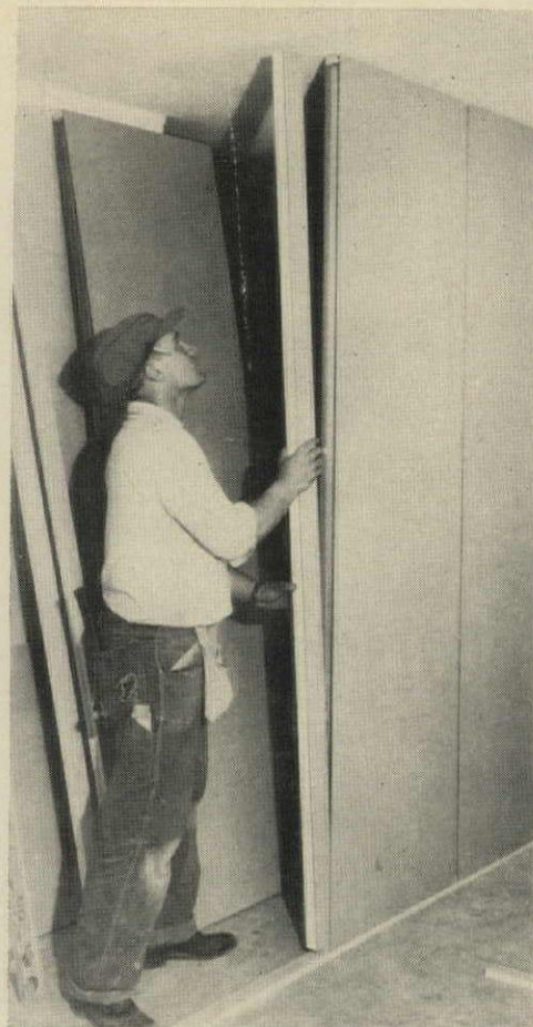
SPLINE fits into recessed edge. It has same surface as panels, is ripped from 4'-wide sheet, can be as wide as desired to stretch out wall.
