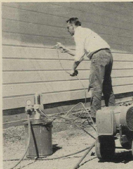
spray walls on the site or . . .
