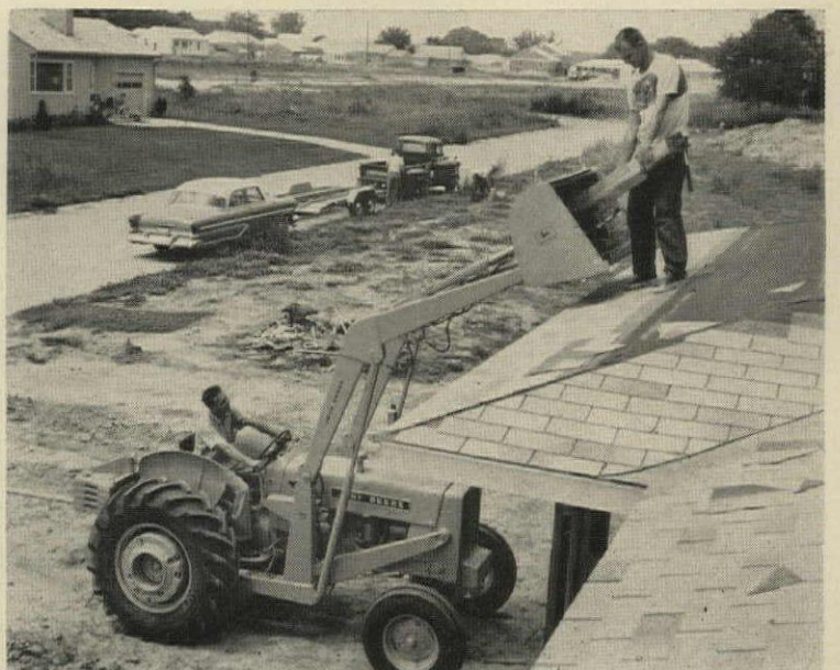
Loader bucket puts shingles on the roof.
