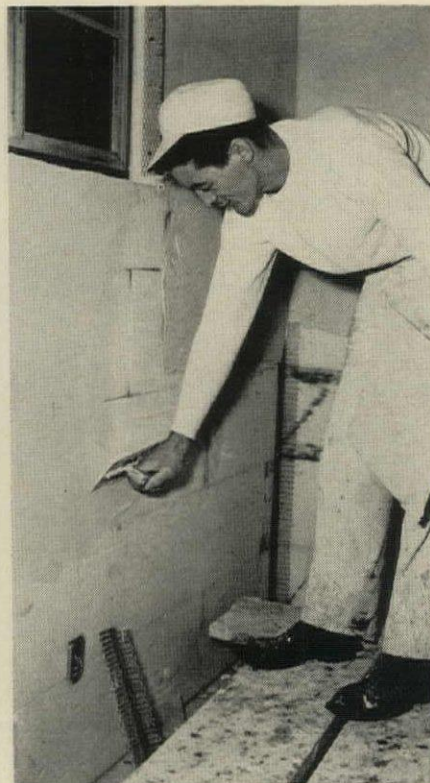
and plaster or drywall it . . .
