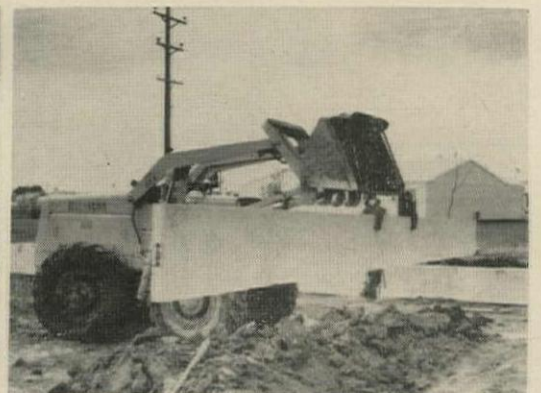
precast concrete grade beams (4,000 lb) . . .
