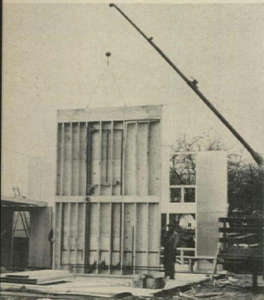
two-story plumbing walls (600 lb) . . .
