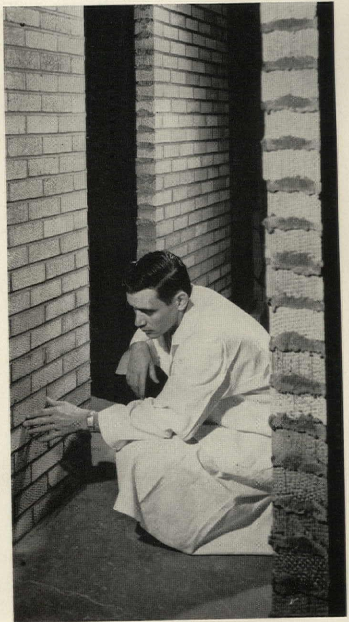
BRICK WALLS are laid up only one wythe (one brick) thick for bearing. Tight mortar-brick bond provides good waterproofing.
