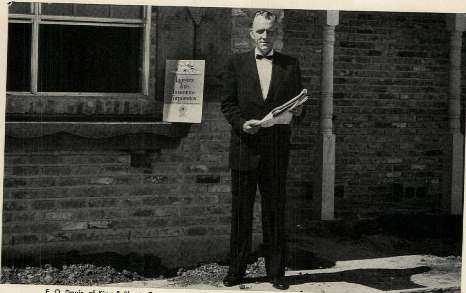
E. O. Davis, of King & Sheets Company, checks the finishing touches on a Houston home nearing completion.
