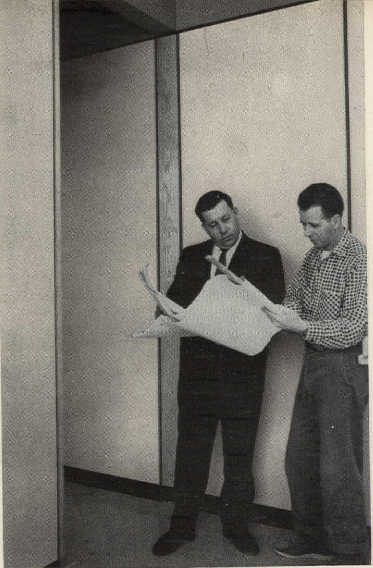
Project superintendent Donald Carson, right, indicates other areas in school where Filled Timblend panels were used for interior fascia.
