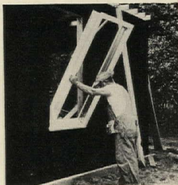
One man can install all but largest R-O-W units, with sash removed for easier, safer handling
