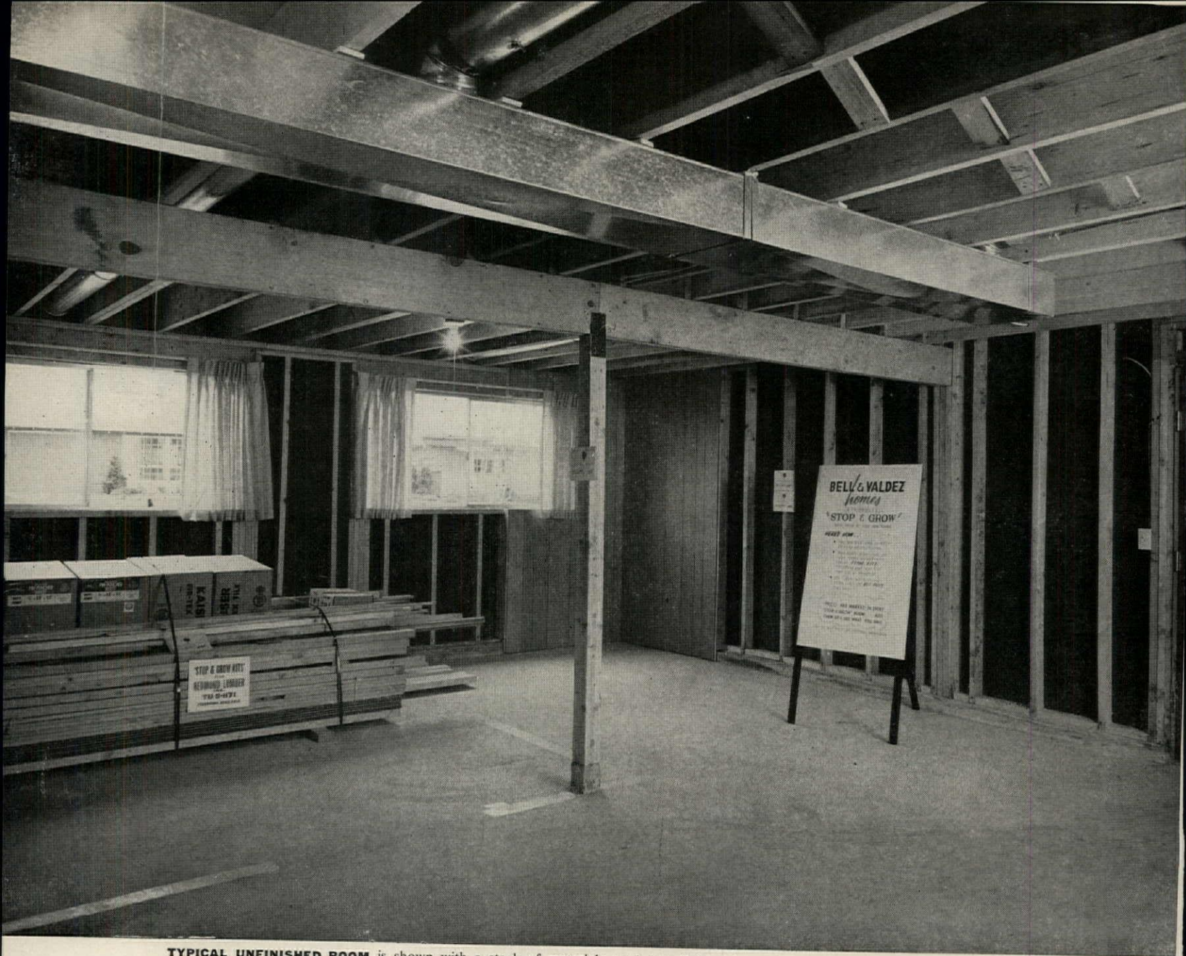
TYPICAL UNFINISHED ROOM is shown with a stack of materials needed to finish job; section of wall is up to show how it's done.
