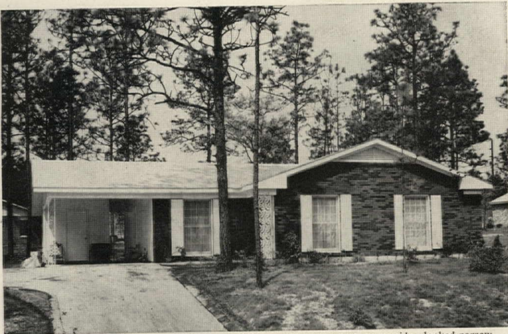
FIRST MODEL —with its broken roof line, vertical lines, and open carport at one side—looked narrow.
