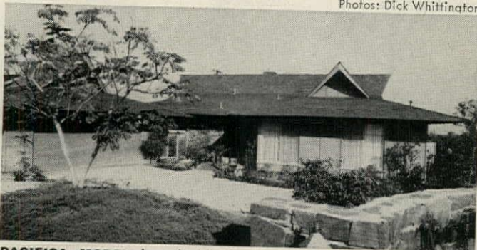
PACIFICA MODEL has double-pitch roof, horizontal siding divided into 4'-wide panels, and an extra-wide garage.
