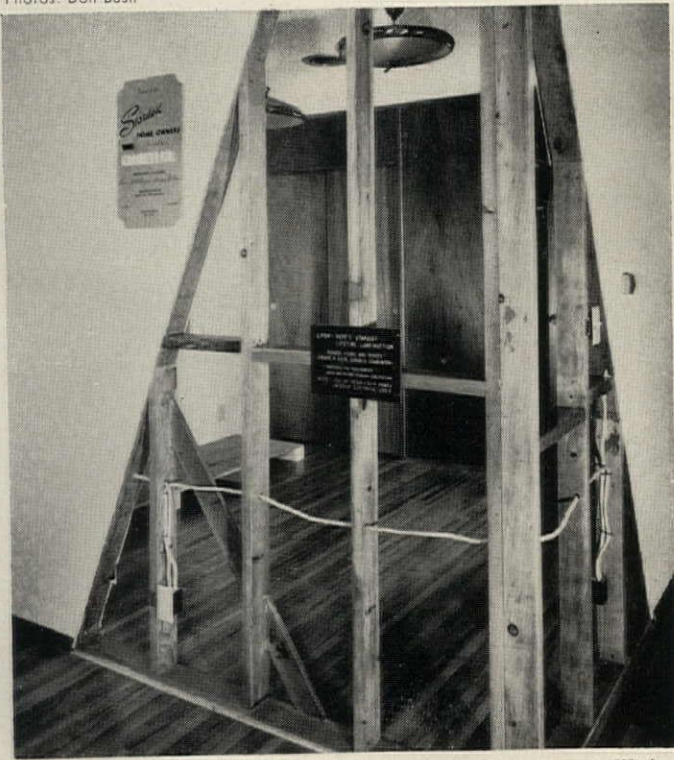
PARTITION CUT-AWAY has sign: "Look! Here's Stardust lifetime construction. Rugged studs and bracing create a solid, durable framework. Note use of heavy-duty, durable interior electric cable."
