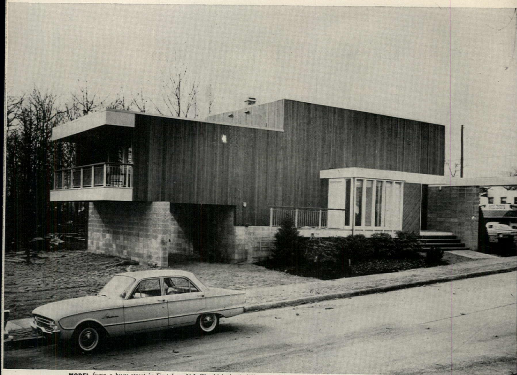
MODEL faces a busy street in Fort Lee, N.J. The high-rise buildings are located on the far side of the 32-acre site, overlooking the Hudson River.
