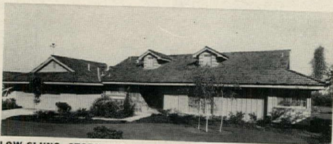
LOW-SLUNG STORY-AND-A-HALF has textured finish characteristic of all models in Weatherstone subdivision.
