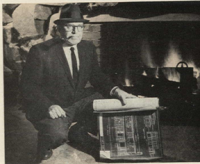
Leonard J. Schear, developer and builder of Northmoor Club Estates, checks restoration work in the 90-year-old Hearth Room of the Country Club.
