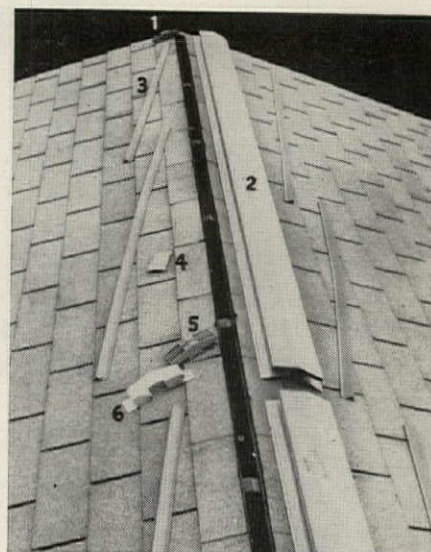
RIDGE VENT provides a continuous opening at peak of roof, has guards to keep out snow.
