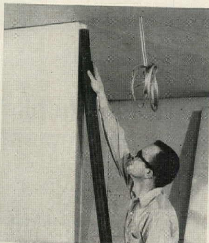
4 Full-length tubular spline is inserted in open edge of starter panel, then tapped lightly with palm of hand to assure snug fit.
