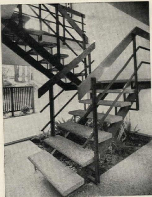
OPEN STAIRWELL , in typical model borrows space and light from two-story glass wall.
