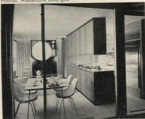
Compact kitchen is open to informal dining area and playroom. Cabinets are teak. Floor is white, matt-finish ceramic tile in 1½" squares.
