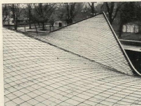
REINFORCING is set on chairs on mortar screed.
