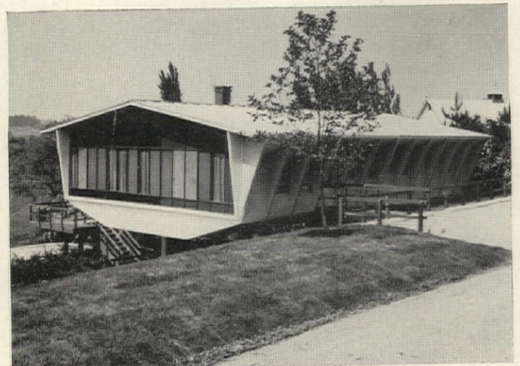
12 Finished house seems to float on hillside. Except for acrylic and hardboard panels on end wall, unglazed exterior is all aluminum.
