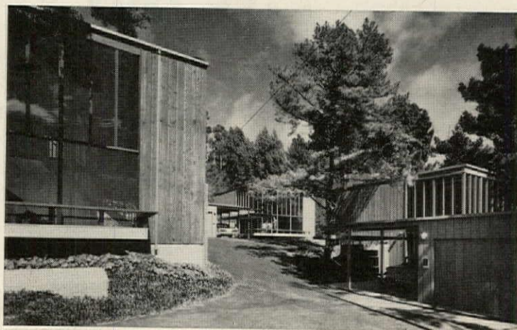
Three houses, seen here from entry road, were placed at different levels on sloping land but sited so that all glass walls face north and west.
