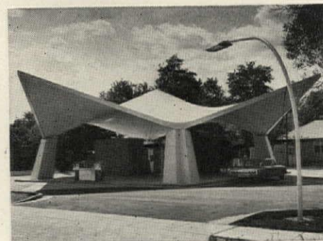
FINISHED ROOF floats on its four supports.
