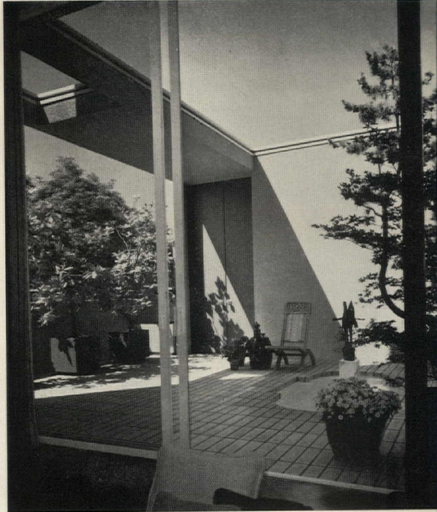
Slender roof slab with decorative cut-out spans court from front door to main building (foreground). Walls are machine-applied plaster.
