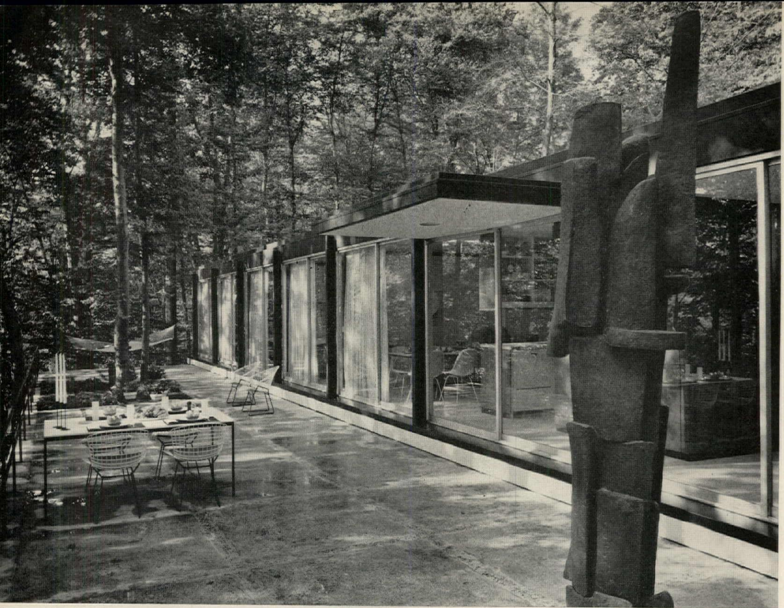
Glass doors across rear of house open every room to 90' terrace. Trees shade rooms in summer. Southwest orientation gains solar heat in winter.
