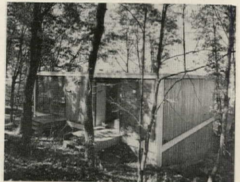
Upper floor of house opens to grade at rear. Dining room is at left, kitchen in center, living room at right. Siding is unfinished t&g cedar.
