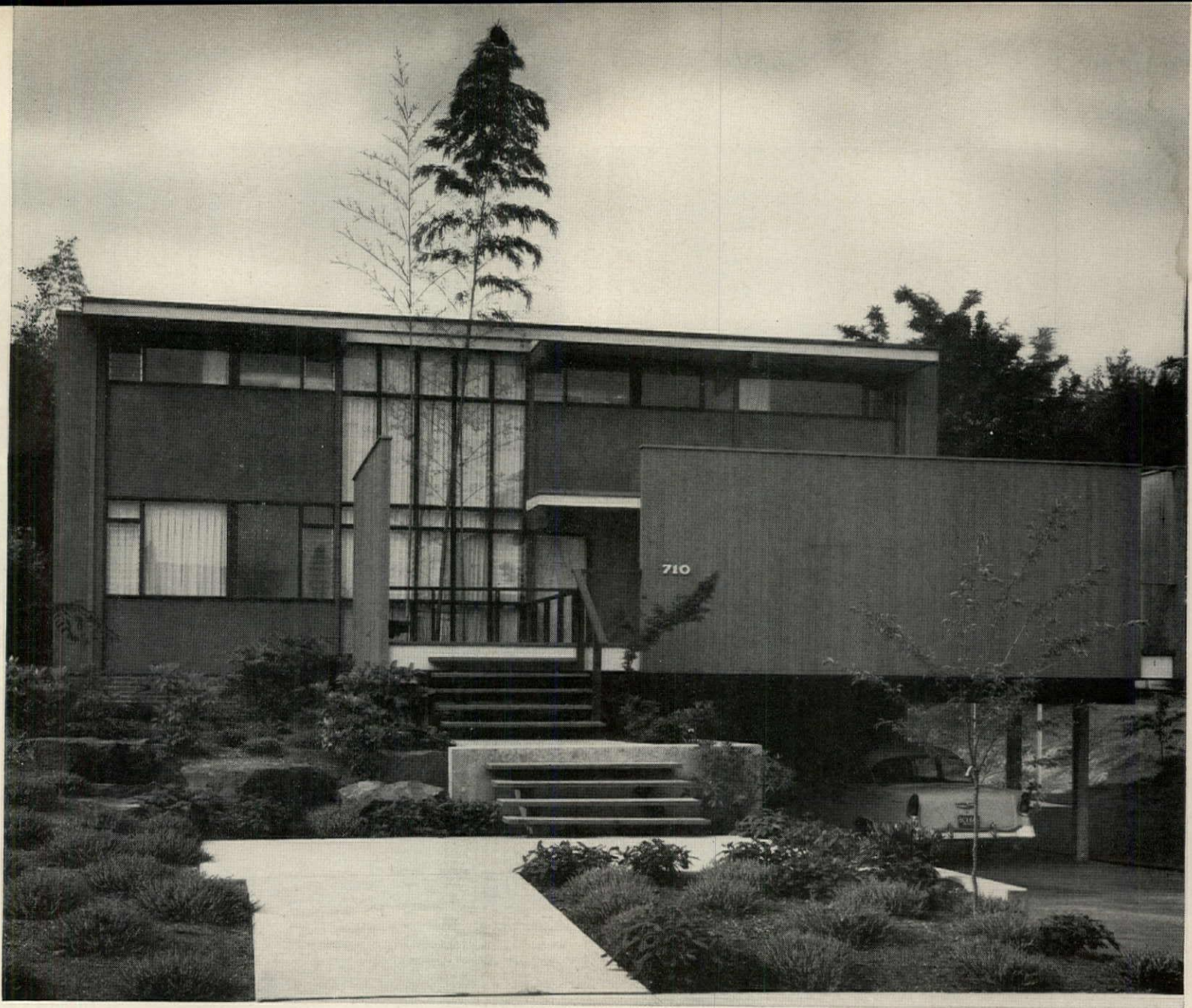
High walls of redwood screen a big front deck from street and neighbors. Carport is tucked under deck. Floor-to-roof glass lets light into interior stairway shown on p 103 .
