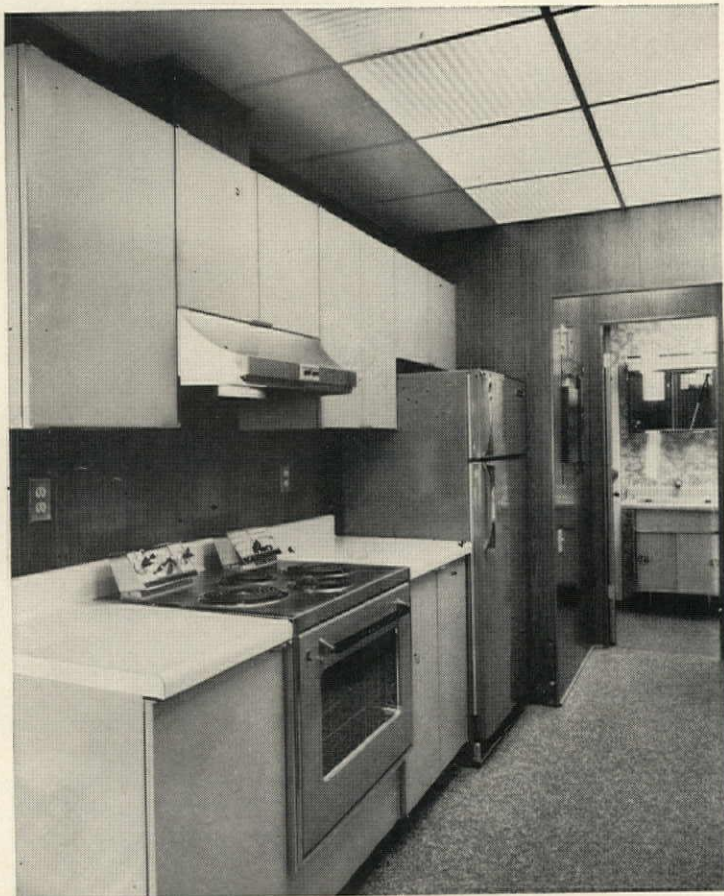
KITCHEN has luminous ceiling panels in aluminum grid. Skylights (opposite) daylight ceiling. Bathroom wall, right rear, is prefinished hardboard.
