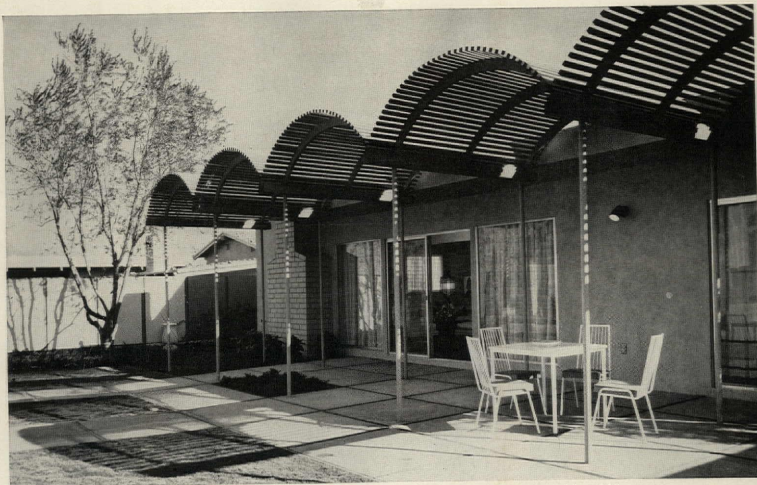
VAULTED SUNSCREENS of 2x2s nailed to built-up ribs and supported on pipe columns shelter the rear patio of this model house.
