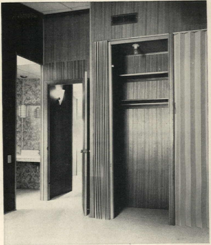
BEDROOM has prefinished paneling throughout. Master bath, left, is only 4' wide—tankless grinder toilet placed in corner makes narrow width work.
