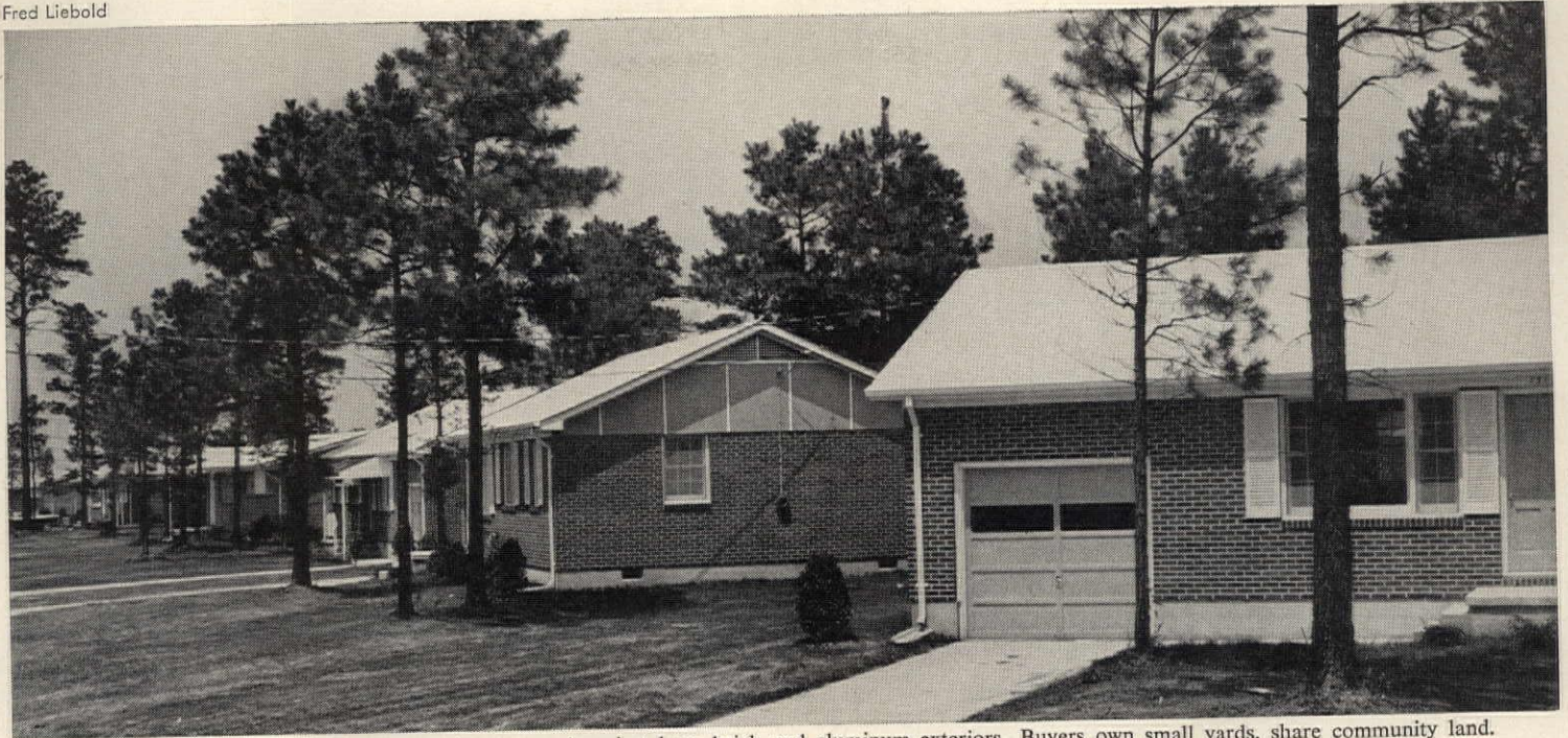
ATTACHED HOUSES in Hartshorn Homes urban-renewal project have brick and aluminum exteriors. Buyers own small yards, share community land.
