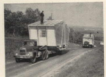
ENROUTE: Section is designed to stand road bumps on way to site.
