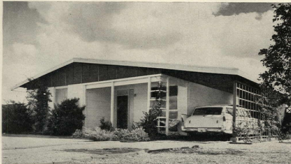
View from street shows how carport (an extra) disguises square plan, makes house look wider.
