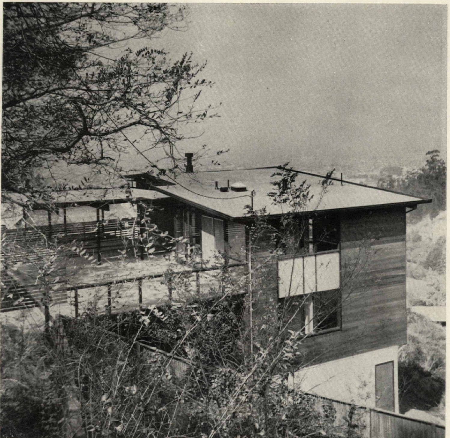
Side view shows expanse of deck connecting house to street. House is wood-framed, has redwood exterior walls, plank-and-beam ceiling.
