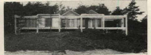
Basic frame is concrete posts and beams. House rests on piers, so it can fit any terrain.
