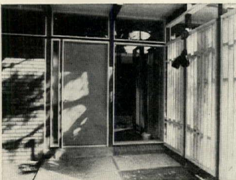
Front door is flanked by glass. Door and window frames are untrimmed pieces of clear 2x6.
