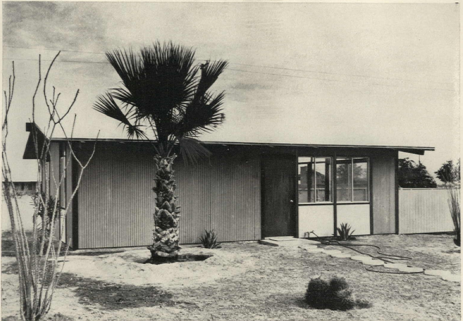
Panel joints are minimized in vertically scored plywood siding, but emphasized at windows.
