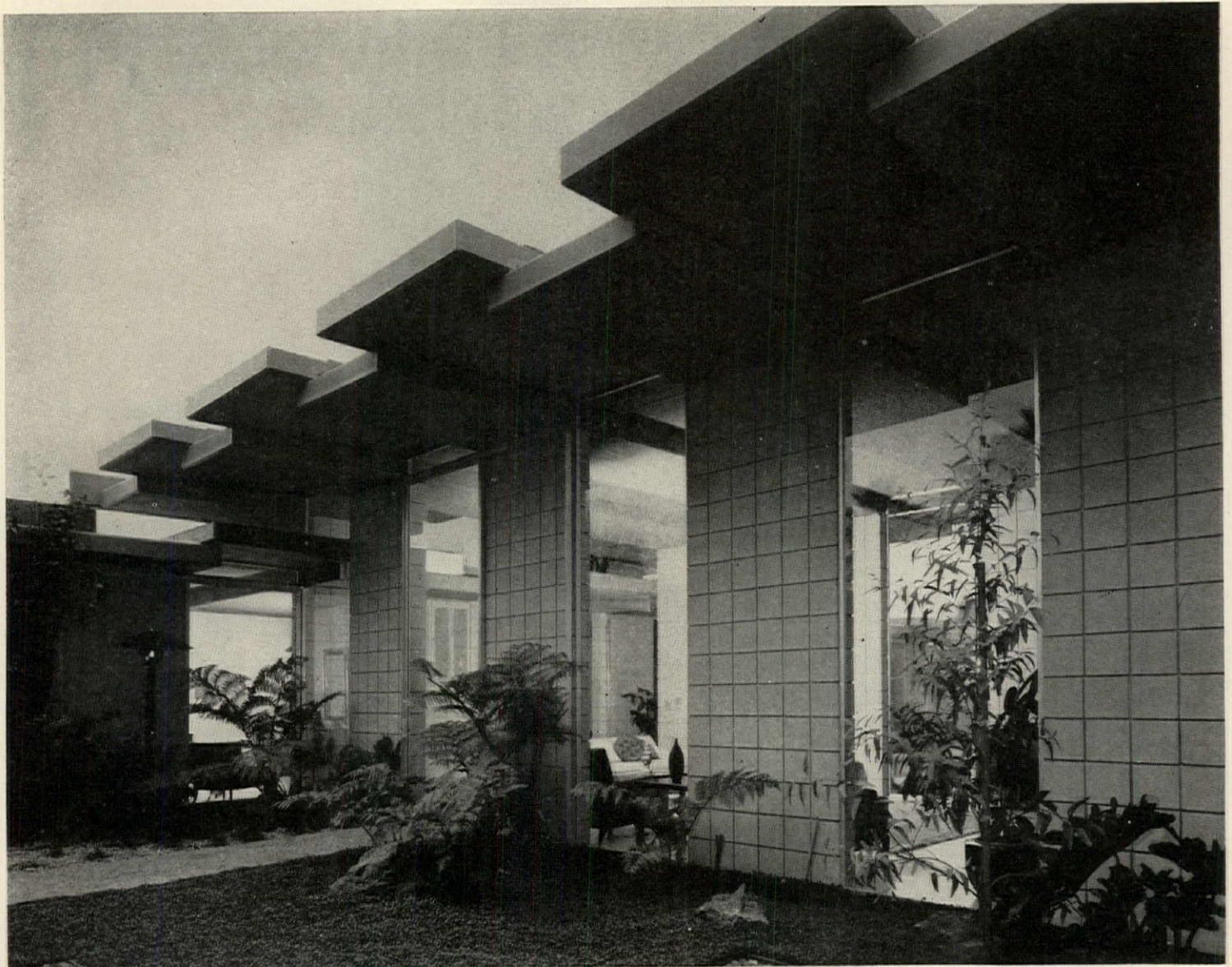
Living room wall shows basic design. Walls are 16"x8"x8" block, scored for 8"x8" pattern. Roof panels are 7½" thick to match wall pattern.
