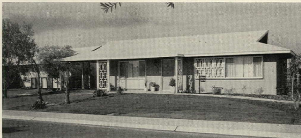
Exterior (one of four) gains interest from decorative screens and Japanese style roof.
