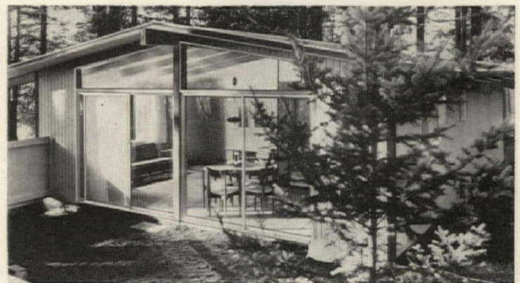
Glass gable end adds to apparent space in house by opening kitchen-dining-living area to patio. Plank-and-beam roof adds custom look at low cost.
