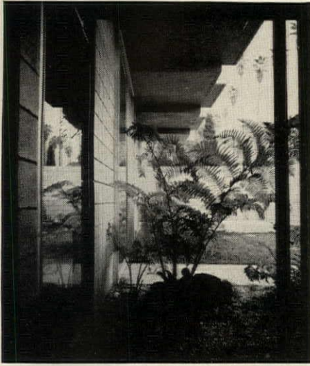
Roof panels overhang 3' and 4' to shade the floor-to-ceiling windows. This is the view across the entry garden from the master bedroom.
