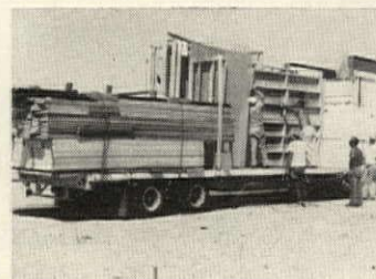
Components are trucked to site. House is assembled in two days.
