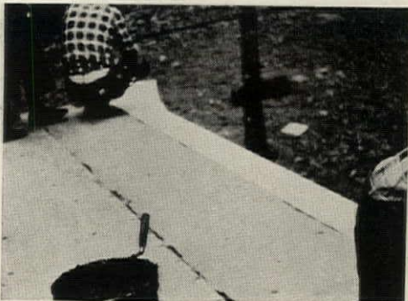
STARTER STRIP of roofing felt can be cemented down over fascia. Smooth surface resembles paint.
