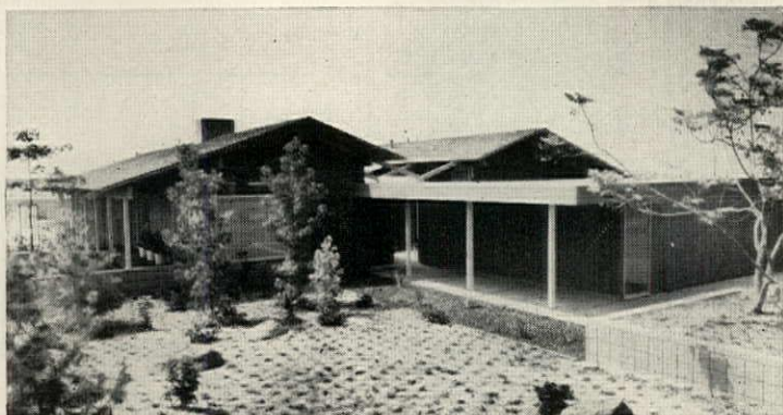
View from street shows how entry court is screened by garage. Flat garage roof extends 8' over entry walk. Vertical siding is rough-sawn redwood.
