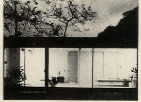
Bedroom pavilion has glass wall opening to brick-paved terrace. Carport is behind camera.
