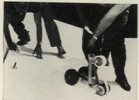
PLASTIC FILM TAPE with pressure-sensitive adhesive coating is applied to side and end laps.
