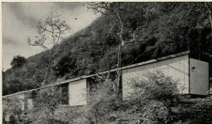
On street side, clean lines of house are emphasized by the continuous fascia and the bright colors used: Panels are light blue; trim is olive drab.
