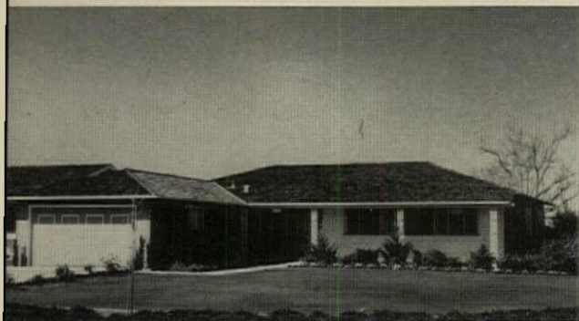
MODEL COST CUTTER 1: Rather than build a new model, Mackay Homes sometimes gives an old model a new look. The model above was revamped, see right, by changing the porch columns, the fenestration, the wainscoat treatment, the garage doors, and the landscaping.
