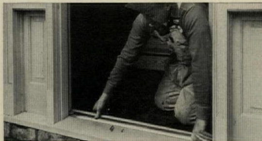
6. Stainless steel threshold lasts longer. This stainless steel threshold will keep its just-new appearance for years. 100% self-sealing to keep out drafts, rain, snow and insects, it installs quickly, needs no special caulking, and costs no more than others less durable and less efficient.
