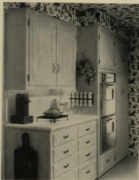
KITCHEN CABINETS , built on job, are pine. Counters are ceramic tile in diagonal pattern.
