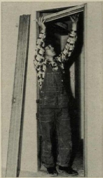
4. Steel door frames adjust and align themselves. Save up to 20% in installation time with these steel doorways. They go in plumb and square because they are self-aligning and self-adjusting. No mortising, no sanding, no hardware preparation.
