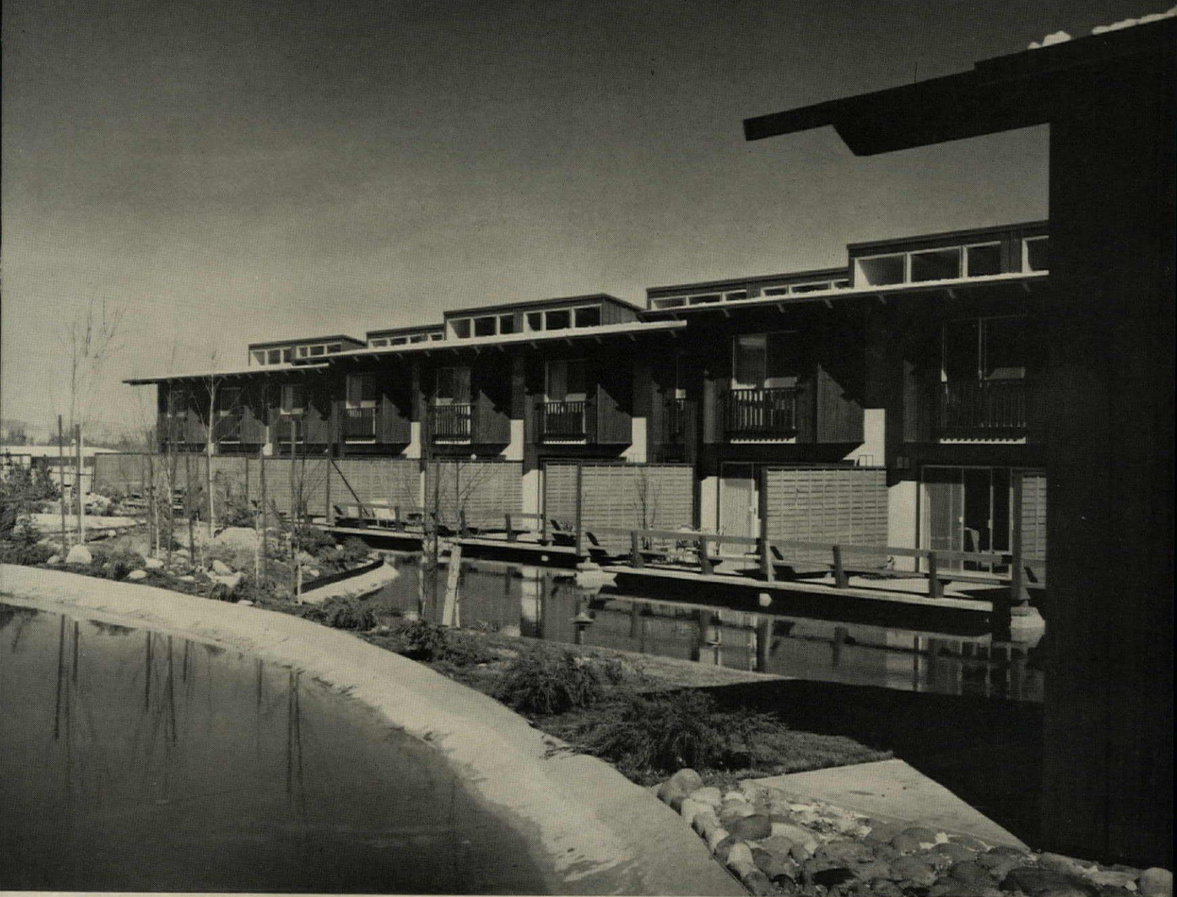
Patios off rear living rooms face central lagoon. Wood siding and fencing are cedar. One-bedroom units are at left, two-bedroom units at right.
