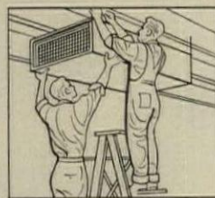
Central-Air Unit ceiling mounts in basement; supplies base heat load, cooling, electrostatic filtering, humidification and deodorizing.
