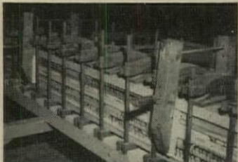
BEAMS of pine boards are laid up with waterproof glue in press.
