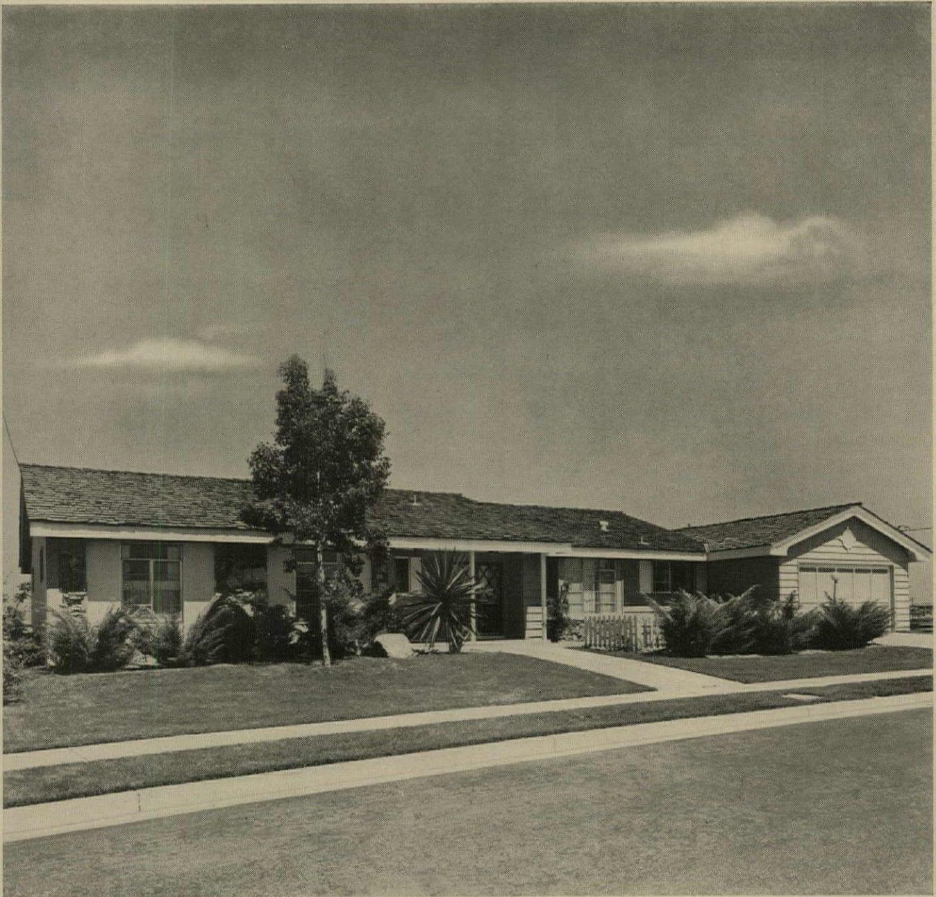
The living room of this six-room rancher is 30' x 16' and it has ash paneling plus a brick fireplace and hearth. Among the home's many other features is the Bell System's Home Interphone which lets the family talk room-to-room and answer the door—by telephone!
