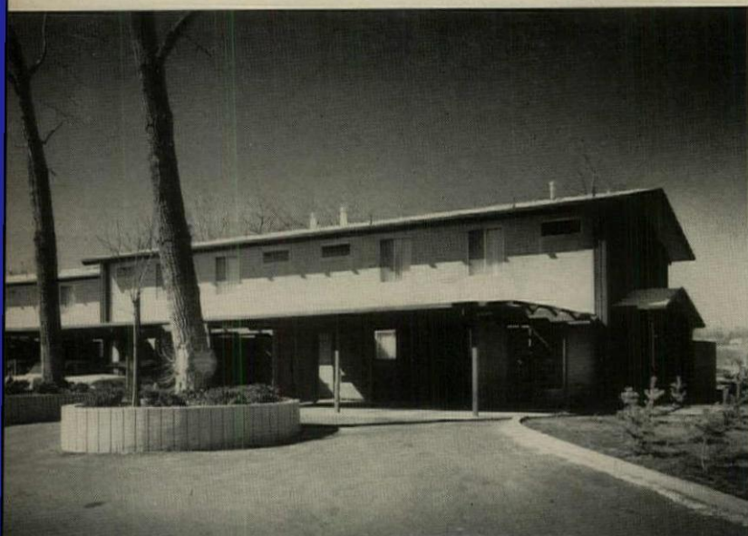
Entrance side of Virginia Lakehill has carports which also shelter the front doors. Light wall covering is exterior plaster in pastel colors.
