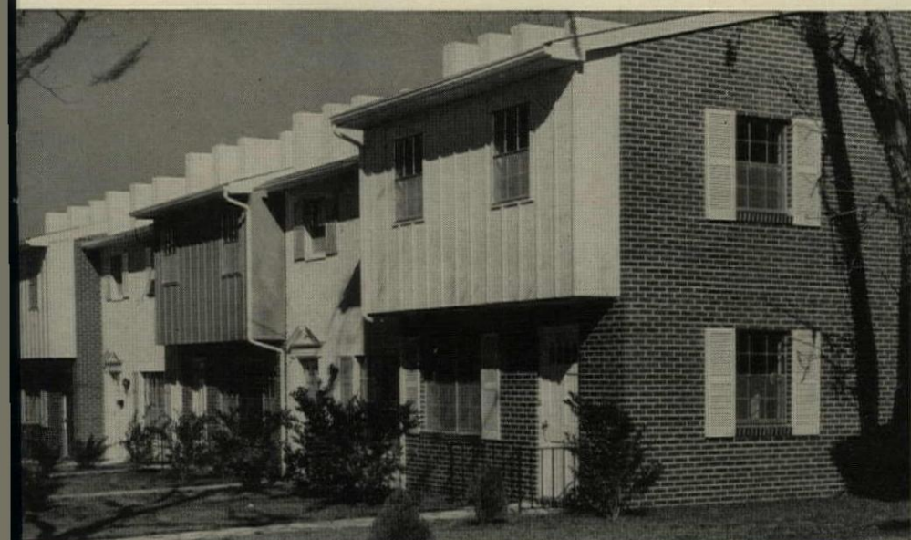
Hercules liked the ease of transporting panels to the second floor of their handsome Town House project.
