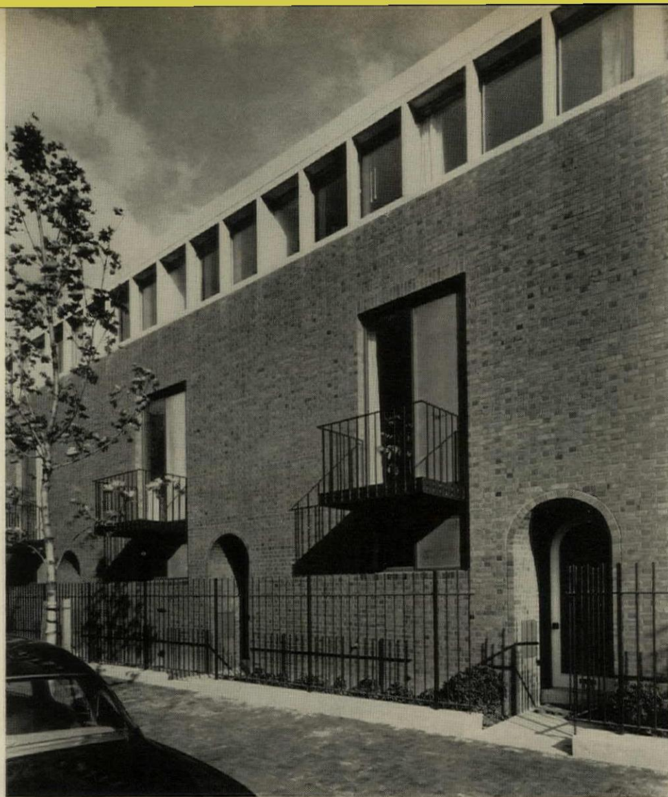
Spirit of old townhouses is caught by brick, iron railings, and arched doorways. Brick sidewalk is in Philadelphia tradition.
