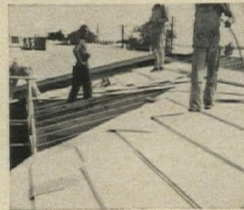
LOW MAINTENANCE HOUSE , one of FHA Sec. 233's first-completed projects, was built by Dallas Builders Fox & Jacobs. The house is expected to need no exterior painting for 15 to 20 years, has an easily washed interior paint surface, experimental film-coated siding and trim, plastic waste and vent lines, and a film-surfaced plywood roof system (right). Estimated extra cost: only 2%.
