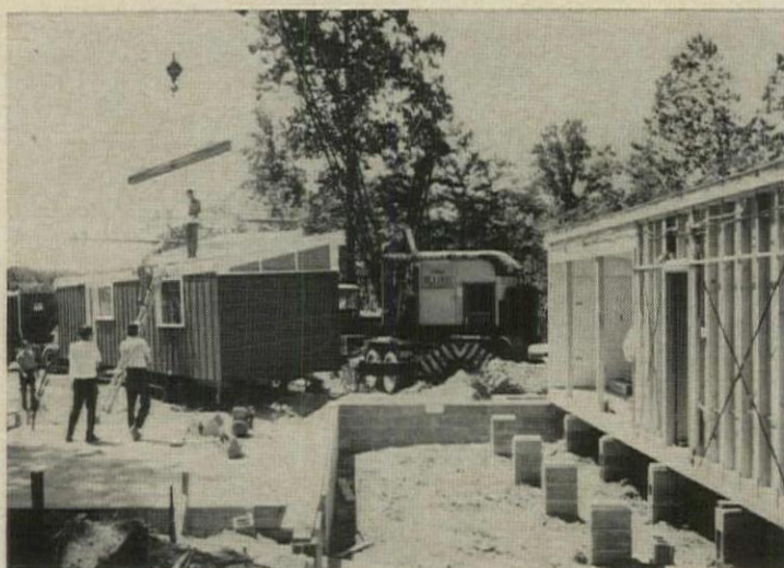
SIDE SECTIONS , completely finished in the plant, flank a panelized, drop-in center section in this pilot house by innovator Carl Boester. This idea solves the problem of over-the-road loads wider than 10' (which are prohibited in many states). Side sections are 10' wide; center section is 4' wide.
