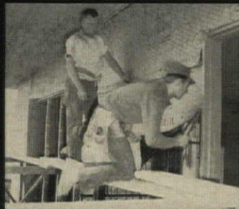
Portland Cement is sprayed on.
