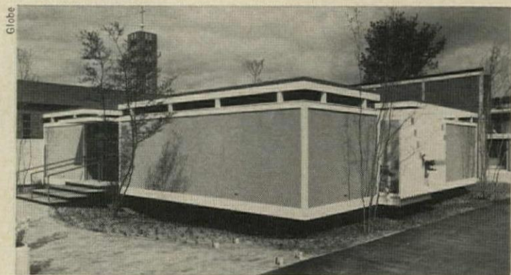
SELF-CONTAINED MODULES in house designed by Architect Robert Engelbrecht for U.S. Plywood at the Seattle World's Fair (H&H, June '62) can be set in line, around a court, or in any other arrangement for a wide variety of floor plans.
