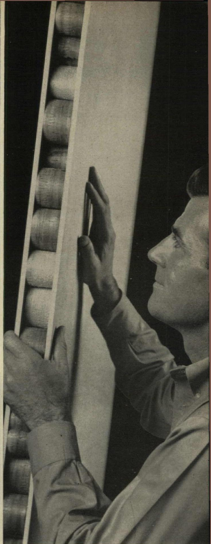
Large 4' x 8' panels go up quickly and easily, with less nailing and fastening, and reduced erection time.
