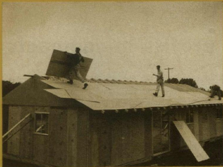
6. As soon as roof sheathing is on, the house is enclosed and doors can be hung. Interior work—which uses as many prefabricated parts and materials as possible—can start any time. It's 1:30.
