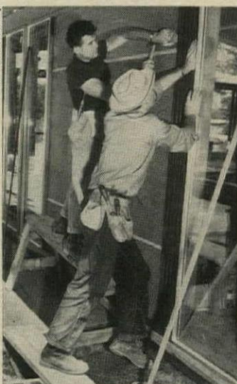
ALCOA CAREFREE HOUSE , designed by Architect Charles Goodman, demonstrated use of prefinished aluminum siding.
