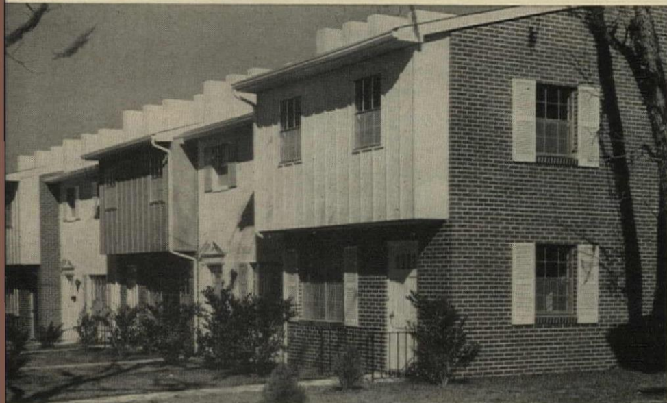
Hercules liked the ease of transporting panels to the second floor of their handsome Town House project.
