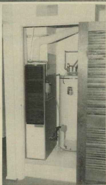
Right: The 12-inch wide, 570 Series conditioner is installed in a central utility closet directly over the return air plenum.
