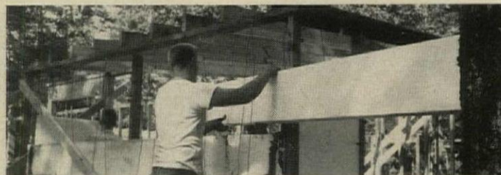
FOAMS began making news as soon as Dow Chemical brought its polystyrene plank on the market. Now taken for granted as foundation insulation, the plank can be used as a plaster base or as the core of sandwich panels. It paved the way for all the foams that are following it.
