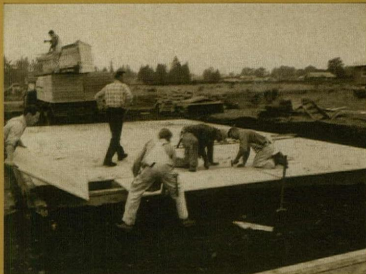
2. The rest of the parts come just as the floor is completed. Buying is simplified because plywood sheathing, wall panels, flooring, trusses and even interior partitions all come from the same supplier.
