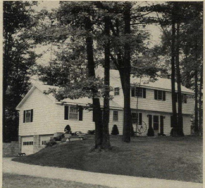
Clifton Knolls, Schenectady, N.Y. In the midst of a severe cold climate, these total-electric homes are kept warm with General Electric baseboard electric heat. Builder R. Van Patten says "... my buyers love it." 130 Gold Medallion homes are already sold; and another 500 are planned.
