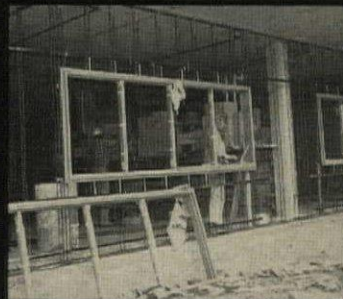
Then Keymesh Paperbacked lath is applied.
