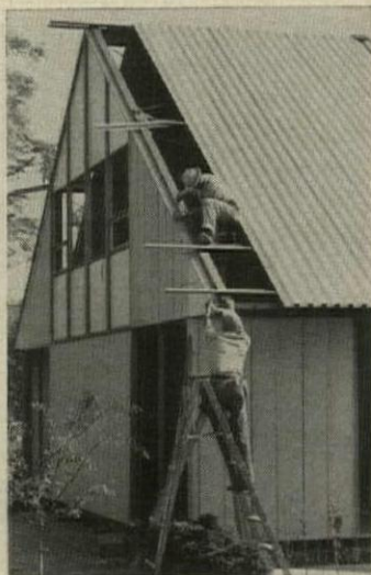
FERRO HOUSE was designed around the long-life qualities of porcelain-enamelled steel. Material was used for both roof and siding.
