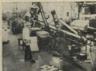
TRUSS MACHINE at Inland Homes positions and drives plates on both sides of truss. Time per truss: 2½ man-minutes.
