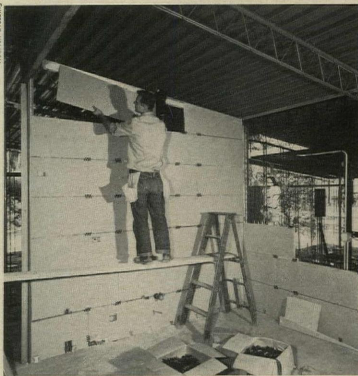
SCPI BRICK HOUSE showed the feasibility of building with prefabricated brick panel sections over a steel frame.
