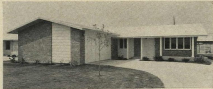
LOW MAINTENANCE HOUSE , one of FHA Sec. 233's first-completed projects, was built by Dallas Builders Fox & Jacobs. The house is expected to need no exterior painting for 15 to 20 years, has an easily washed interior paint surface, experimental film-coated siding and trim, plastic waste and vent lines, and a film-surfaced plywood roof system (right). Estimated extra cost: only 2%.
