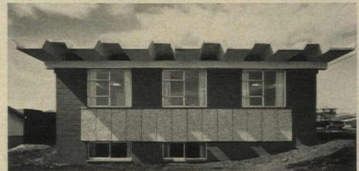
CAST CONCRETE in roof shapes can take on almost as many unusual forms as sprayed concrete. Architect Robert Des Lauriers used four hyperbolic paraboloids for the roof of the San Diego house shown at the top; Walter Weber of Colorado Springs precast trough shapes for the roof above.
