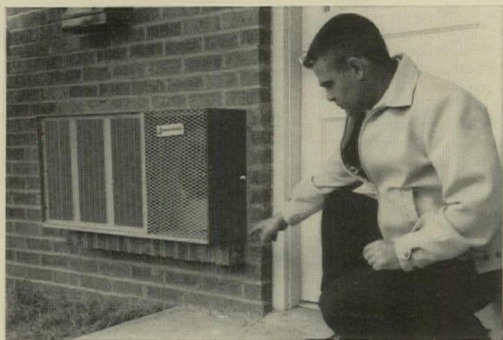
Below: The through-wall condensing unit is flush with the inside wall, yet has only a slight exterior projection.
