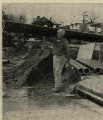
Lightweight sewer pipe has ribs and skins of ABS plastic with perlite filler, is tough, durable and flexible. Joints are chemically welded in 60 seconds, can be buried immediately. Ten-foot lengths can be handled by one man, require 60% fewer joints than conventional pipe. Kyova Pipe, Irontown, Ohio. (For details, check No. 24 on p. 176)
