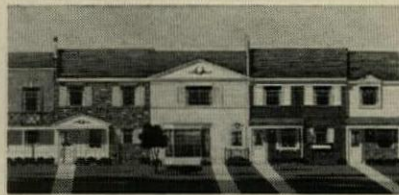
Fleetwood’s new Williamsburg Square features Chrysler Airtemp 1253 snap-in units with resistance heat. Installer: Climate Control, Inc., Phoenix, Arizona.
