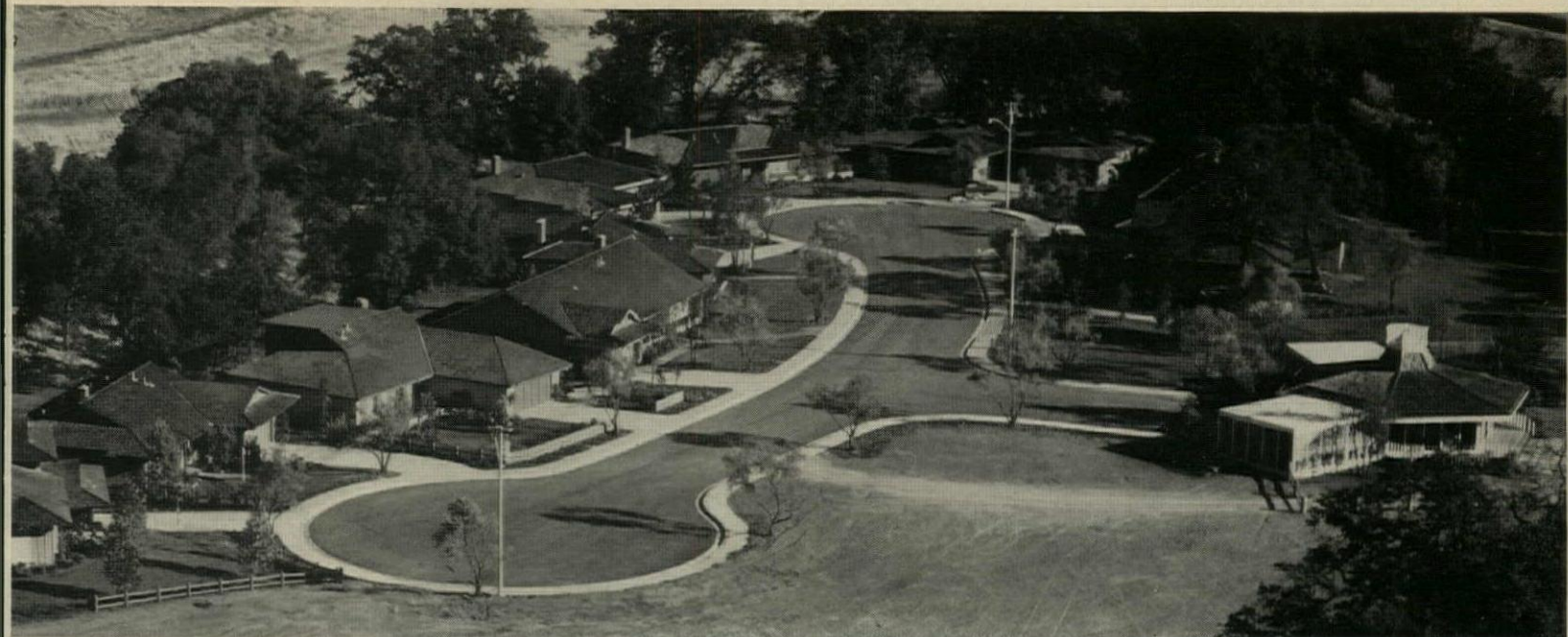
City of Sunset, Sacramento, California , being built by the Sunset International Petroleum Corporation on the famous 12,000-acre Spring Valley Ranch, will include 400 Medallion homes, recreational activities, community facilities and an industrial park—a complete new city.
