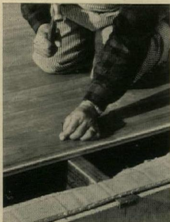
SPIRAL-SHANK NAILS 2" long are driven through flooring directly into the steel beam.
