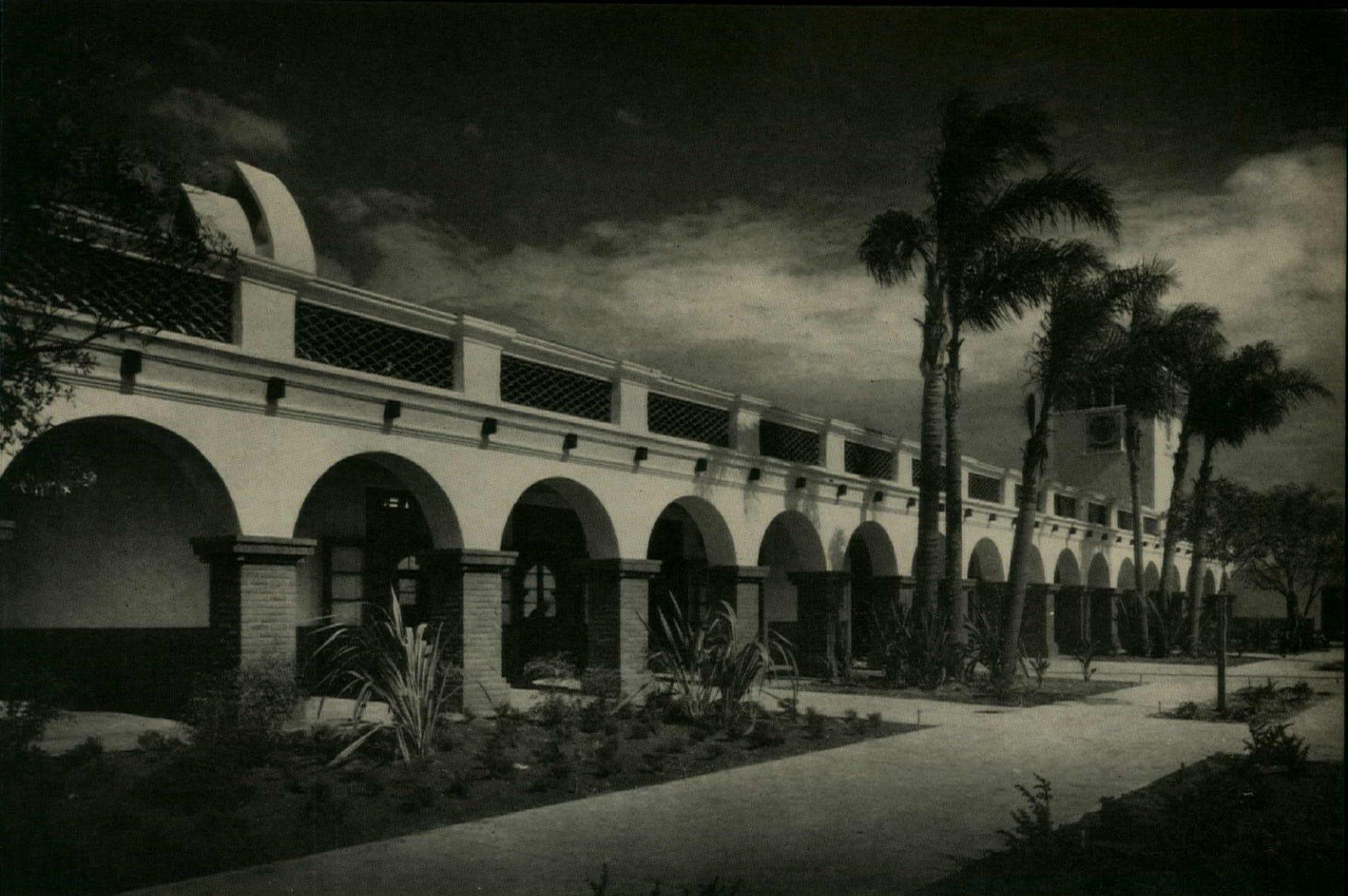
$850,000 CLUBHOUSE was completed before Ross Cortese opened the gates to prospects in his latest Rossmoor Leisure World in Laguna Hills, Calif.
