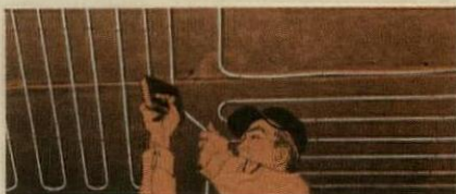
Ceiling Cable , imbedded in plaster or drywall, is totally silent, completely clean, fully automatic with individual room controls. Easily installed.
