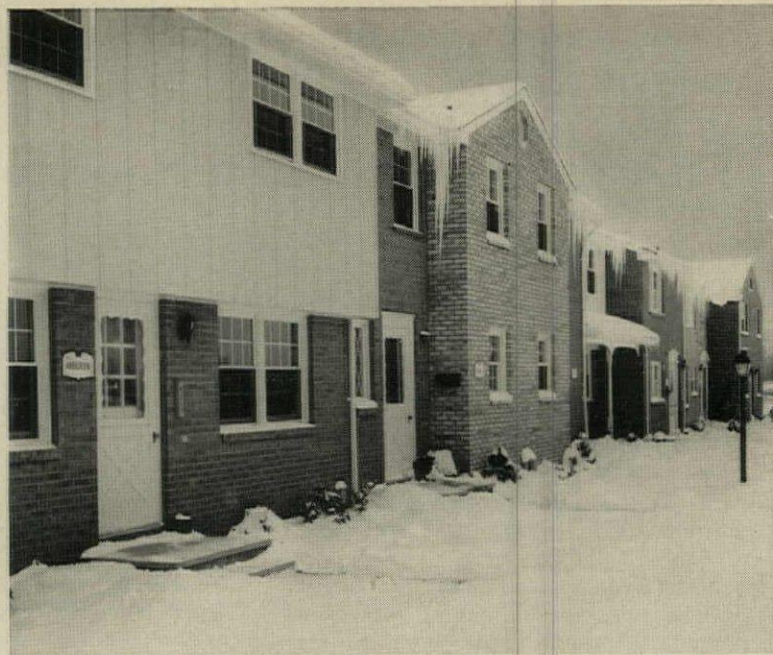
Belmont Village, Syracuse (Liverpool), New York, will offer 616 Gold Medallion townhouses featuring electric resistance heating and General Electric appliances. Builder John L. (Roy) Bellinger, president of Bellinger Construction Company, finds customer reaction to total-electric living to be a "big plus" in his sales program.
