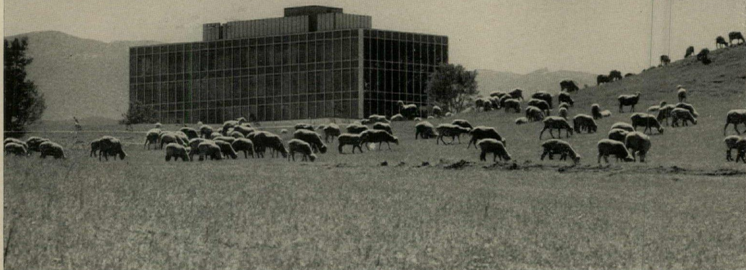
$5 MILLION DEFENSE PLANT , amidst grazing sheep, occupies 100-acre site in a 1,000-acre industrial park at Rancho Conejo northwest of Los Angeles.
