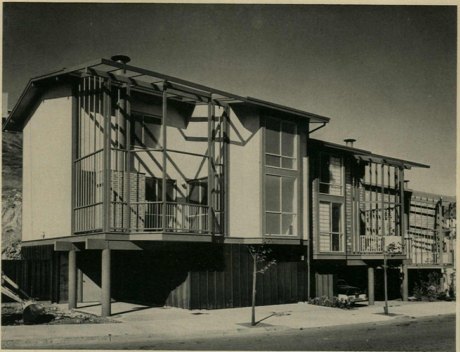
THREE-STORY HOUSES on steep lots are kept shallow (32') to minimize excavation of the rocky hillside. Two car garages are beneath.
