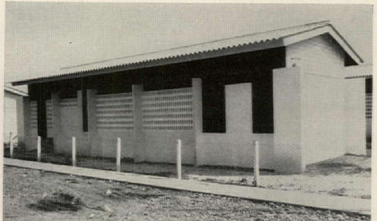
LOCAL MATERIALS , except for some plumbing fittings, make up the house. A ventilated cavity between the roof and ceiling helps keep houses cool.
