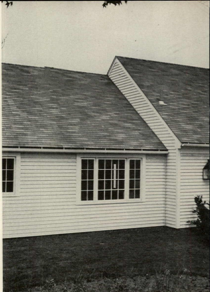
COLONIAL EXTERIOR , finished with solid vinyl siding and random-design asphalt shingles, is typical blend of the old and new.
