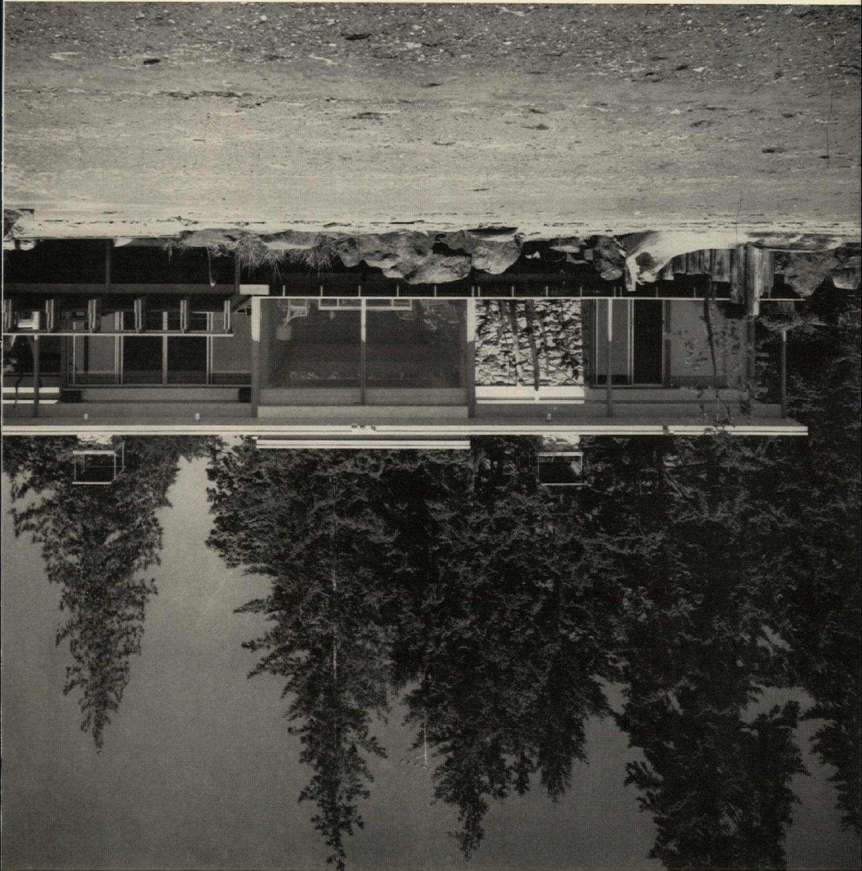
Beach-front house with a glass wall facing the water won an Honor Award. Designed for year-round use, it is raised above possible high tides on 3½"-thick concrete pilings. (For plan and photos, see p. 78; for details, see p. 84.)
