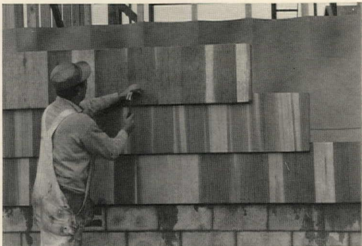
Eight-foot shake panels can save up to 70% of installation time compared to regular shakes. E-Z-Ply has outer layer of unstained or gray primed cedar shakes, cross-bind center layer and undercourse layer. Shaker Town, Cleveland. (For details check No. 13 on p. 147)
