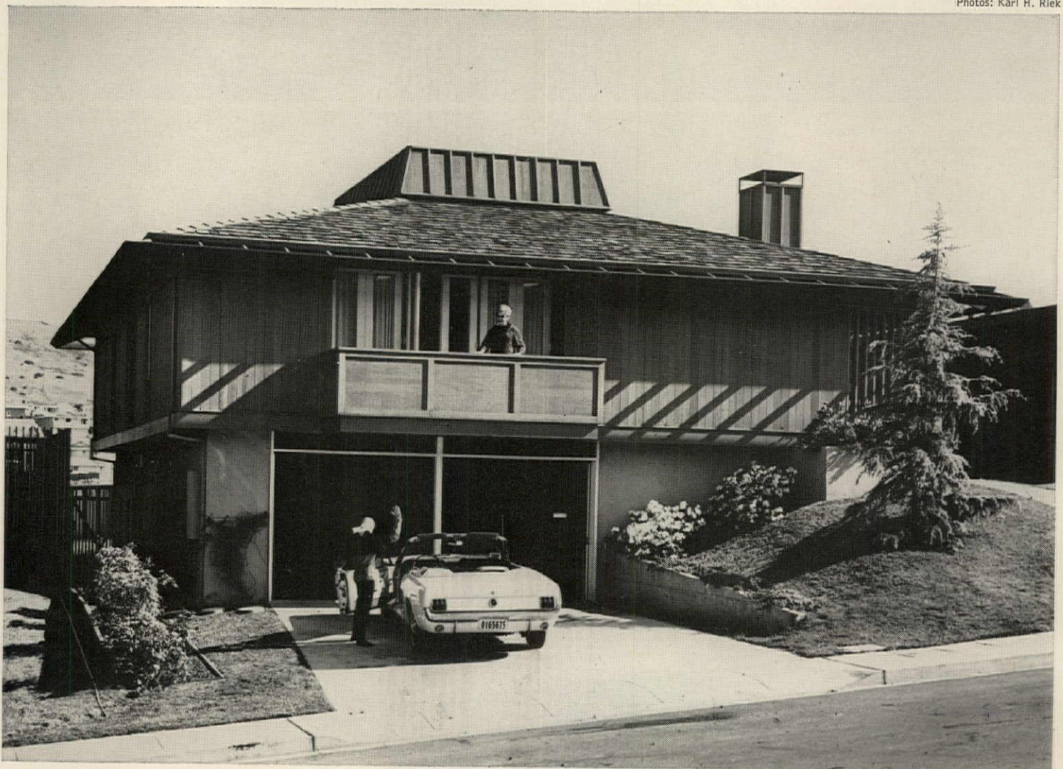
Roof pyramid is capped by a monitor that hides a skylight, plumbing vents and flues. Gray finish is used on exterior.
