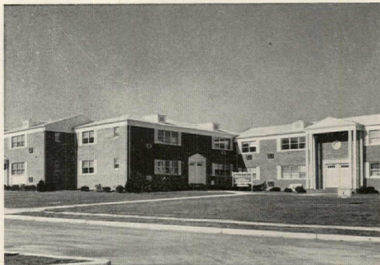
Aberdeen East, Matawan, New Jersey , is an attractive community of 240 Gold Medallion Garden Apartments being built by Arthur Goldberg and Paul Waters of Parr Associates, Inc. The sales appeal of these total-electric apartments is enhanced by the modern General Electric lighting and underground power system.
