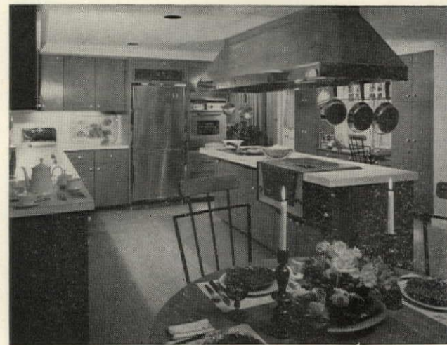
CEILING-HUNG HOOD vents island cooking center's drop-in range and barbecue. Lights are recessed in the ceiling and under cabinets.
