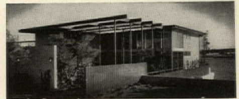
Severe lines of the house and its fencing are softened by a wooden trellis over the garden-entry court. All rooms are oriented either to a view of the bay or inward to the court.
