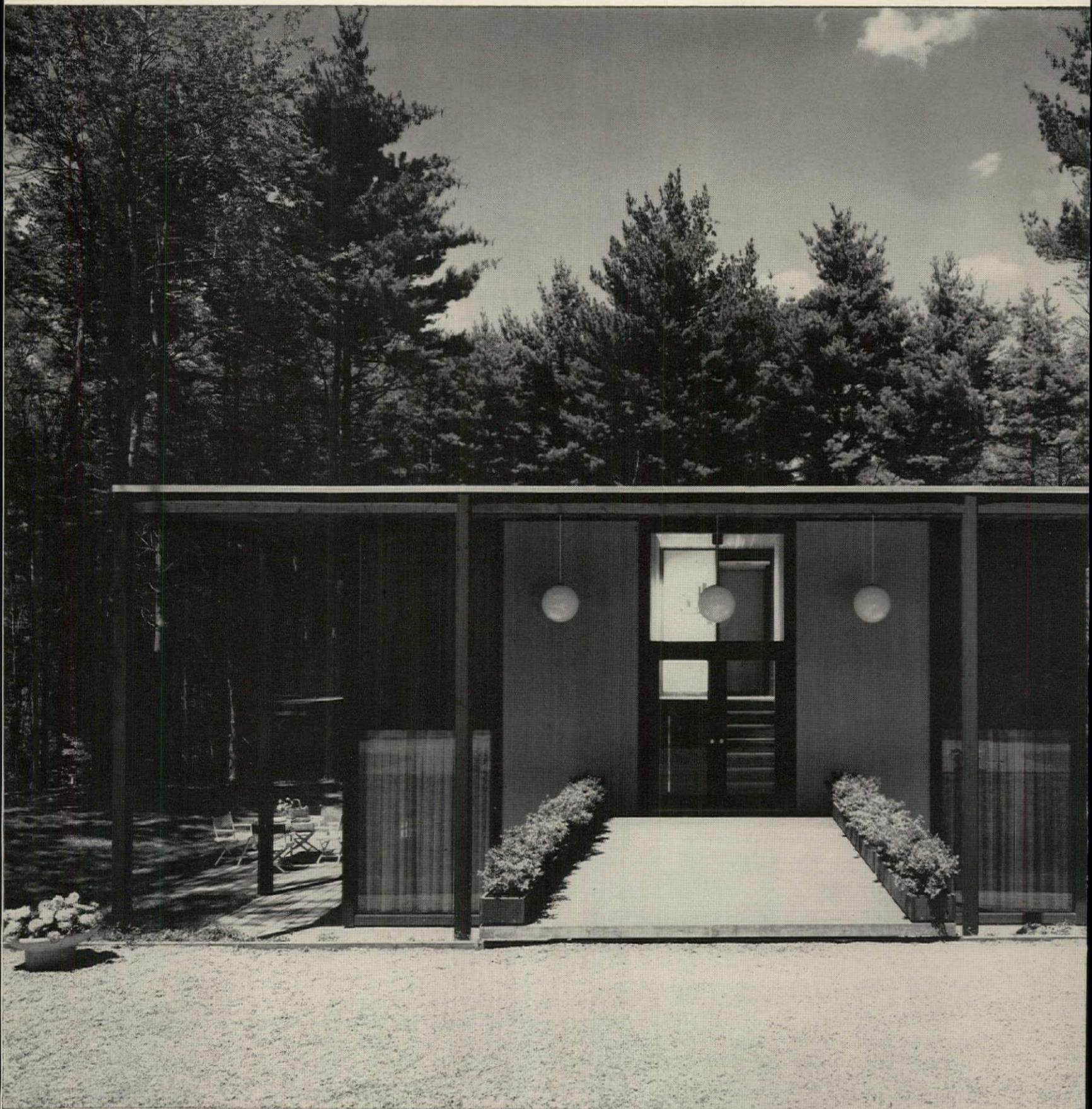
Classic simplicity of this post-and-beam house by Architects John Black Lee and Harrison DeSilver proves that the difficult split entry can be handsome in appearance, workable in plan.
