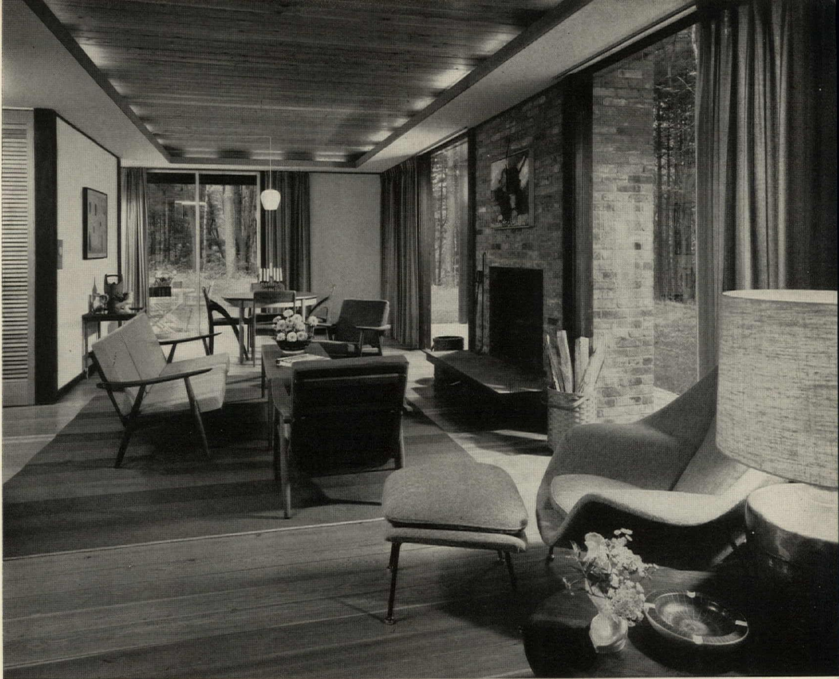
Sweeping expanse of living-dining area (31') opens to terraces on two sides. Ceiling is underside of 2½" wood decking.
