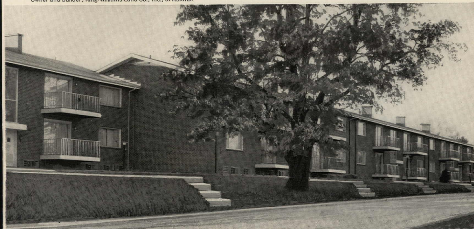
Warren Park Apartments , Baltimore, Maryland. Five buildings, with a total of 200 apartments, are air conditioned by York Flex-O-Metic systems, including Borg-Warner furnaces. Owner, Warren Park Associates; Builder, Gorn Bros., Inc.; Architect, Morris Steinhorn, A.I.A.
