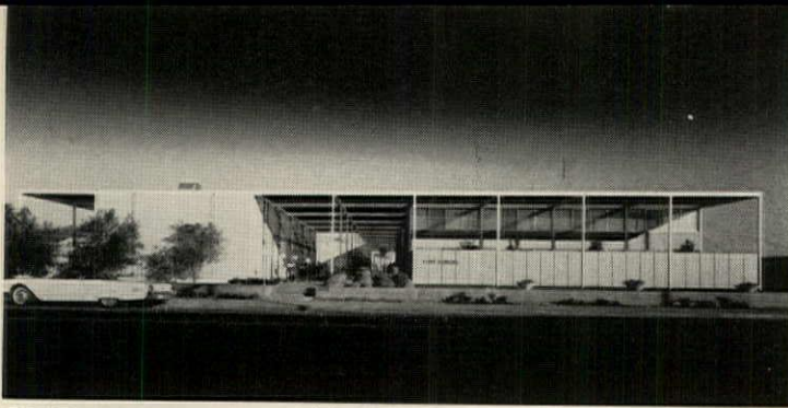
FIRST 22 UNITS are grouped in sections of five and four. Each apartment has two floors, 1,024 sq. ft. of space and 1½ parking spaces in rear.
