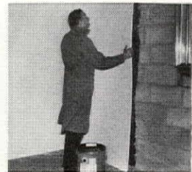
Bonding polystyrene foams — does not collapse foam.
