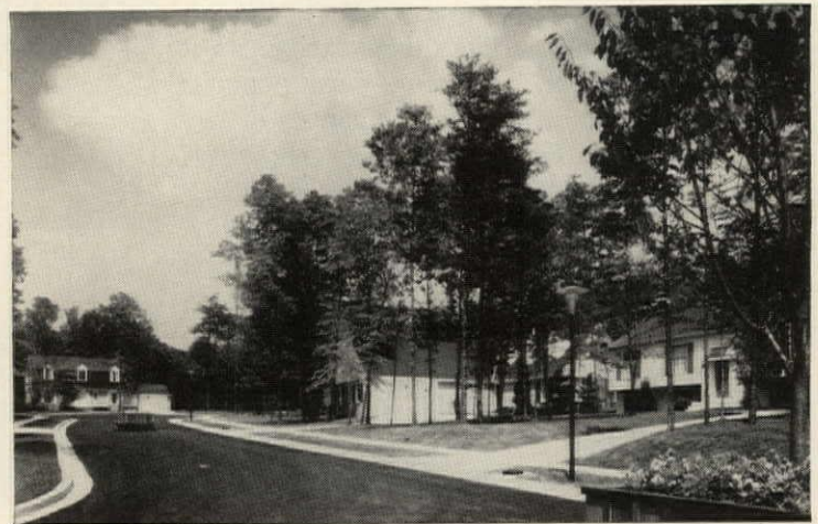
MODEL-HOUSE AREA (upper left in plan) is typical of wooded neighborhoods at Crofton.
