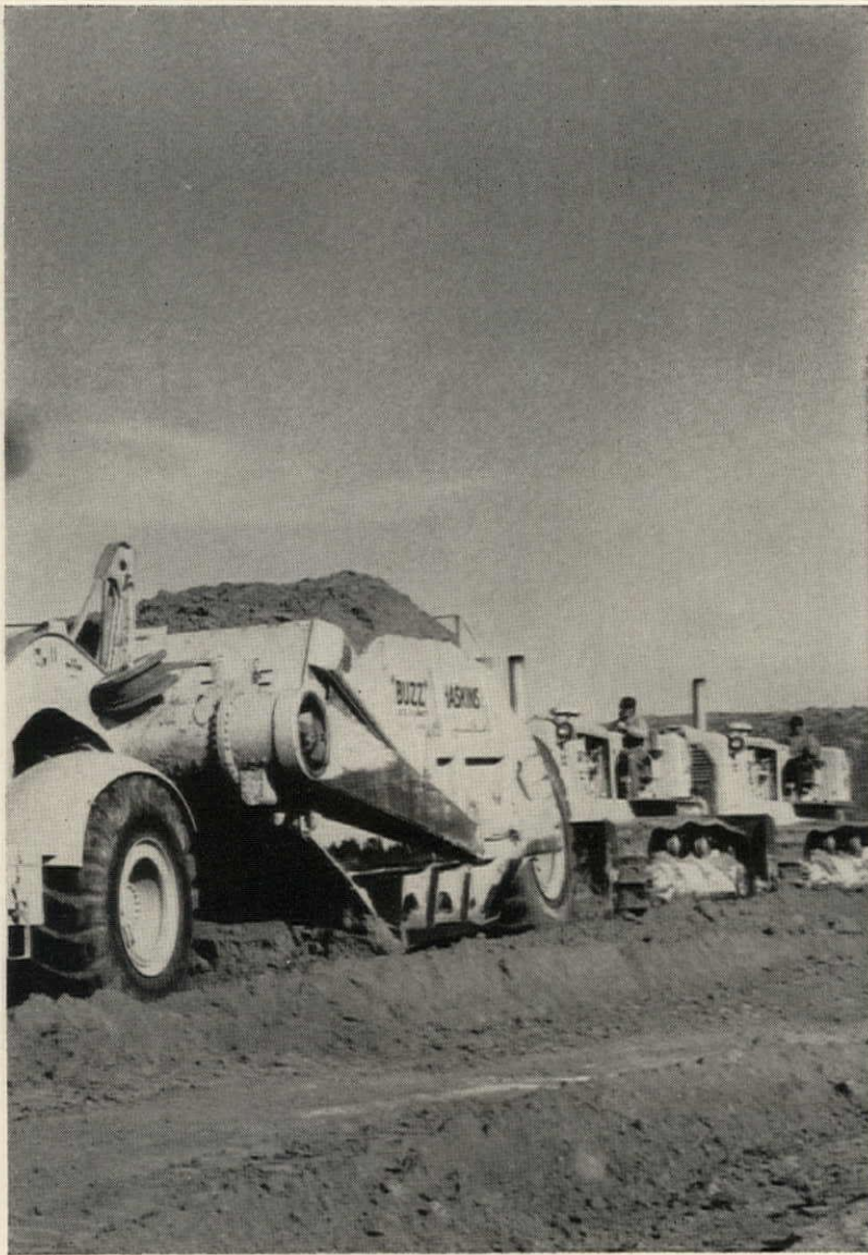
DOUBLE-PUSHING 40-yard scrapers with two 32-ton tractors gets loads out of cuts fast.
