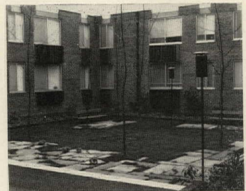
16. Lights in grass court are black cans set on poles and topped with car hubcaps.
