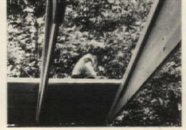
plate. Workmen butt next post-truss against panel girts, nail, add two panels and another post-truss.
