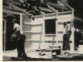
with gable-end truss and corner panels. Overlapping plywood is nailed to posts, floor beams, sill
