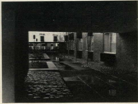
5. Court area is blacktopped, with grass plots, left, delineated by raised concrete curbs.
