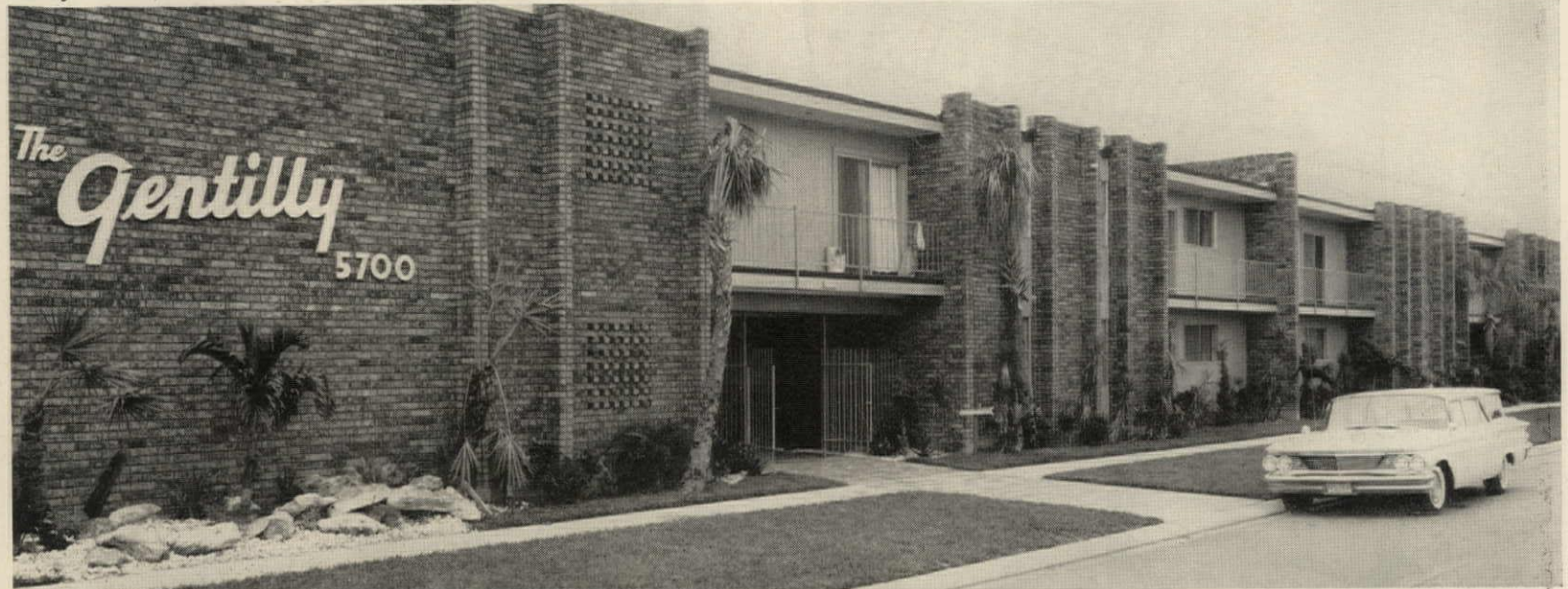
Gently Apartments, New Orleans, Louisiana , where results were so successful that owner David Craig is planning another Medallion project. The 65 Gold Medallion units are built with courtyards, one with swimming pool. Individual metering permits separate tenant billing.
