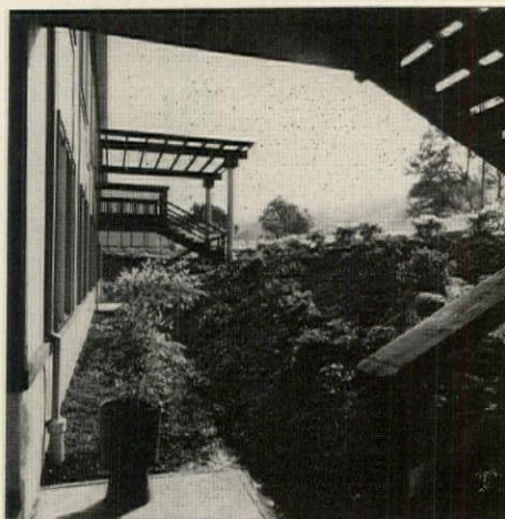
STAIRS to second and third-floor apartments are shortened by bringing grade above first floor.
