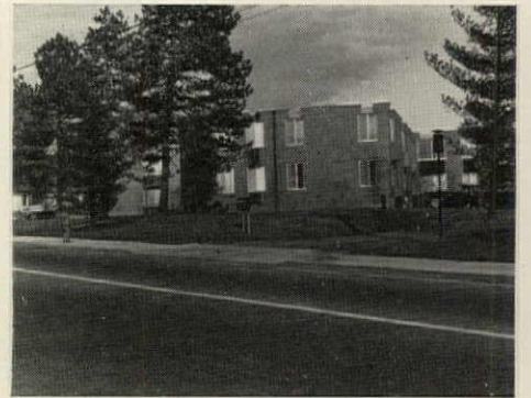
1. Street facade is on the angled end of the narrow site. Frontage is only 285'.
