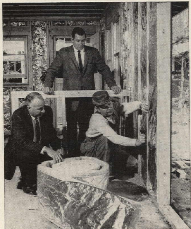
PROPER INSULATION builds in economy and comfort. Here Hobart Smith and construction manager Rousseau check on the installation of full-thick batts in outside walls.
