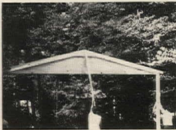
INTERLOCKING FRAME of trusses in slotted posts ( above ) tilts up. Erection ( below ) starts
