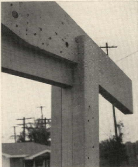
INTERLOCKING FRAME of trusses in slotted posts ( above ) tilts up. Erection ( below ) starts
