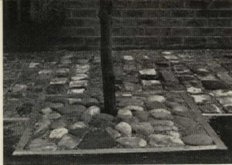
9. Belgian blocks, behind tree, are hard to walk on, keep passers-by away from apartment windows.
