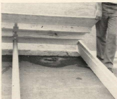
INTERLOCKING FLOOR has panels of 5/8" plywood nailed to notched 2x4 purlins. Beams, 2x10s
