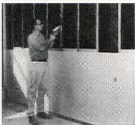
Stud adhesive — bonds to wood and metal.
