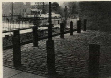
11. Wooden bollards, made of sawn-up telephone poles, are used to outline court areas.
