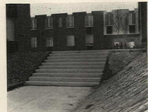
17. Sloping areas are paved with Belgian block, right, or covered with wood-chip mulch, left.
