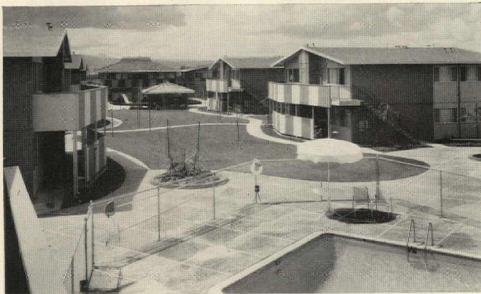
CENTER GREEN includes swimming pool, in foreground, and laundry, in small hip-roofed building at far end. If the project were converted to
