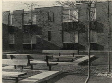
6. Wooden benches are set into the concrete borders of small grassy areas.
