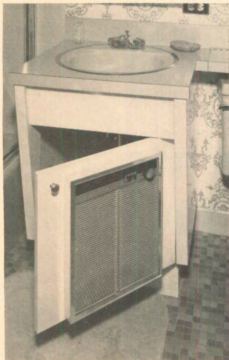
COMPACT HEATING UNIT fits into vanity front and is shallow enough so storage space inside vanity need not be sacrificed.
