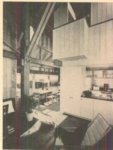
KITCHEN BLOCK open toward dining area, supports bathroom, balcony, storage area above.
