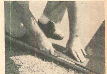
4. Metal spacers leave 1/16" contraction joint between tiles.
