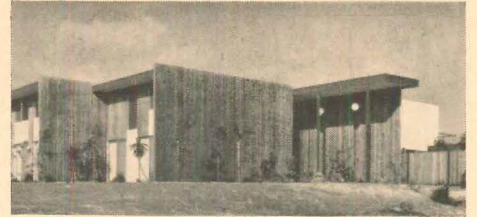
RECESSED WALLS of these units near the formal entrance provide protection from sun.
