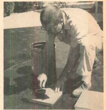
2. Adhesive is applied to back of tile with a 3" trim roller.
