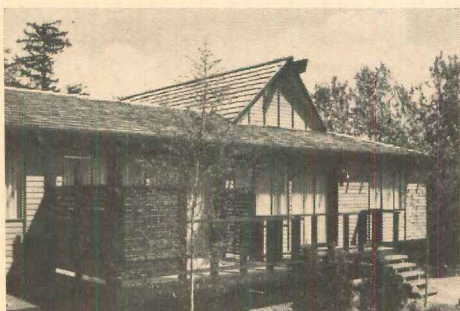
REAR DECK , shared by two units, is divided and screened for privacy by redwood fencing.
