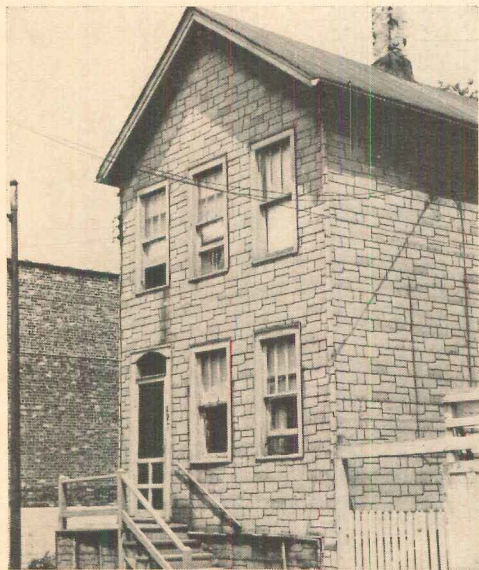
CHICAGO FRAME HOUSE , a higher-cost custom job, was jacked down 3' and heavily altered. Remodeler: Old Town Contractors Inc. For Old Town's production methods, turn to page 92.
