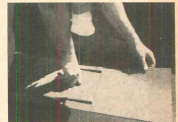
6. Excess tile at edges can be cut with sharp linoleum knife.
