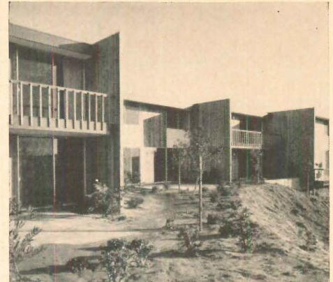
PROJECTING WALLS between units increase privacy of outdoor living on two levels.
