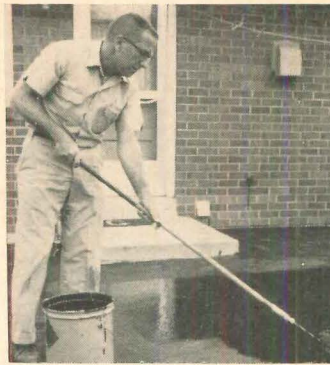
1. Neoprene adhesive is roller-applied over neoprene primer.
