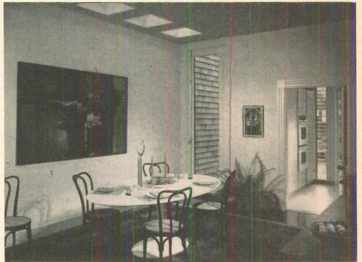
SERIES OF SKYLIGHTS admit daylight to dining room from upper-level light well.
