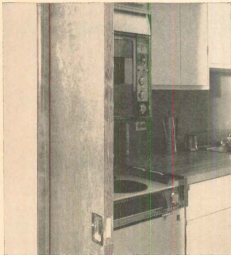
POCKET DOOR —a natural space-saver—is planned into virtually every job, particularly in tight kitchens that open off narrow halls.
