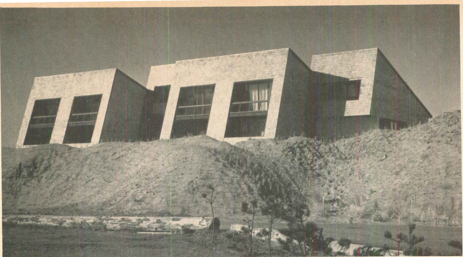
LAND SIDE OF PROJECT features sheltered balconies, cut out of the steeply sloping shingled roofs, which provide protection from the wind.
