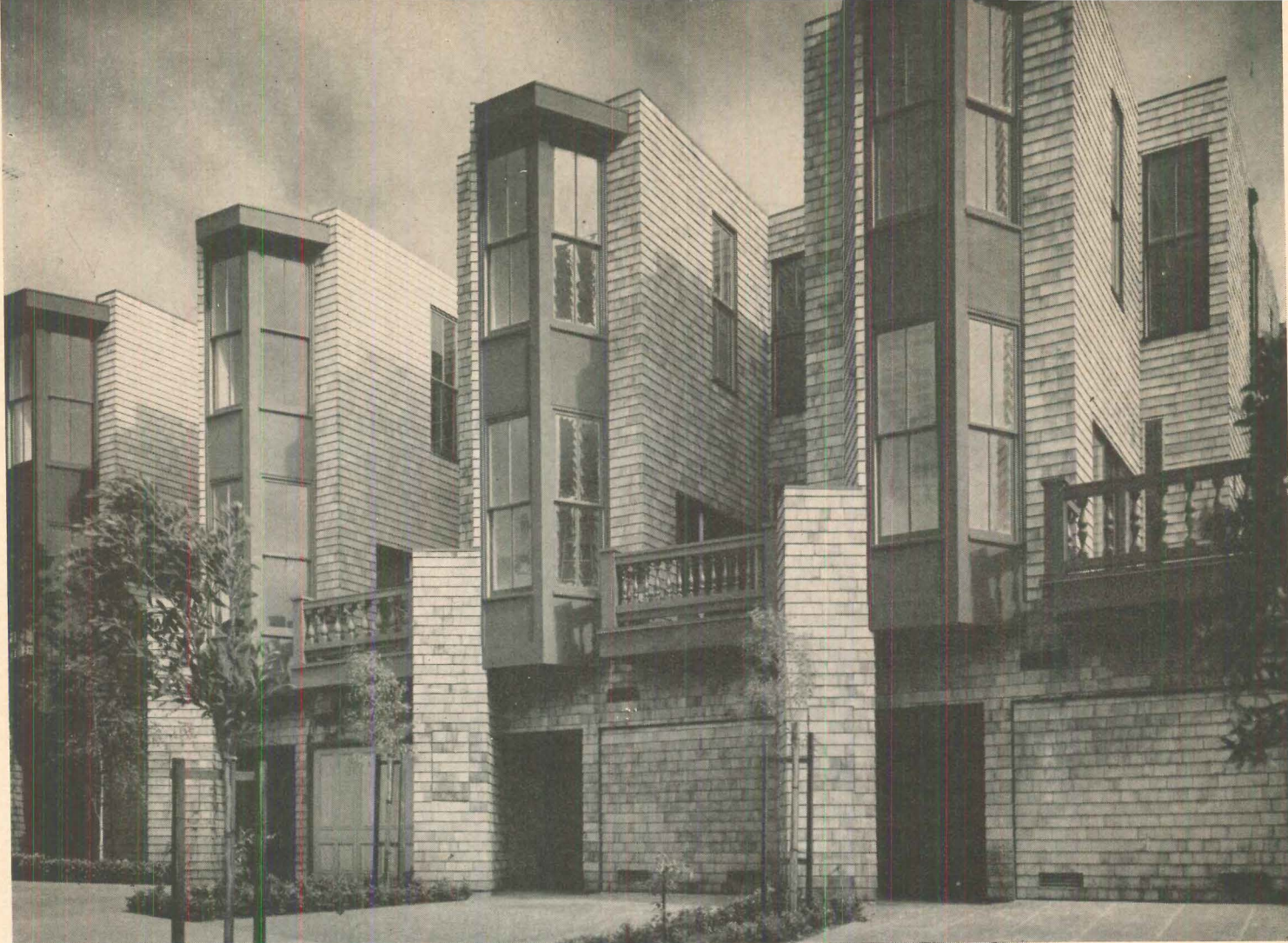
REGIONAL FLAVOR of San Francisco in 1890s is carried out by shingled facades, tall windows, old-style porch railings, paneled or shingled garage doors.
