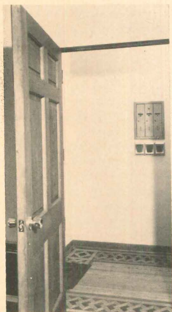
JOB-LAMINATED DOOR FACING of birch or walnut plywood converts one side of raised-panel door to flush style, so same door blends with both restored floor and stairs in public hall and modern apartment interior.
