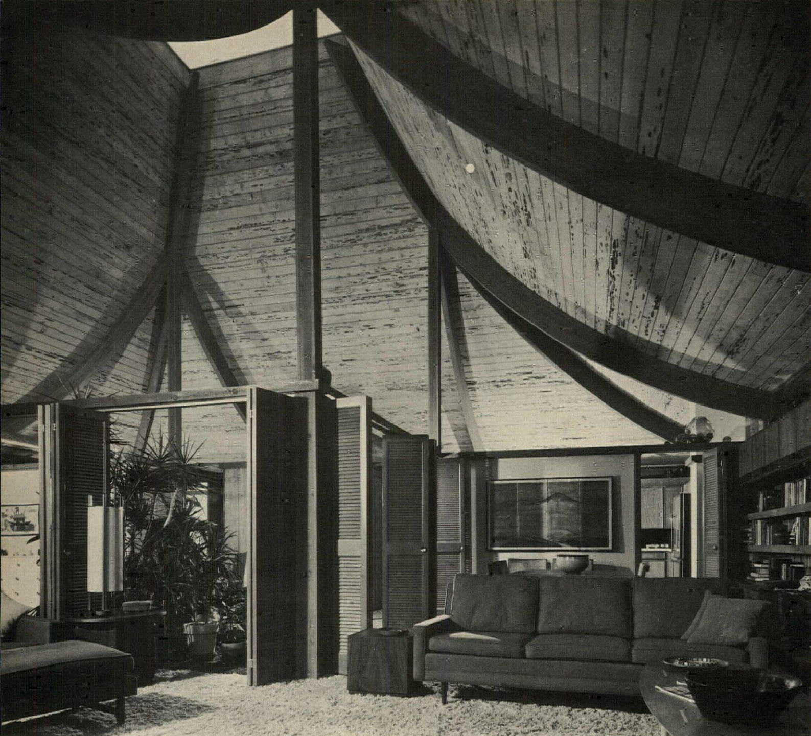
VAULTED ROOF over main living area (view 1 in plan) is framed with curved glue-lam beams, planked with pecky cedar. Skylight is 25' above floor.
