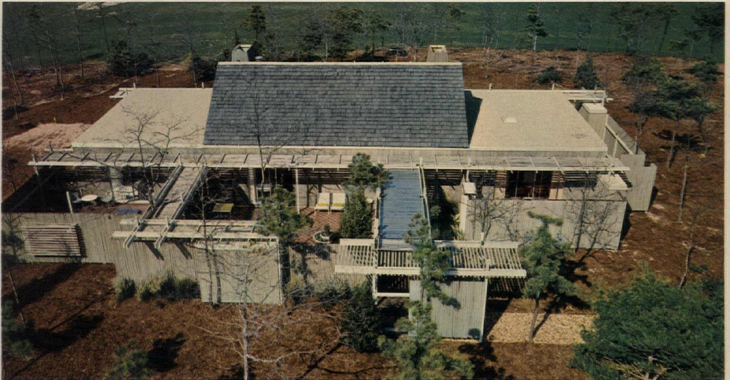
AERIAL VIEW of front (2) shows relation of terraces to the basic house. Entrance is under trellis in foreground, service yard at far right.
