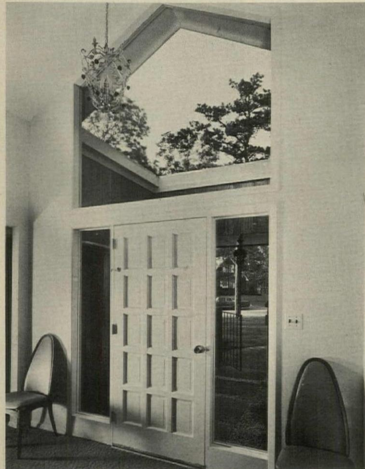
FOYER (2) gets daylight through glass gable end and glass panels flanking door to entry court.
