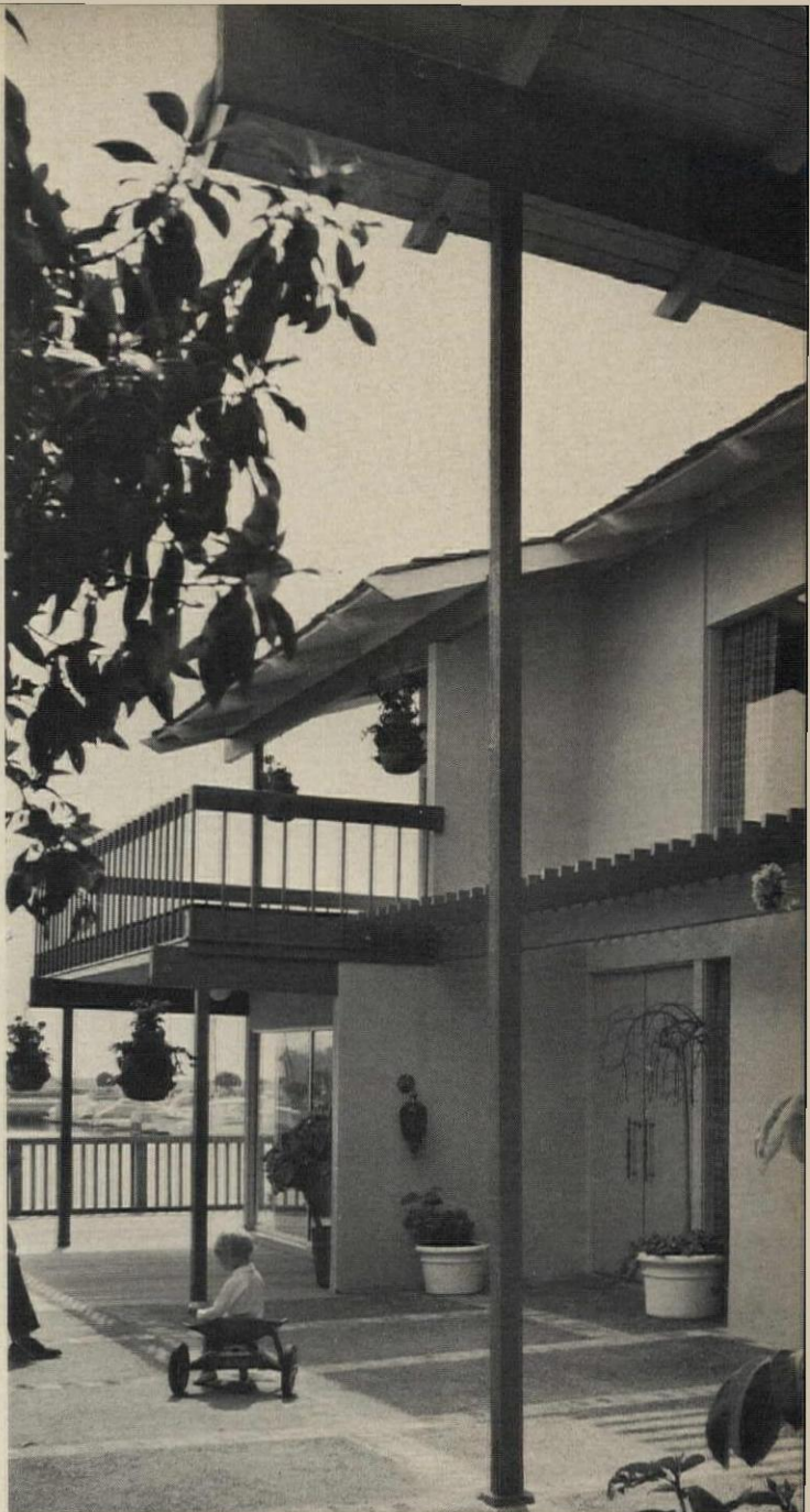
ENTRY COURT (3) leads to inset front door at right. Upper deck opens off master bedroom.
