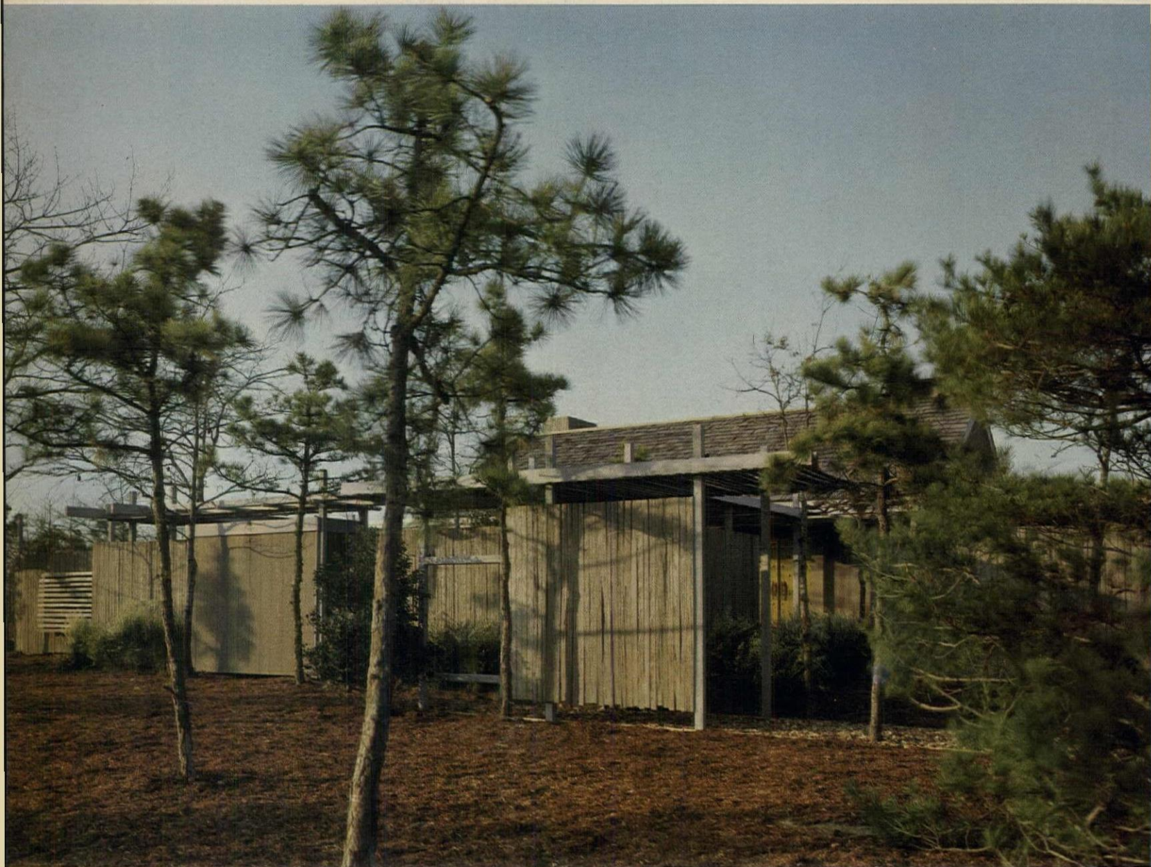
STREET VIEW ( 1 in plan, p. 65 ) shows only fences and gable roof. Fencing is not standardized; buyer gets a package of stakes, plans his own terraces.
