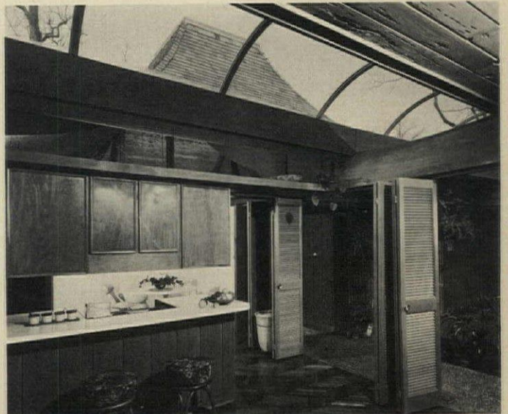
STRIP-PLASTIC SKYLIGHT (4) bridges gap between main house, left, and garage wing, right.
