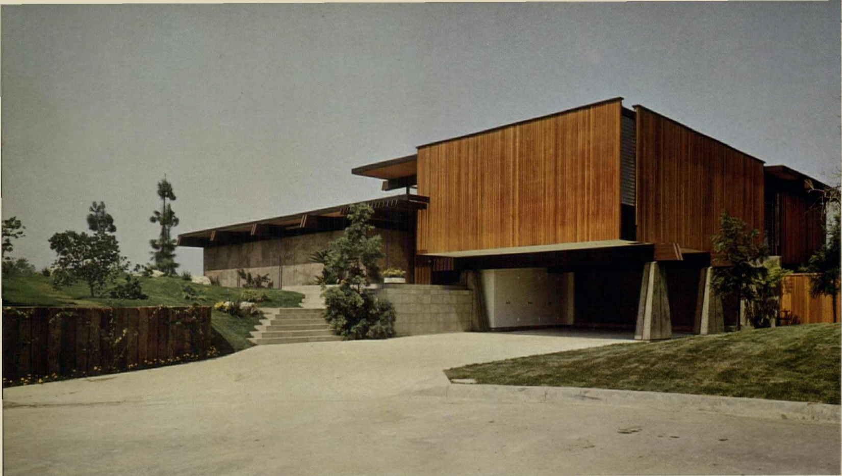
WINDOWLESS FACADE (view 1 in plan) faces street for privacy. Bedroom wing over carport is supported by glue-lam beams on concrete piers.
