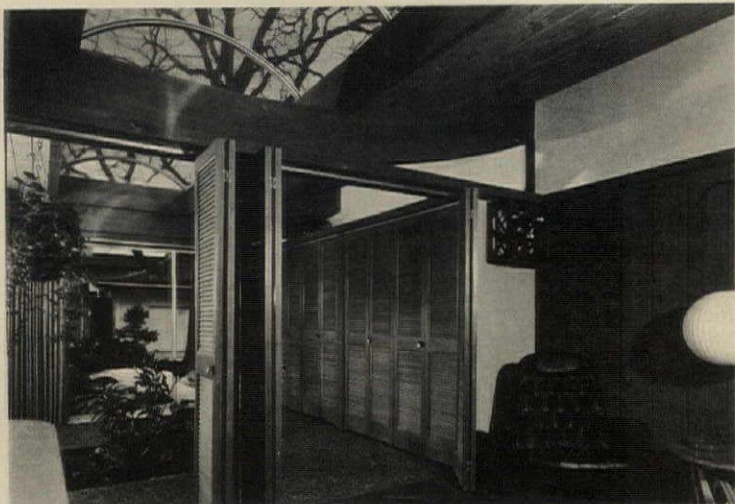
ENTRY (5) , beyond folded doors, has terrazzo floor with planting area in center.
