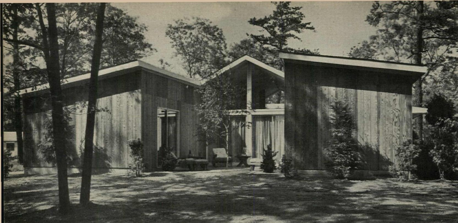
REAR ELEVATION (view 1 in plan) shows shed roofs over wings, gable roof over center living room. Siding is stained vertical boards.
