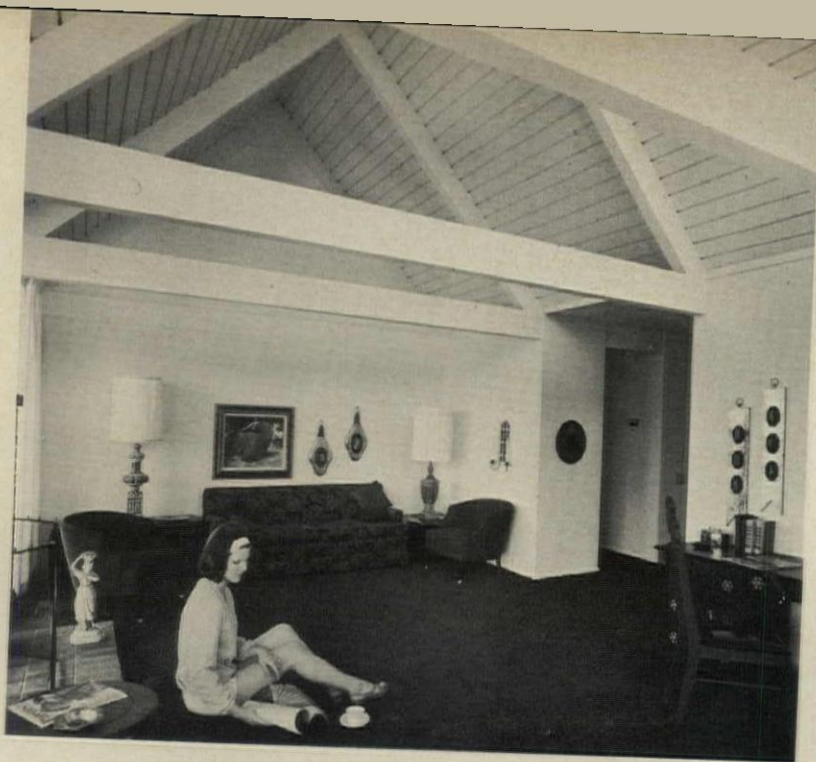
PEAKED CEILING (3) with heavy rafters and collar beams gives living room a spacious feeling.
