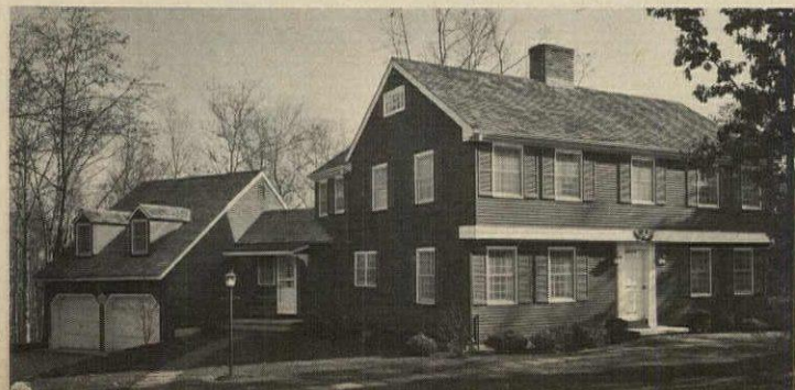
GARRISON MODEL gets bigger second floor from overhang. Note 4" exposure of clapboards.
