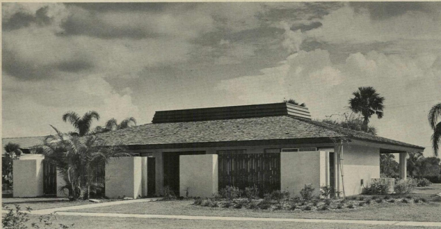
TERRACE FENCING (view 1 in plan) of alternating masonry and wood panels, an optional extra, screens front of house. Roofing is hand-split shakes.
