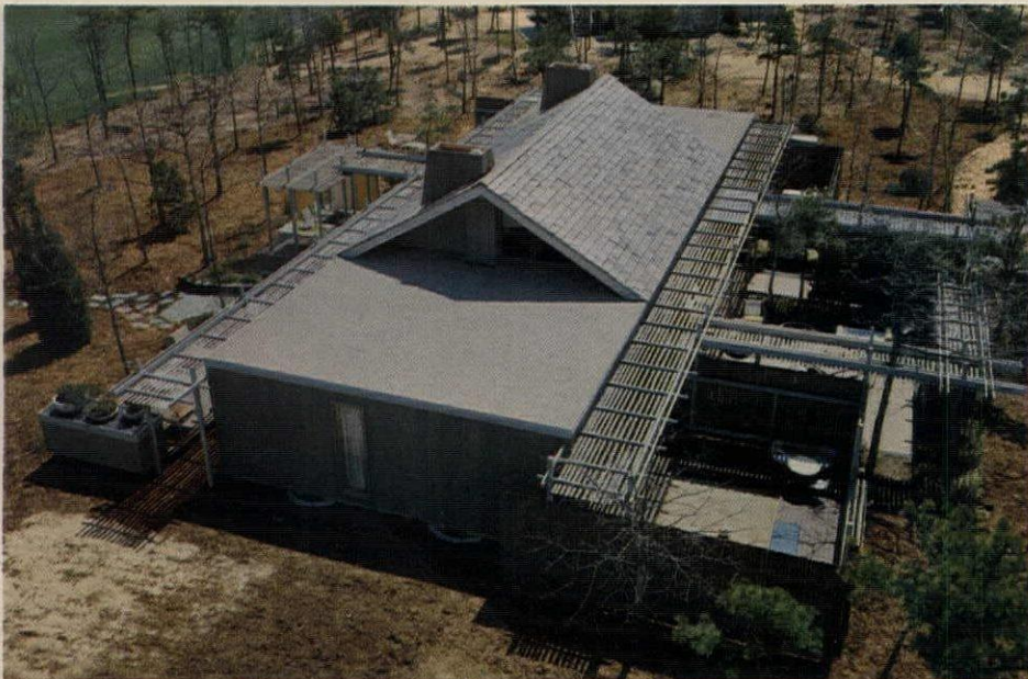
FRONT AND REAR PATIOS (3) are visible in end view. Eave trellises extend 3' as sun shields.
