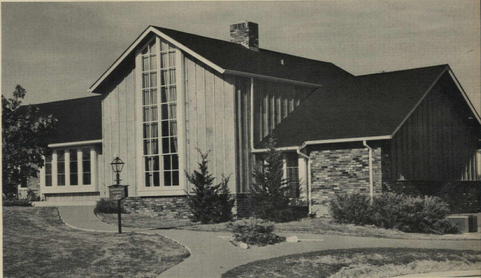
FRONT ELEVATION (3) features two-story living-room window. Wing at right has two bedrooms and a bath; wing at left includes kitchen, dining room.
