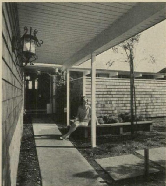
ENTRANCE WALK (2) is sheltered by a post-supported extension of the flat garage roof.
