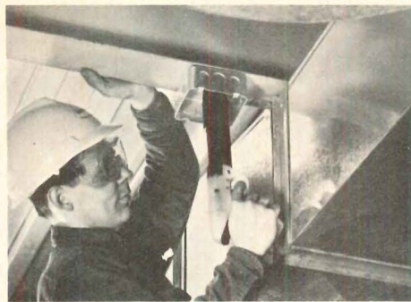
POWER PILL for fastening guns is unique because it has no cartridge case. It comes in lots of 100, in three energy levels color-coded for identification.
