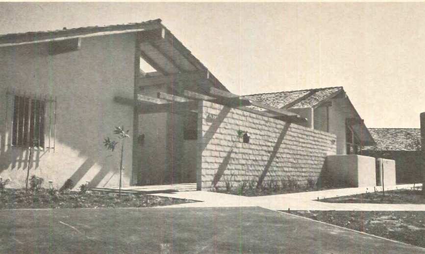
ONE-STORY HOUSES are sided with stucco, fenced with adobe brick. Roofs are shingled on one-story units to keep over-all costs down.
