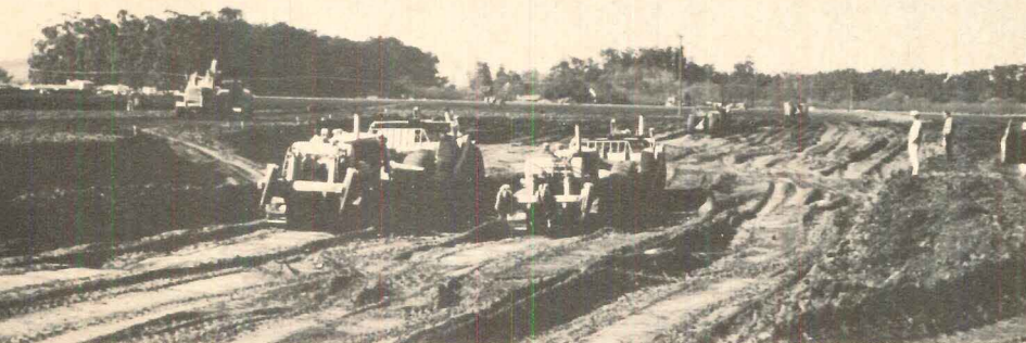
LAKE BED is cut by scrapers (above). About 500,000 cu. yds. of earth were moved. Two 18" openings (left) lead water to municipal drains, also maintain lake's basic 7' depth. Lake was filled (below) from wells that also make up water losses from seepage and evaporation.
