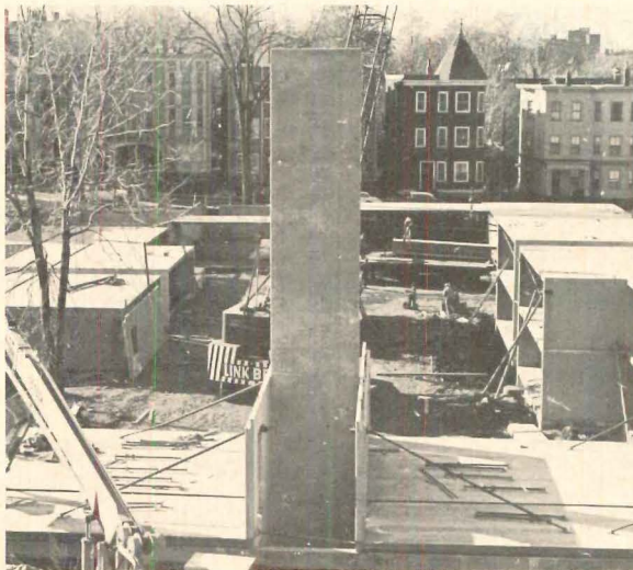
PRESTRESSED SHEAR WALL , held up by two wall panels (left), is the rigid nucleus around which Techcrete panels are erected (above). Shear walls, at right angles to loadbearing panels, extend to full building height and form stairwells. They are prestressed, 4" thick and 6' wide.
