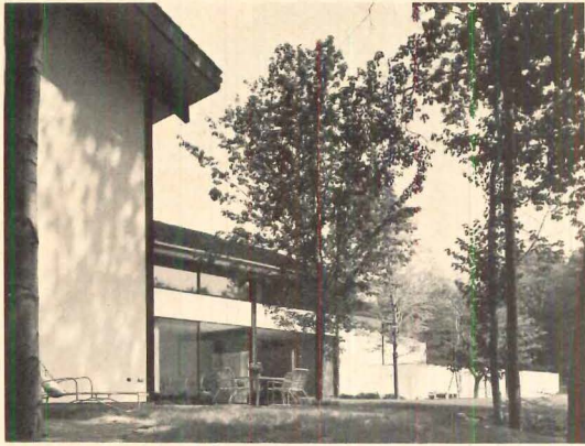
ADULTS' WING , left, juts out from rear of house. Family area is in center, service area at right.
