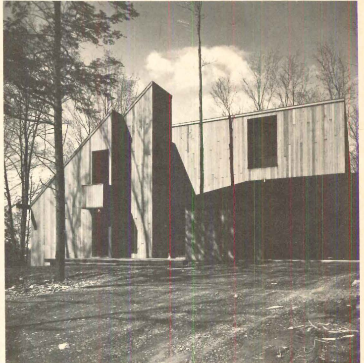
STREET ELEVATION , which faces south, is almost windowless. High section set out from wing at left houses circular stairway.
