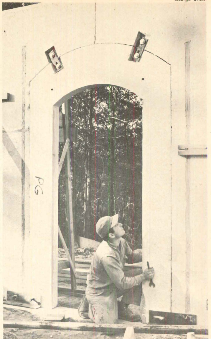
CONNECTIONS consist of plates and angle-irons bolted to cast-in fasteners. Furring strips for attaching interior finishes are also cast in.
