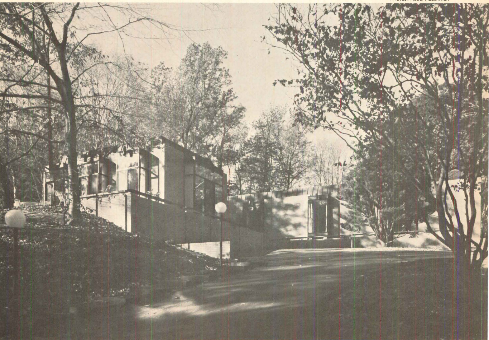
NORMAL TERRACES surround living room, left. Driveway leads to front entrance beyond living room and to left, then continues to below-grade garage.
