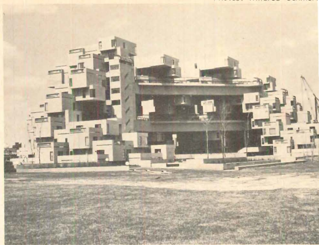
BUILT-IN PEDESTRIAN STREETS also function as structural beam and as conduits for sewers, water and electrical service. City of Montreal pays cost of utility lines from level to level.
