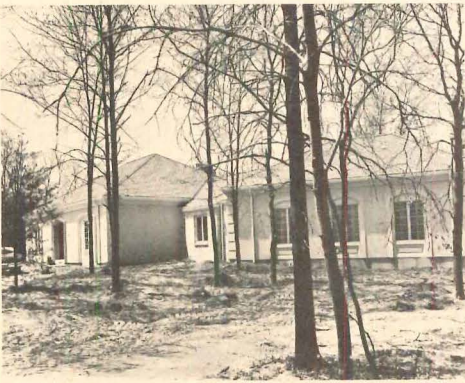
PRECAST HOUSE looks normal from street because roof was built and pitched conventionally.
