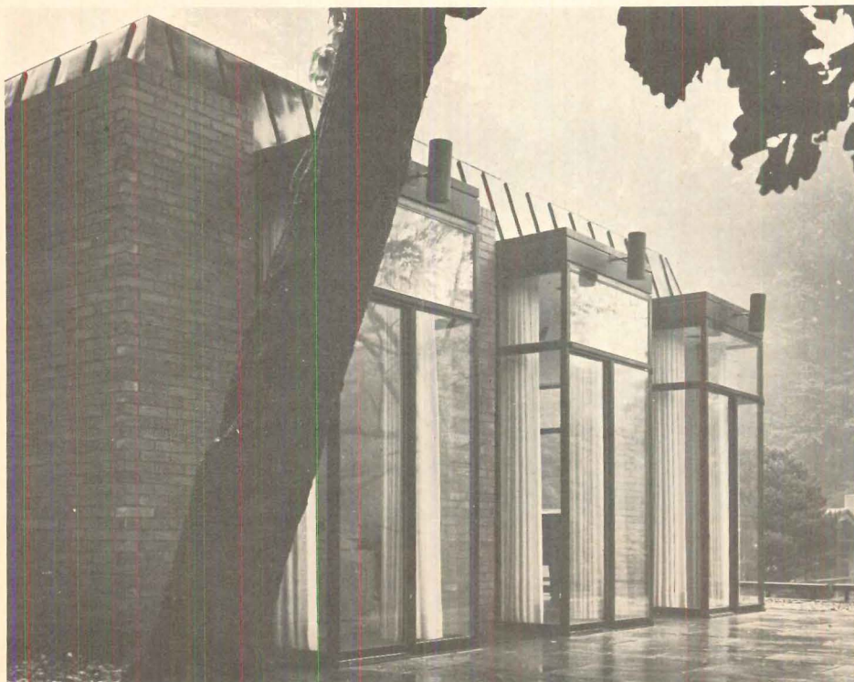
BAY WINDOWS on long side of living room are 5' wide, 10' tall. Frames are black aluminum.
