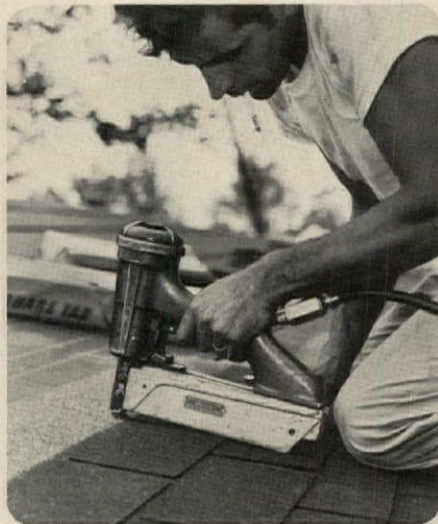
6. Asphalt shingles are laid faster and tighter with wide-crown Duo-Fast Staples.
