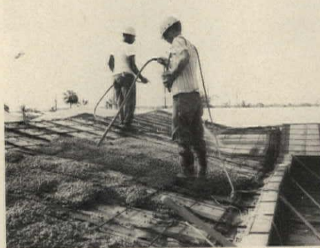
SPUD VIBRATOR consolidates concrete in the narrow 3 5/8" space between truss forms.
