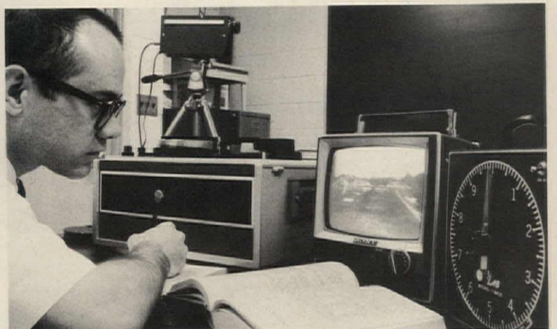
TIME-AND-MOTION STUDY of a critical-path-method operation is logged from a tape viewer. The student will try to find a more efficient work schedule.
