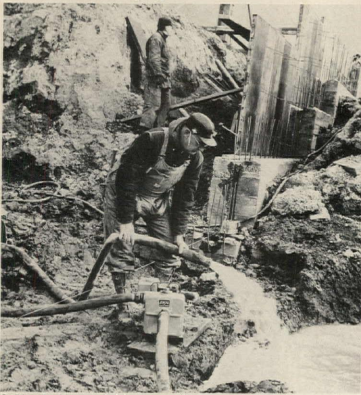
Self-priming portable pump for excavation, ditch and caisson work pumps 13,800 gph at a total head of 50', yet weighs only 106 lbs. Three other models with head capacities of from 20' to 100' are available. Skil, Chicago. Circle 211 on Reader Service card
