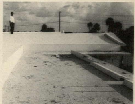
PRECAST FASCIA , used as rain-water barrier, is applied separately to roof perimeter.
