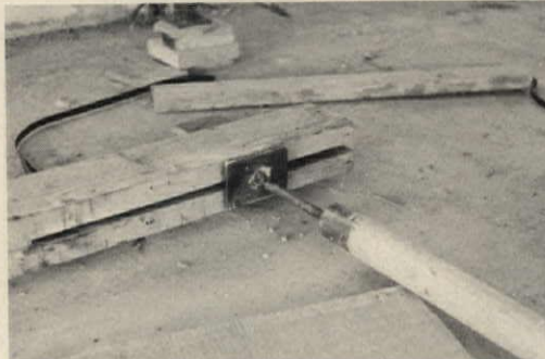
PIPE CAP contains a welded-on pin that fits into a hole in the fitch beam (left), but the beam is supported by a 1/4" steel-plate wedge (right). Beams can be dropped 2" by knocking out wedge.
