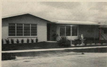
FINISHED HOUSE requires minimum exterior upkeep and is highly storm resistant.
