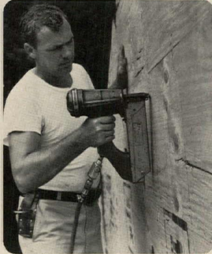
3. Sheathing holds tighter with 2" staples driven by a Duo-Fast Staple Nailer.
