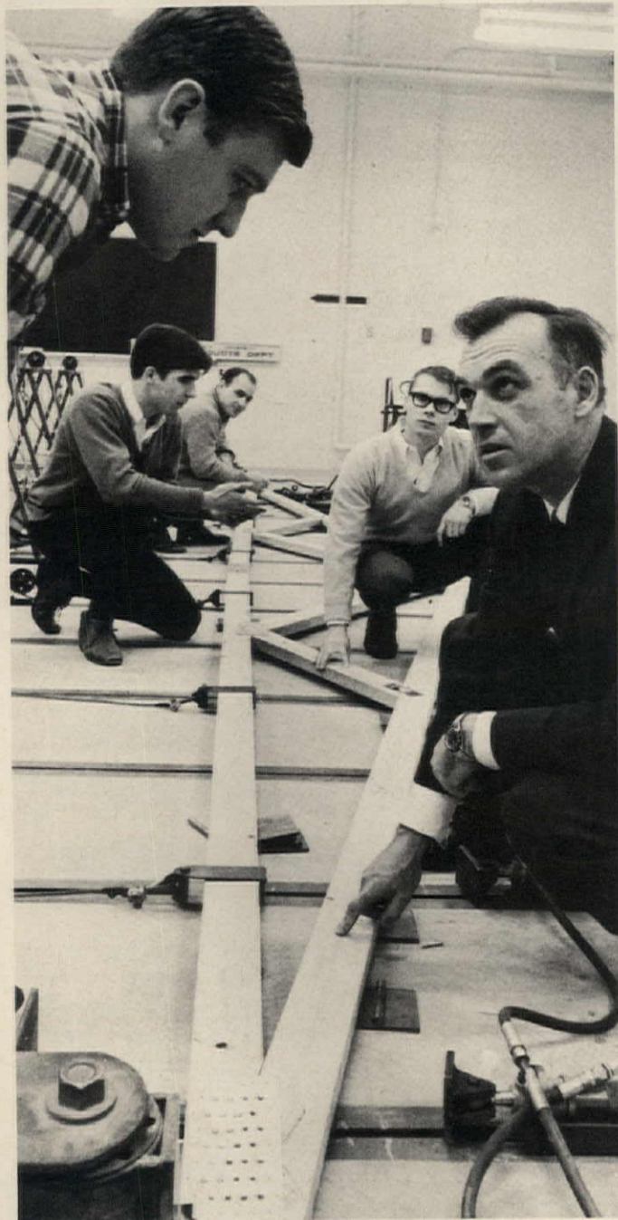
STRUCTURAL EXPERIMENT determines the strength of a low-pitched W-truss nailed together with steel connector plates. Hydraulic stress rig, called "the rack" by students, can create virtually any kind of load condition. Students themselves built the truss.
