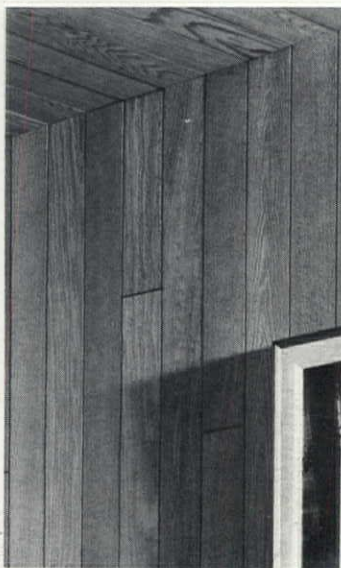
Two-way redwood paneling with T&G rough-sawn face for walls can be reversed to expose a smooth back ( ceiling, above ) with hairline joints. The 3/8"-thick panels come 4" and 6" wide in random lengths. Simpson Timber, Seattle. Circle 221 on Reader Service card
