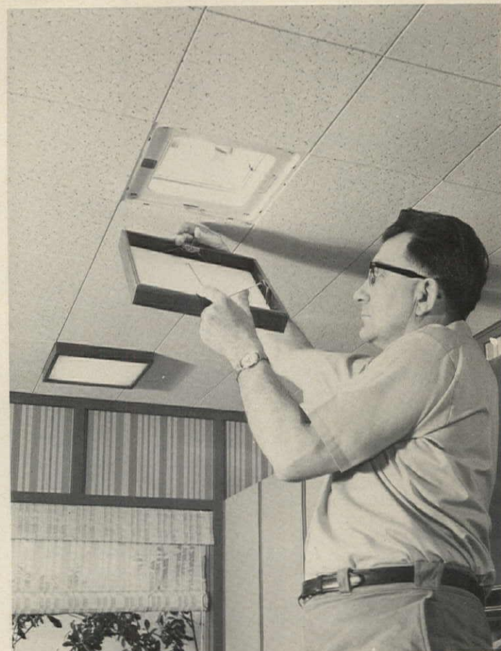
Ceiling fixture —the same size as a standard 12"x12" ceiling tile—is easily inserted in place of a tile ( above ) during ceiling installation, eliminates cutting and fitting. It has a woodgrained lens frame. Armstrong, Lancaster, Pa. Circle 215 on Reader Service card
