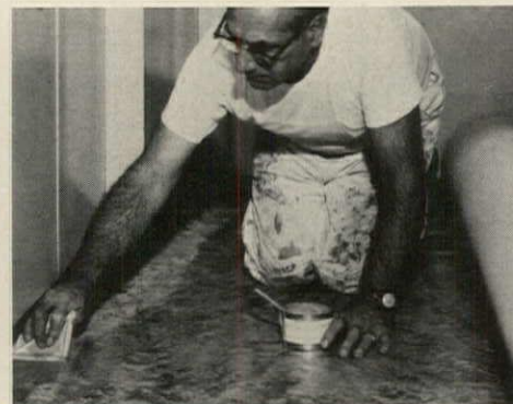
2. CEMENT is spread only on sanded strips, which include seam lines as well as perimeter.
