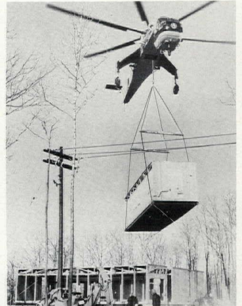
TEN-TON HELICOPTER used for this stackup job may also be used to transport modular boxes designed by Modular Facilities ( letter, below ).
