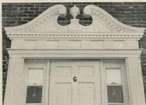
PLASTIC TRIMWORK is already used by prefabbers. Above: a Kingsberry Homes molded lintel.
