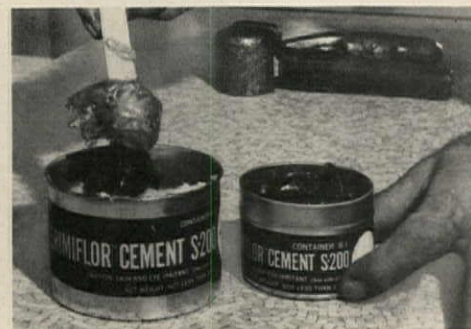
TWO-PART ADHESIVE is blended on the job. The amount shown covers a 4" strip 35' long.
