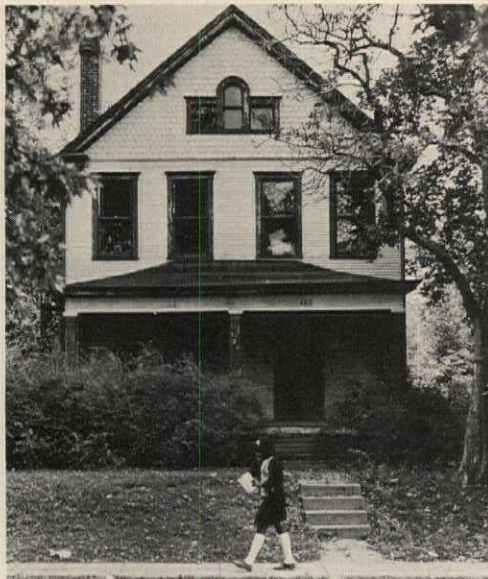
SINGLE-FAMILY HOUSE is one of ten being renovated in Columbus, Ohio, by National Gyp-
