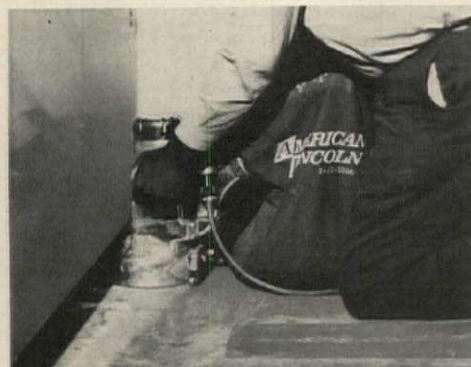
1. SANDING MACHINE roughens old linoleum in a narrow strip around perimeter of kitchen.
