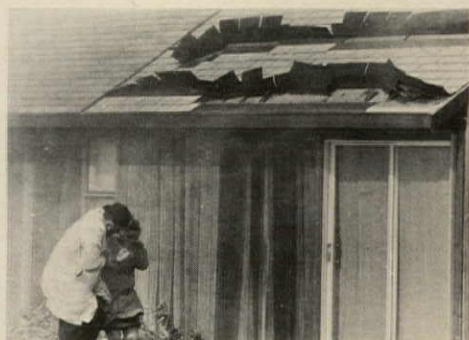
SEVERAL COURSES of conventional shingles are raised by winds. Wind-seal shingles remain flat.
