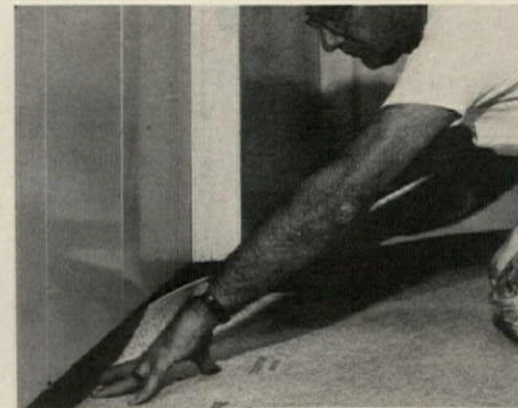
3. NEW VINYL is installed in precut sheet and then hand-rolled to fill seams with cement.
