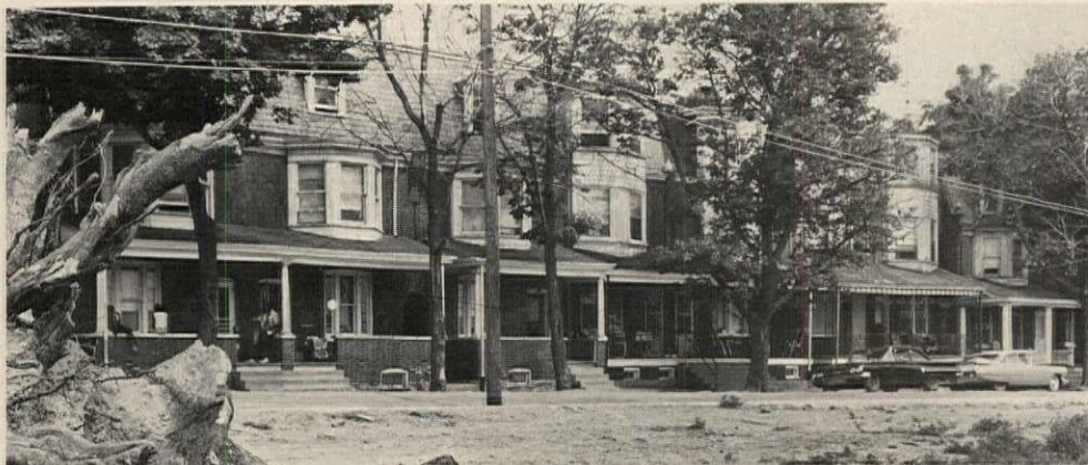
ROWHOUSES in Lancaster, Pa., provide Armstrong Cork Co. with a proving ground for re-
