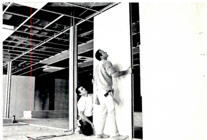
Partition system has prefabbed panels of gypsumboard glued to paperboard ribs. Panels are shipped flat, opened to 1 \frac{5}{8} " rib thickness at site, positioned on floor runner, tipped into position and attached. Pabco, San Francisco. Circle 334 on Reader Service card
