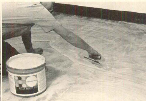
HOW IT'S DONE (left to right): Sand old flooring to remove finish; trowel on adhesive; apply new tile within 18 hours after adhesive turns tacky.
