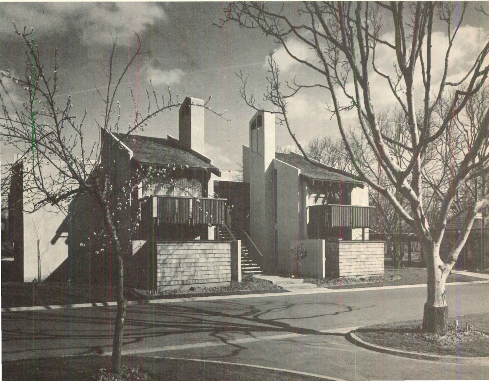
OUTSIDE STAIRWAY is a private entrance to a second-floor apartment. Pre-cast concrete stair treads are surfaced with pebbles.
