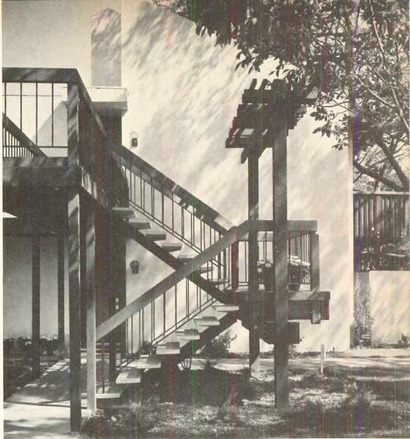
OUTSIDE STAIRWAY is a private entrance to a second-floor apartment. Pre-cast concrete stair treads are surfaced with pebbles.
