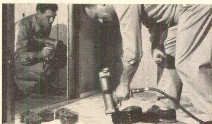
Drive them with a Bostitch Model N2 air-driven coil-fed nailer. It's almost
