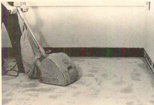
HOW IT'S DONE (left to right): Sand old flooring to remove finish; trowel on adhesive; apply new tile within 18 hours after adhesive turns tacky.
