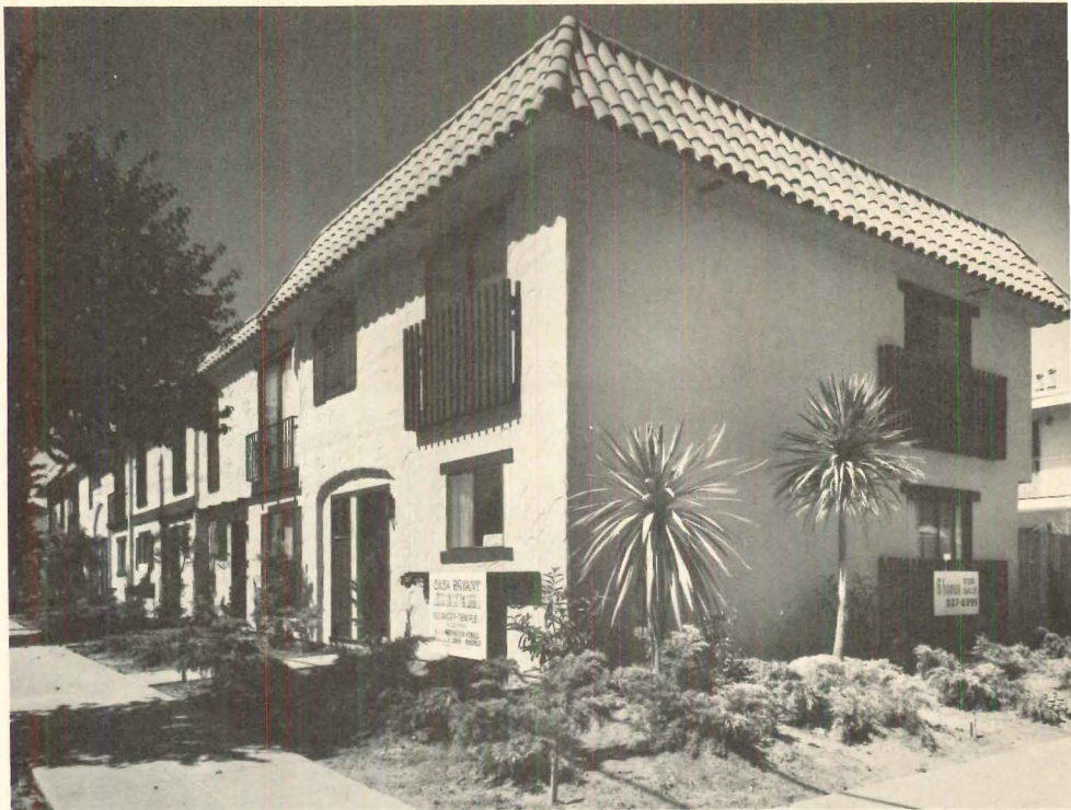
SIX-UNIT TOWNHOUSE PROJECT contains two-bedroom condominiums with top price of $33,200. Basement ( drawings, below ) provides 300 sq. ft. of extra utility and storage space for each unit.
