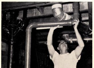
PVC pipe is self-extinguishing and thus prevents flame from spreading along pipes between walls. It also resists abuse and does not allow scale to build up inside pipe or fittings.
