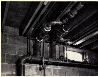
Now that PVC is fast growing in acceptance for drain/waste/vent systems in new construction as well as rehabilitation, the builder who hasn't looked into its advantages stands a chance of falling behind.
