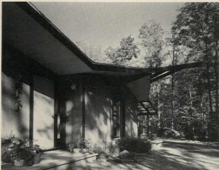
LARGE OVERHANG shelters entrance. Use of four modules allows the unusual folded-plate roof. Trellis, in background, is above side deck.
