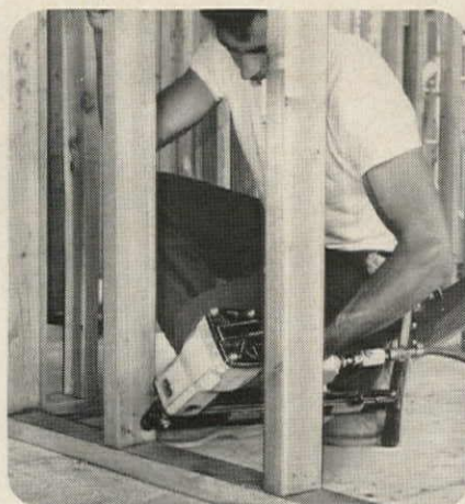
CN-137 makes fast work of toe-nailing
