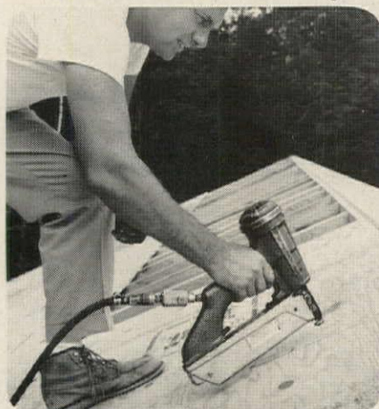
Staple Nailer anchors down plywood roof deck
