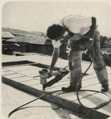
Fast on-site component construction with CN-137
