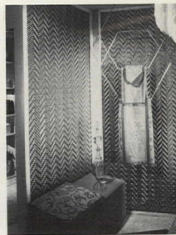
are applied to walls with mastic, then framed with matching moldings. Styles include mirror finish ( left ) and herringbone ( right ). Schacht, Bronx, N.Y.
