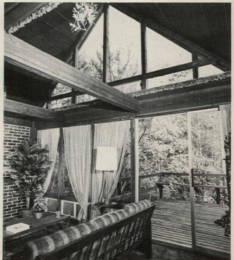
Gable window wall is butt-hinged at upper plate (double 2 x 4s) and folds down in transit to site. Deck off living room was added at owner's expense.
