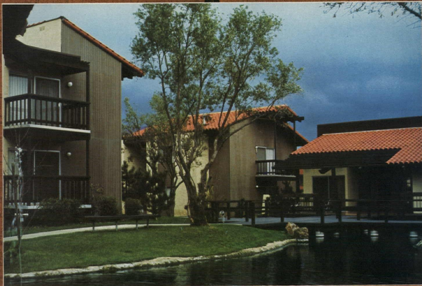
Ruf-Sawn Shadow Groove on Casa Grande Apartments Architect: Maxwell Starkman Developer: Hy Weisel
