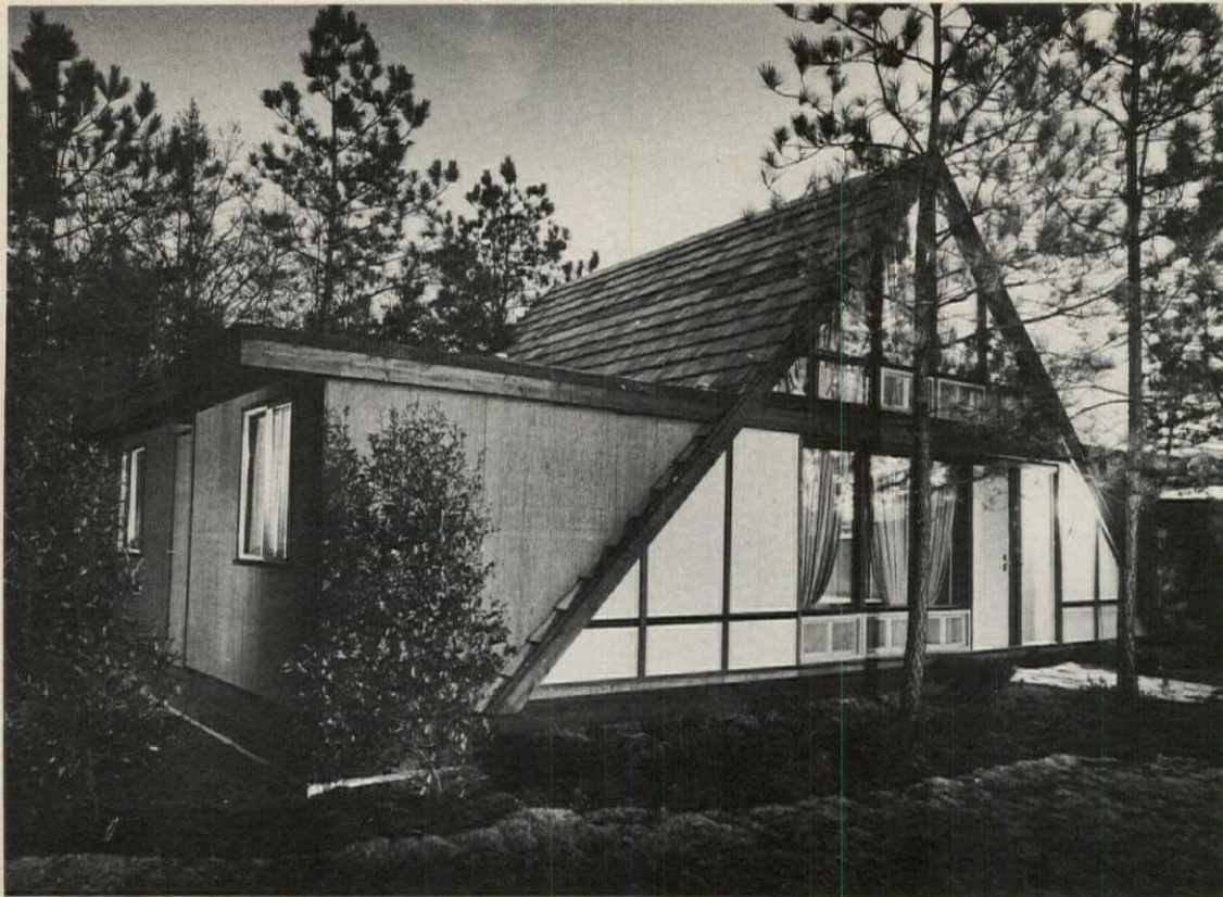
Double-wide modular plan includes two bedrooms and two baths on the first floor and third bedroom above. Total living area is 1,100 sq. ft. House rests on steel I-beams on concrete piers and has electric heat.
