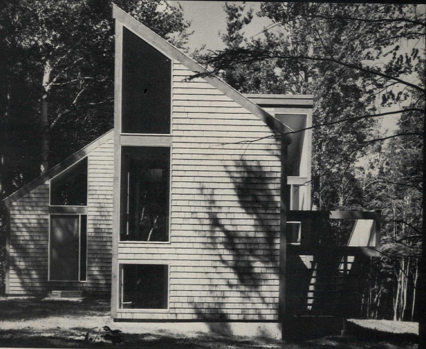
Vacation home at Francestown, New Hampshire. Certigrade Shingles No. 1 Grade 16" Fivex. Architect: Brett Donham.
