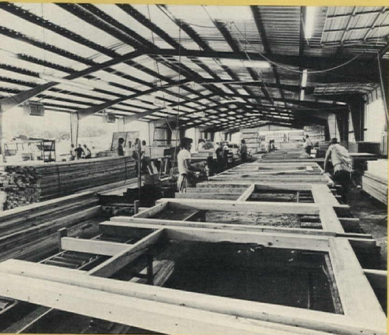
Component factory turns out walls and partitions as well as millwork items like cabinets, railings, etc. Company has recently put greater stress on such pre-site fabrication.
