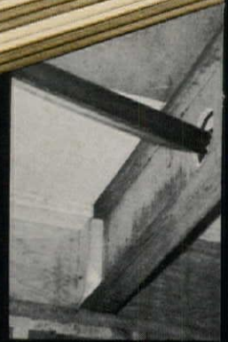
Plywood web cuts easily
