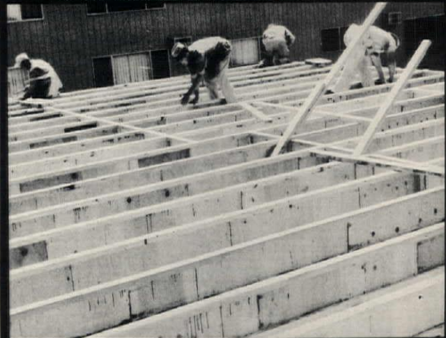
I Series joists go in place 2 to 4 times faster than 2 x 10's.
