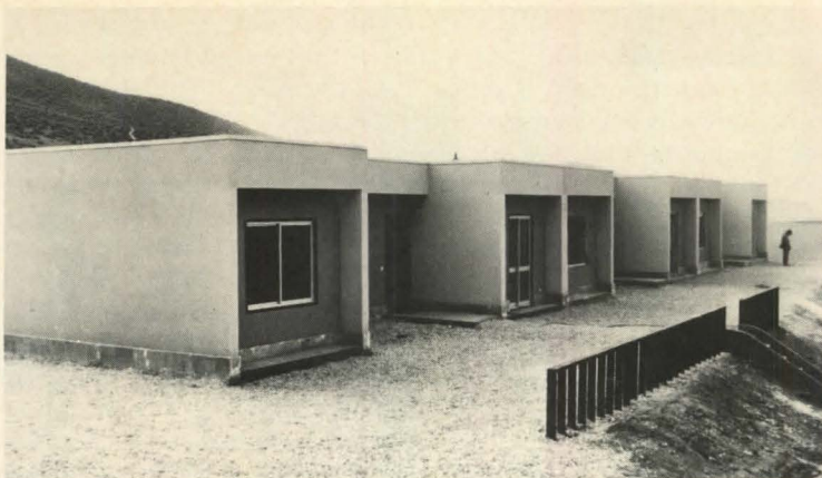
Prefab houses from GE , all in a row in Sar Cheshmeh, Iran. Besides building 500 units here (see story), GE's licensee, Gostareh Maskan Co., has a $50,000,000 contract to start a new town for 200,000 people.
