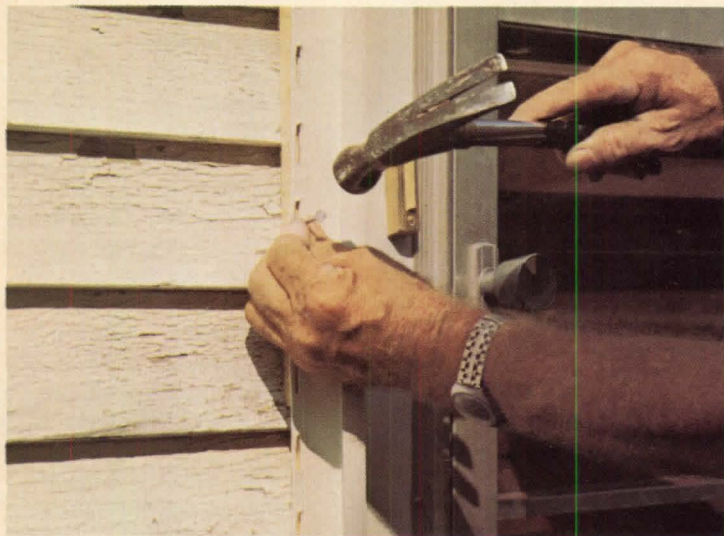
4. Trim sides and tops of doors and windows with J channels or window/door caps. Installation of siding panels now begins.
