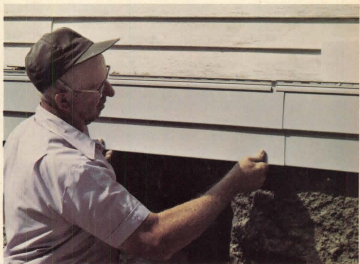
5. Snap bottom panels into the starter strip and nail. Backer board can be used for extra insulation.
