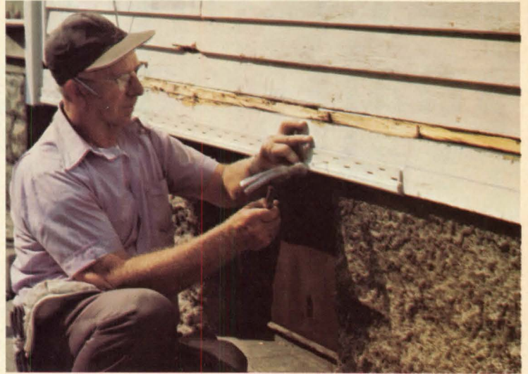
3. Position starter strip with top edge on the chalk line. Do not nail too tight; stop when hammer head touches edges of nailing strips.
