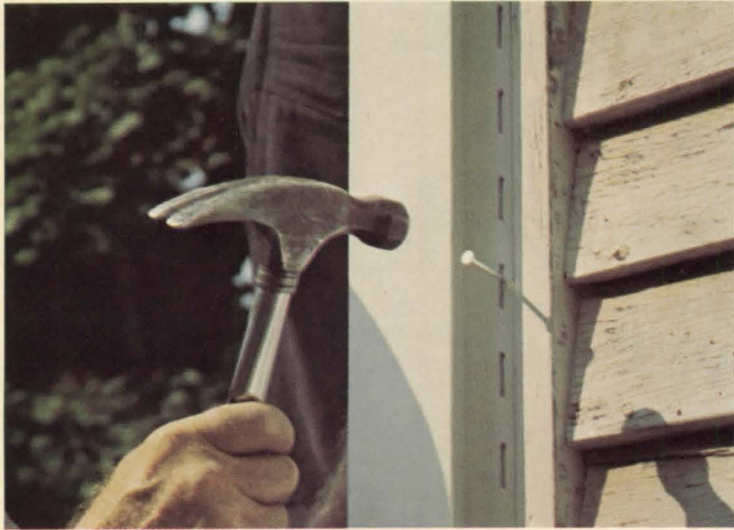
2. Install all inside and outside corner posts. Leave \frac{1}{4} " at top. Finish nailing every 10" to 12" in the center of the slots.
