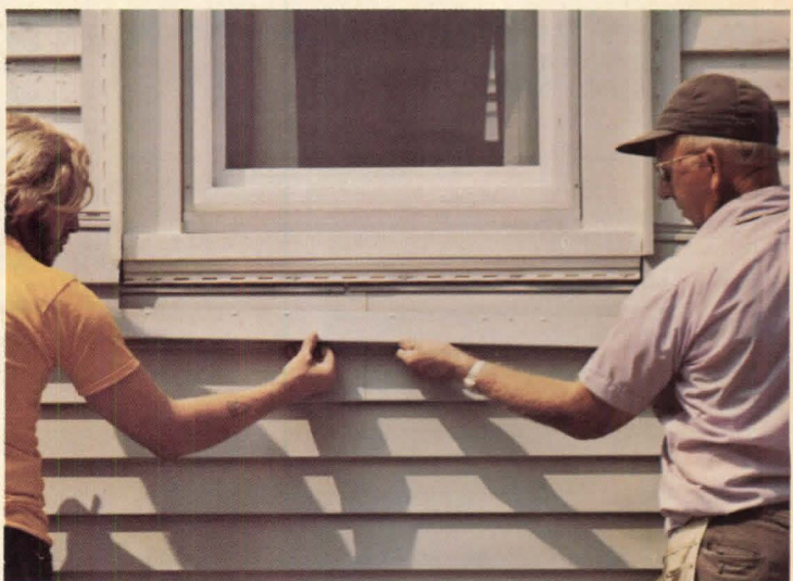
9. Slide the panel into the undersill trim. Installation of the top course follows a similar procedure.
