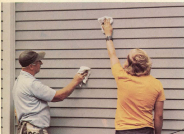
10. When installation is completed, wipe clean with mild detergent solution and you have a vinyl clad house that will stay beautiful for years.
