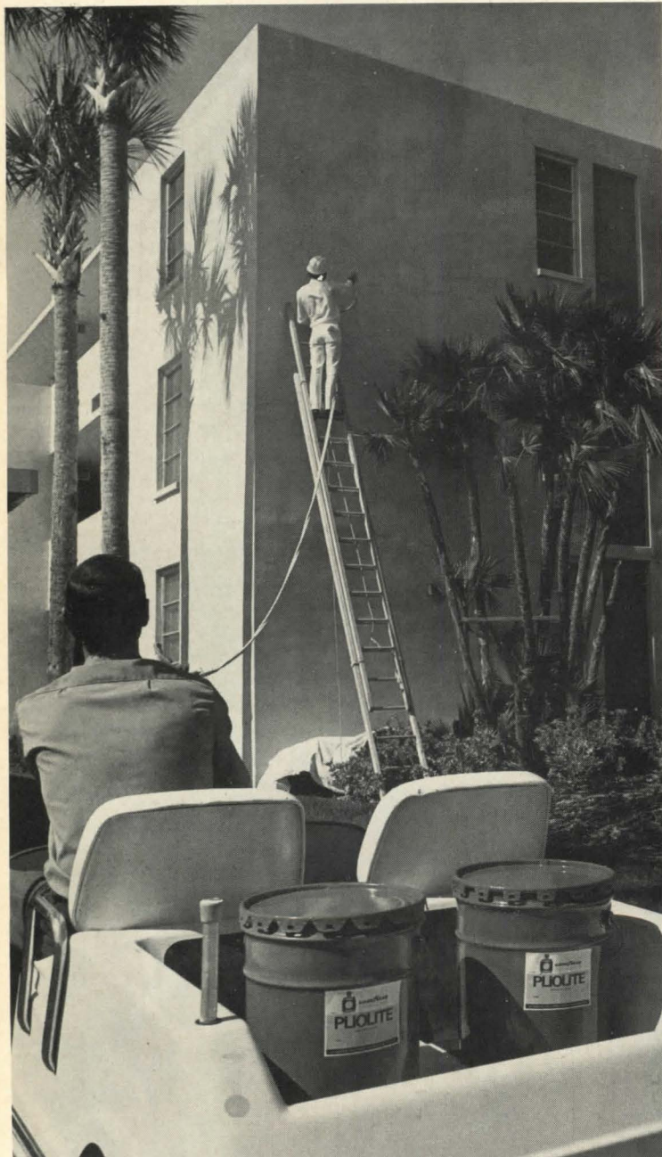
Textured protective coating with Pliolite resin base helps preserve the surface of a concrete building. Imperfections are hidden and water, salt, mildew and air-pollution damage are prevented. Spray-applied coating is offered in textures ranging from gritty to pebbly and in white and most standard colors. Goodyear, Akron. CIRCLE 253 ON READER SERVICE CARD
