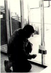
Plastic junction box, non-shock type, is feature of F&J houses, which provide abundance of electric outlets that are placed conveniently.
