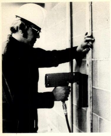
Pneumatic nailer, "Model M111," drives hardened nails through wood or light steel into concrete. Nailer, which operates on air pressures from 60 to 90 psi, is equipped with narrow nose for easy access into corners. Nails in four lengths have .097" shank diameter. Bostitch, E. Greenwich, R.I. CIRCLE 260 ON READER SERVICE CARD
