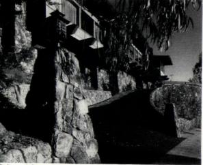
Cultured Stone Veneer ® (above) simulates the color and texure of natural stone. Made from Portland cement, the inte-ior/exterior veneer can be applied with mortar over uneven ub-surfaces and corners. Stucco Stone, Napa, CA. Circle 216 in reader service card
