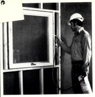
Polymeric foam sealant, Polycel OneTM (above), forms a permanent closed-cell barrier against infiltration of air and moisture. Sealant is easy to apply. Coplanar, Oakland, CA. Circle 224 on reader service card
