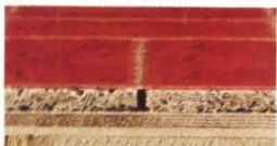
Tredway adjusts to seasonal subfloor changes.
