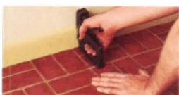
Tredway installs with staples.
