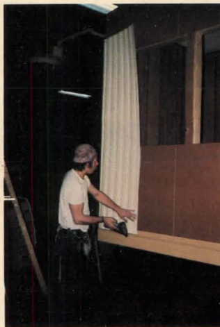
Siding, insulation and Fome-Cor sheathing board.
