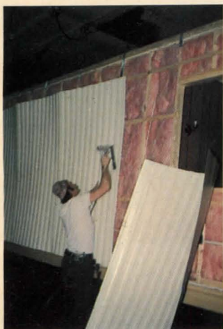
Siding, insulation and caulked seams.
