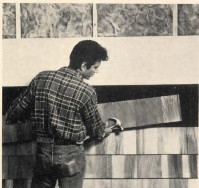
Prefabricated section of red cedar shingles (above) may be applied over foamed insulation. Shakertown, Seattle, WA. NAHB booth 1372. Circle 359 on reader service card
