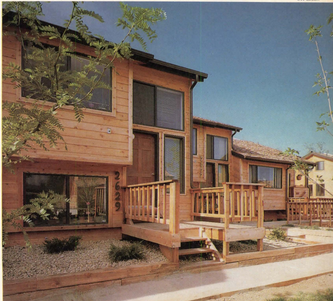
Cedar siding and cedar-shake roofs give townhouses a rustic look.
