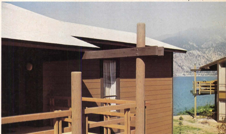
Washington Condominiums, Howard S. Wright Construction Co.
