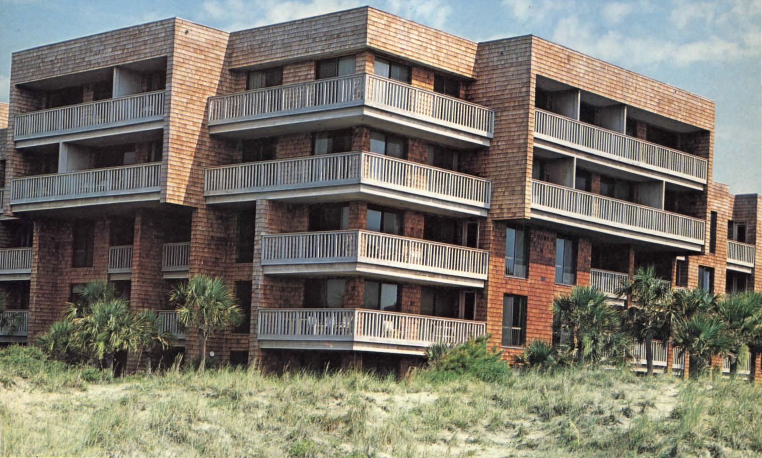
Shipwatch Villas, Kiawah, South Carolina Owner: Kiawah Island Company Architects: Jova/Daniels/Busby
