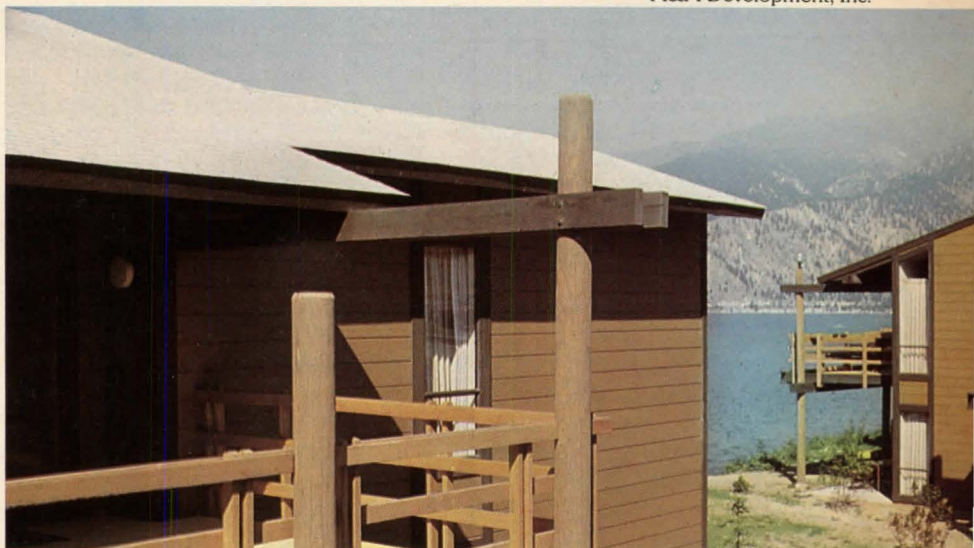
Washington Condominiums, Howard S. Wright Construction Co.
