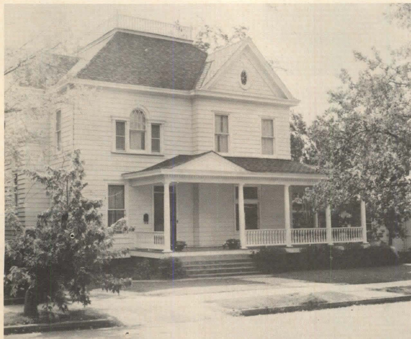
Weathergard™ columns and Colonial spindles (above) give this turn-of-the-century home a Victorian look. Wood columns are available in stock sizes from eight to 20 ft. E.A. Nord, Everett, WA. Circle 235 on reader service card
