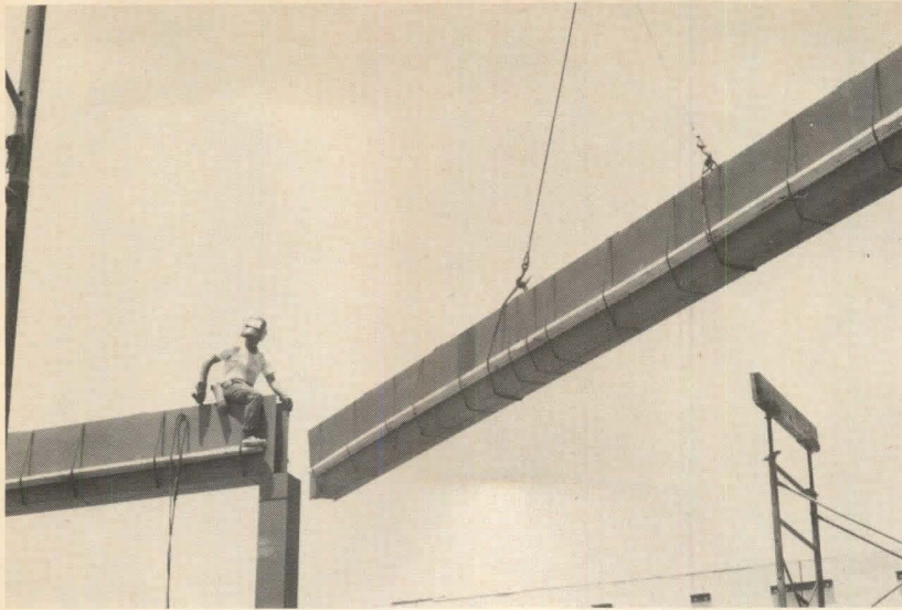
Column-and-beam concrete forming system (above) features prefabricated metal forms which can be left in place. Only erection, bracing and concreting are required on the job site. Dayton Sure-Form, Miamisburg, OH. Circle 233 on reader service card
