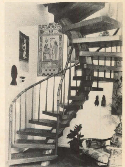
Spiral staircase (above), with two handrails, is precut and shipped in cartons. The staircase is assembled and tensioned (by cables) on the job. Stair treads and risers are made of laminated pine. Diameters range from 6'0" to 7'6". Spiral Manufacturing, Baton Rouge, LA. Circle 238 on reader service card
