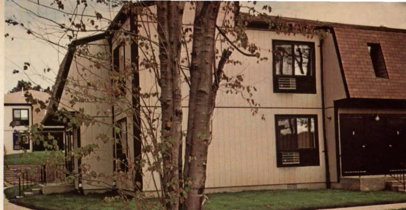
New York Apartments, Mar-Jef Construction Co.
