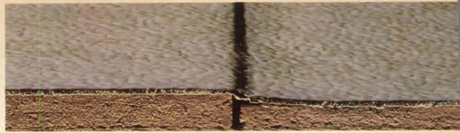
Conventional flooring can ridge or split.
