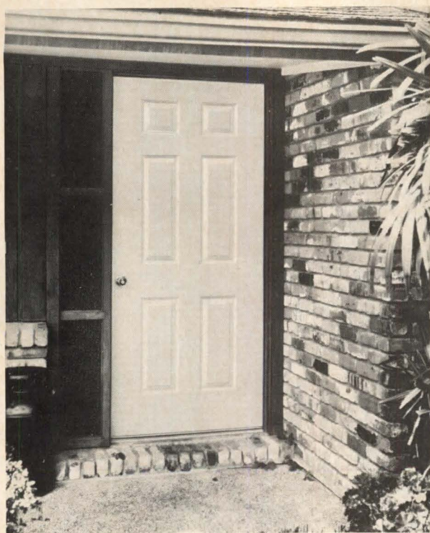
Pre-hung entry door (above) is constructed of 24-gauge steel sheet. Door is insulated with seven pounds of polyurethane foam and has a vinyl sheet thermal barrier. National Industries, Ocala, FL. Circle 211 on reader service card
