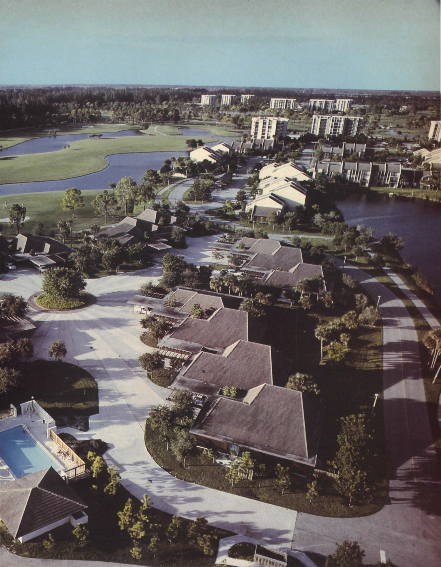
Boca West —Arvida Corp.'s 1,436-acre community in Boca Raton—is the site of Woodcrest, one of south Florida's newest projects (see page 69).
