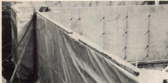
Concrete foundation wrapped with Tu-Tuf vapor barrier sheeting.
